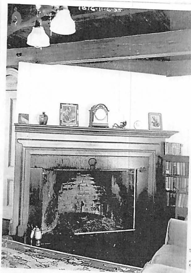
The Jacobus Van Derveer house, interior. Detail of mantel, west wall of living room, first floor, November 6, 1935.
