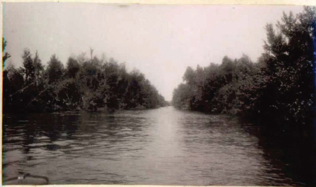
4. This canal, built in part some years ago by logging interests and more recently extended on through the swamp to the Tangipahoa River, provides unnatural drainage for a major portion of the area during periods of high water.
