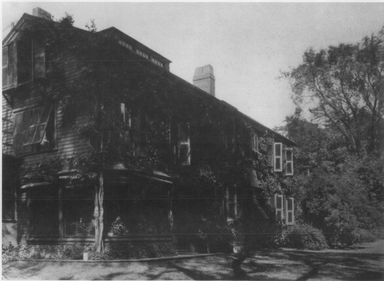
Figure 2. View of the west elevation at Fairsted which shows a steel strapping trellis system built as early as 1884. Photo courtesy of Olmsted National Historic Site.
