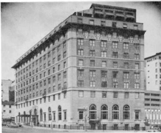
This Washington, D.C. hotel had windows with a multiple pane configuration before rehabilitation.
