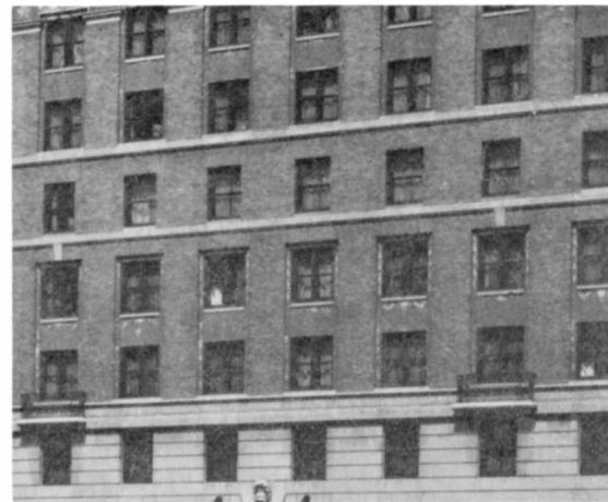
While the pane configuration was not retained in the rehabilitation, the character of the facade as a whole was not significantly changed, making these replacement windows an appropriate solution. Decisions about window replacement must be made on a case-by-case basis.
