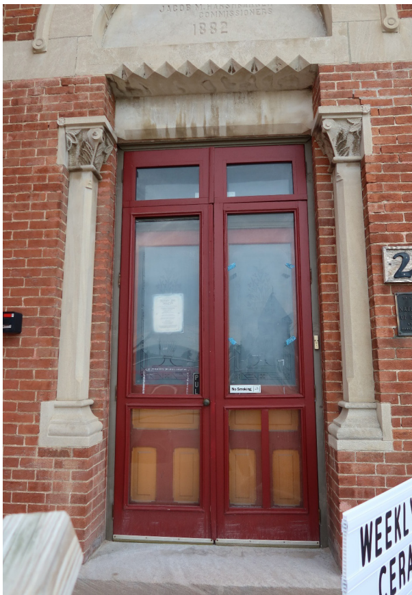
Figure 2.36: Front doors based on original doors with wood storm doors.
