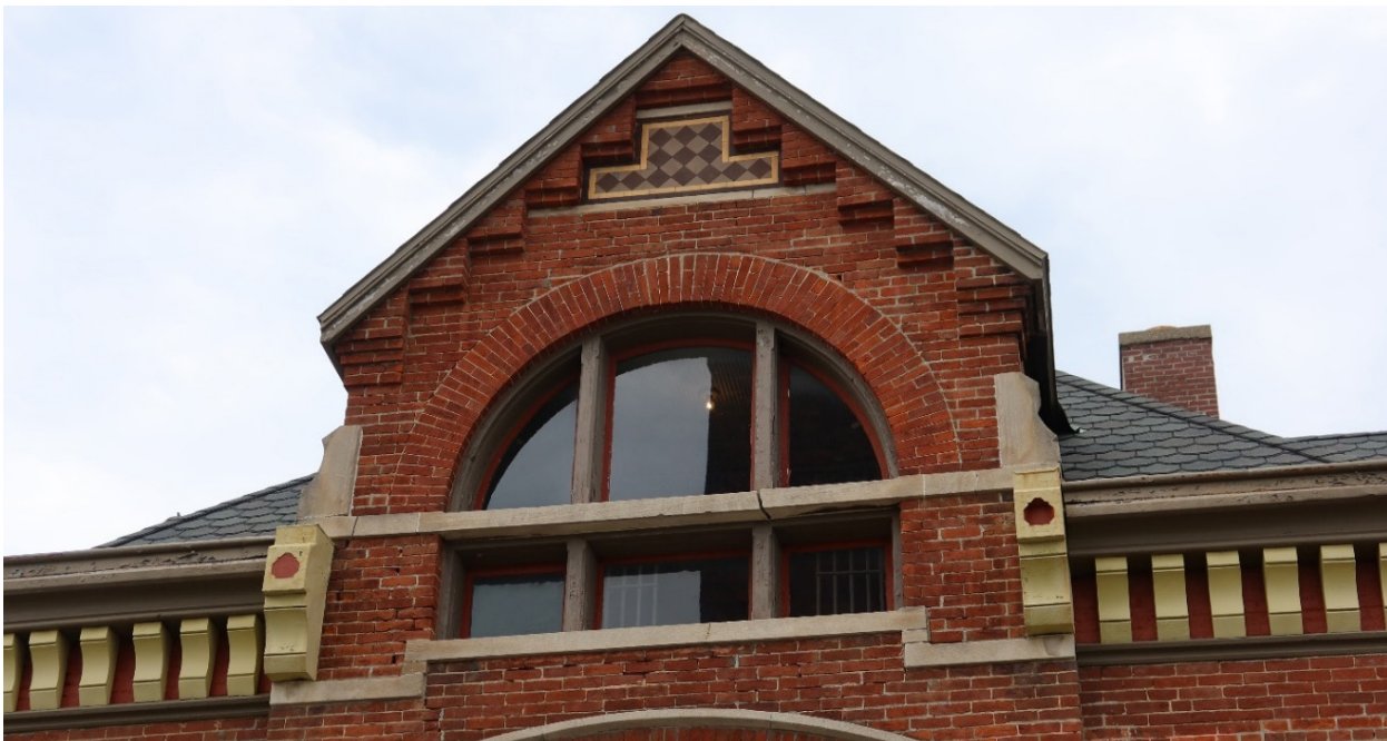
Figure 2.30: Historic wood windows at the residence and jail attic are in fair to good condition overall.
