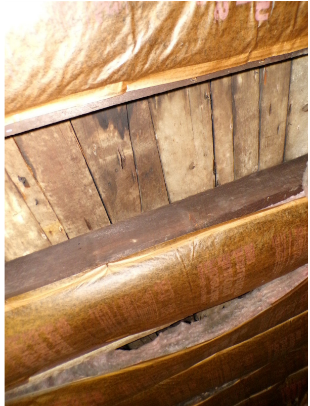
Figure 2.16: Board sheathing was used beneath the roofing.
