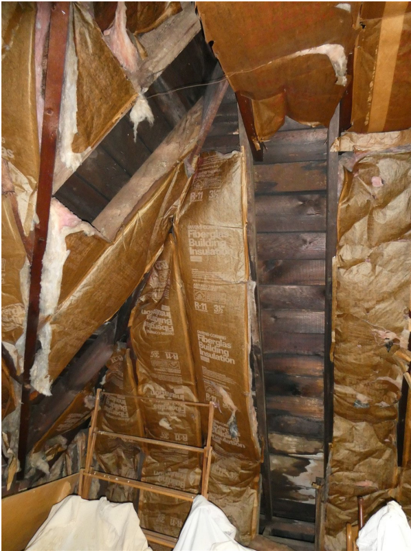
Figure 2.15: Typical view of the roof framing as seen from the attic level.
