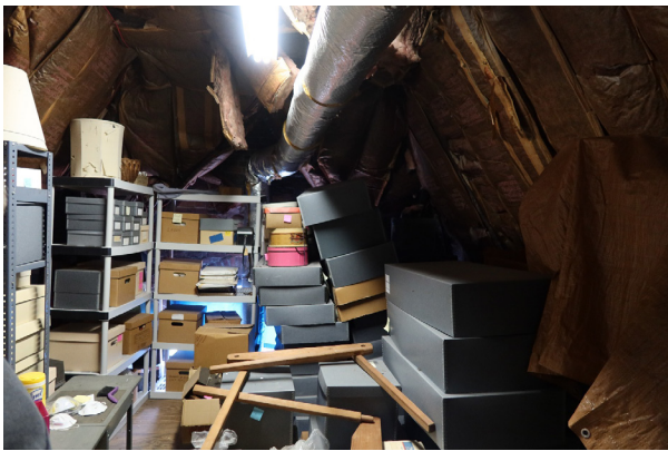
Figure A.2: A prior volunteer curator moved many artifacts to the unconditioned attic in preparation for collections storage improvements that never occurred. This is an unsuitable environment for artifact storage. Attic temperature was 92 degrees Fahrenheit at 10:00 a.m. during site visit.
