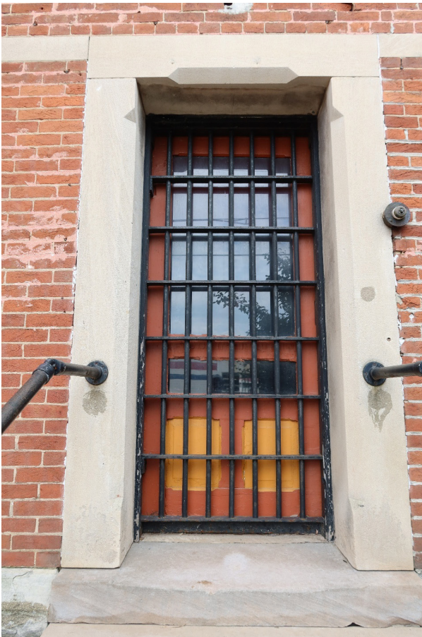
Figure 2.39: Guard room door with exterior bars.
