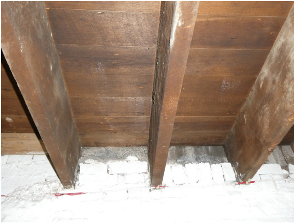
Figure 2.12: The wood framing was visible in several locations in the basement. The wood joists are typically pocketed by the masonry walls.
