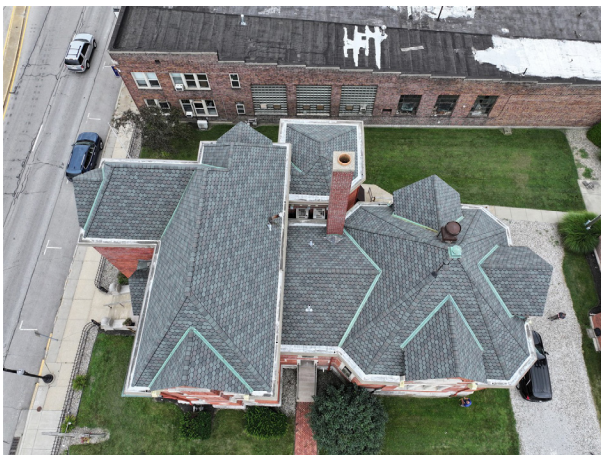
Figure 2.7: An aerial view of the Museum showing the various roof levels, facing south.
