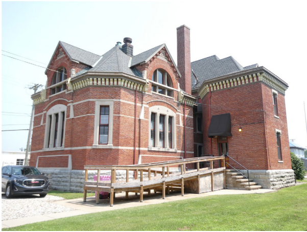
Figure 2.5: The rear of the facility, facing northeast.
