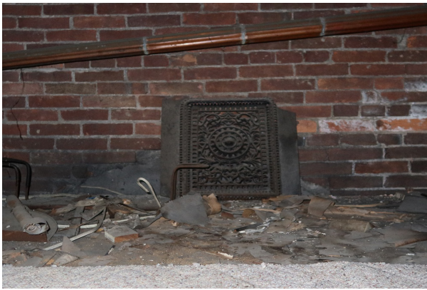
Figure A.1: Cast iron summer cover (left) stored in the residence vestibule's attic probably came from the original parlor fireplace. It matches the cover still in place in the southeast bedroom (right). The sitting room and north bedroom have summer covers of a corresponding design but a different shape.
