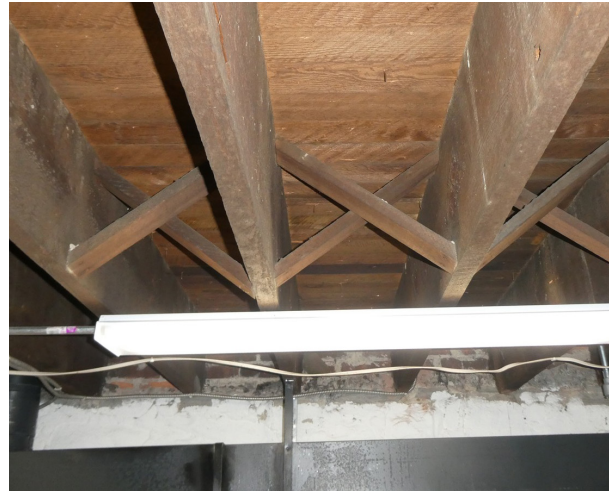
Figure 2.13: Cross bracing was observed within the first-floor framing.
