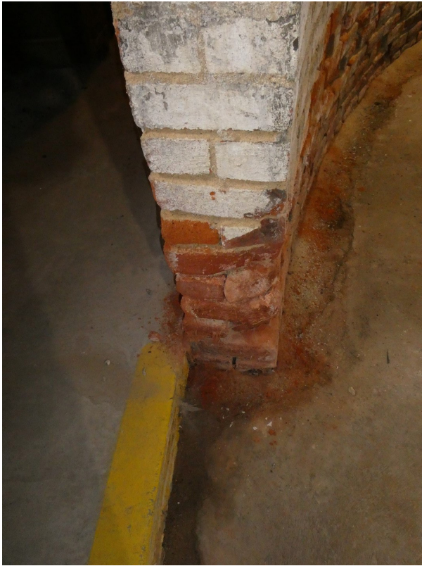
Figure 2.10: The wall is only two wythes in thickness.
