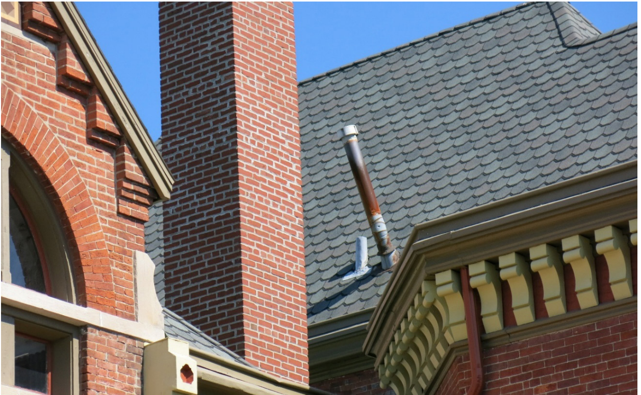
Figure 2.45: West face of house roof showing metal chimney.
