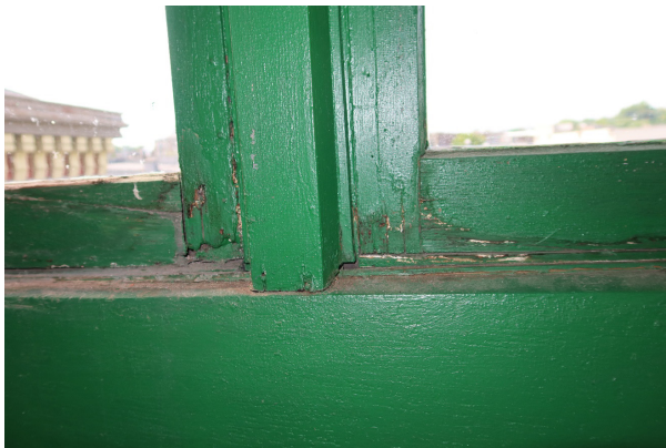
Figure 2.32: Typical jail attic window in fair condition.
