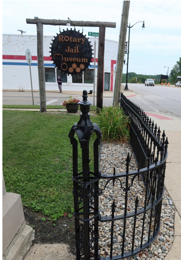
Figure 2.24: The iron fence was recently cleaned and painted and is in good condition overall. The cap of the north fencepost (far end of fence) recently broke loose and is stored inside the building.
