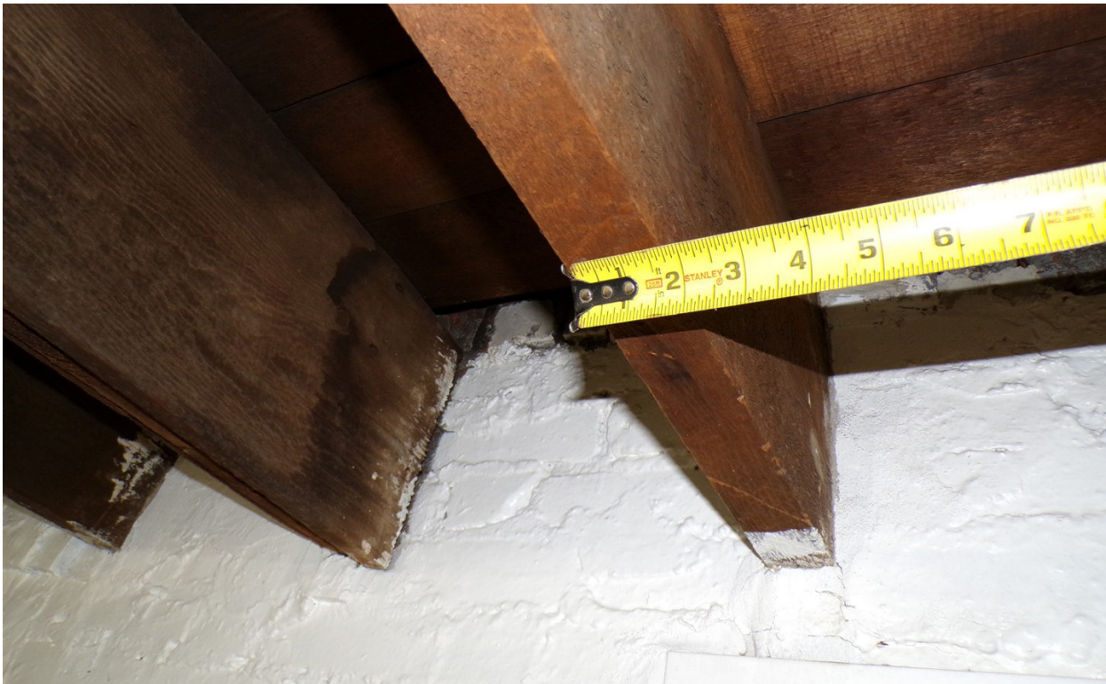
Figure 2.14: The joists were measured to be nominal 2x10 lumber in this location.
