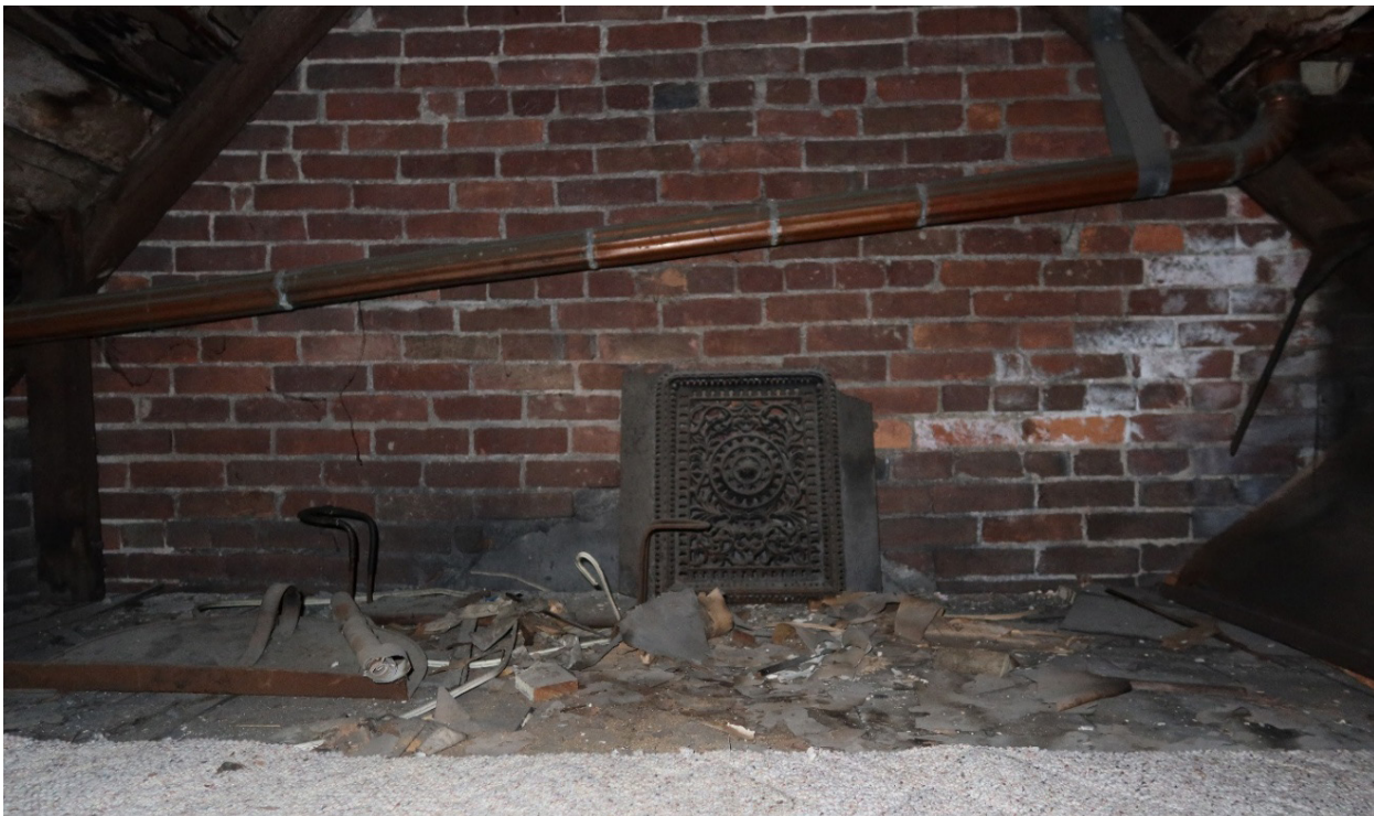
Figure 2.47: Residence vestibule attic, facing east. The downspout draining the south face of the residence vestibule roof passes through the vestibule attic. This appears to be the original detail and does not show any signs of leaks. This attic should be inspected quarterly for signs of leaks.
