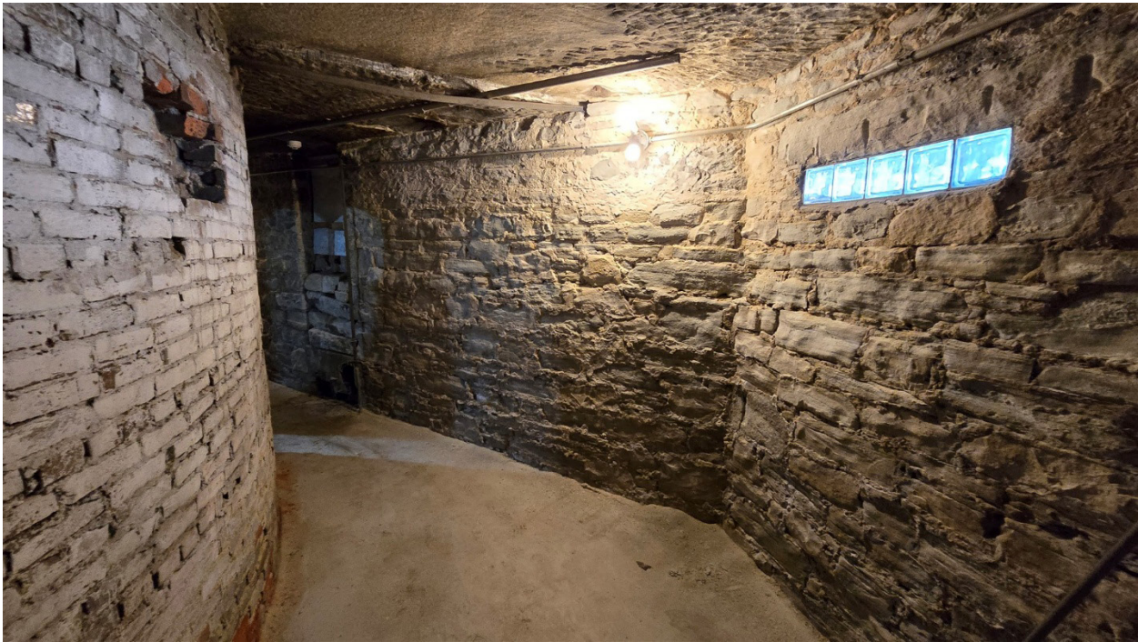
Figure 2.11: The rough limestone foundation of the jail.
