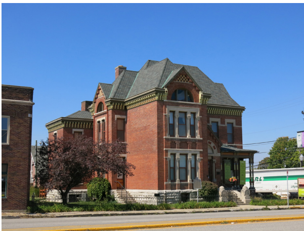
Figure 2.6: The Montgomery County Jail / Rotary Jail Museum in Crawfordsville, Indiana, facing northwest. Source: Personal Collection, Benjamin L. Ross.
