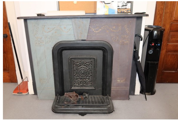
Figure A.1: Cast iron summer cover (left) stored in the residence vestibule's attic probably came from the original parlor fireplace. It matches the cover still in place in the southeast bedroom (right). The sitting room and north bedroom have summer covers of a corresponding design but a different shape.
