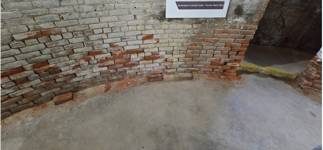
Figure 2.8: The brick masonry wall beneath the rotary jail mechanism.
