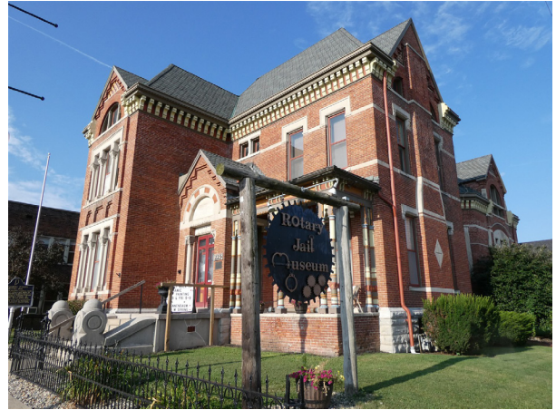
Figure 2.2: The Montgomery County Jail / Rotary Jail Museum in Crawfordsville, Indiana, facing southwest.
