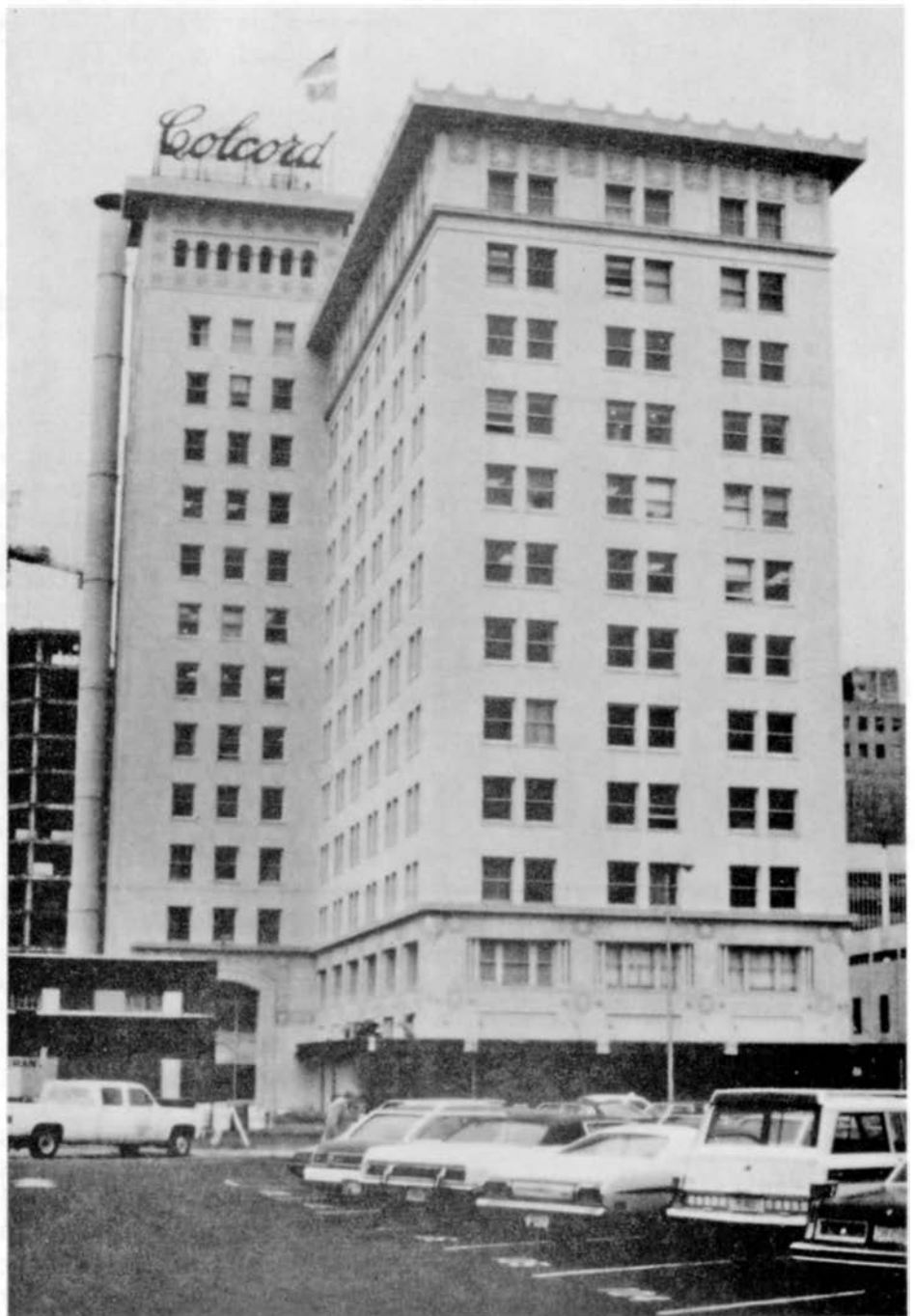
Figure 1. The Colcord Building, Oklahoma City, Oklahoma. This 12-story poured-in-place concrete building with terra-cotta ornamentation was built in 1910 and is individually listed on the National Register of Historic Places. (Photo: H. Ward Jandl)
