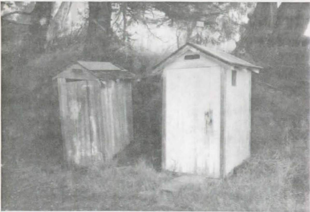
Figure 24 - Structures 14 and 12, outhouses, west and south sides.
