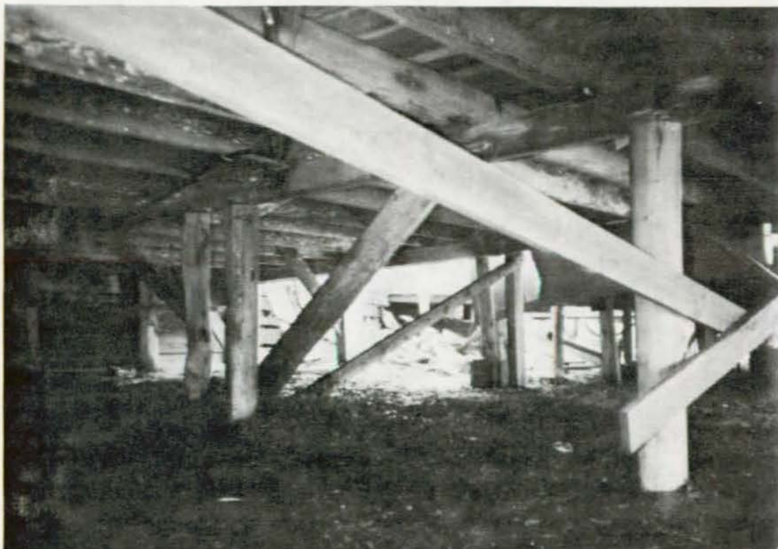
Figure 29 - Structure 17, Spiegel cabin, pilings and subfloor. Typical of all structures at Hamlet.
