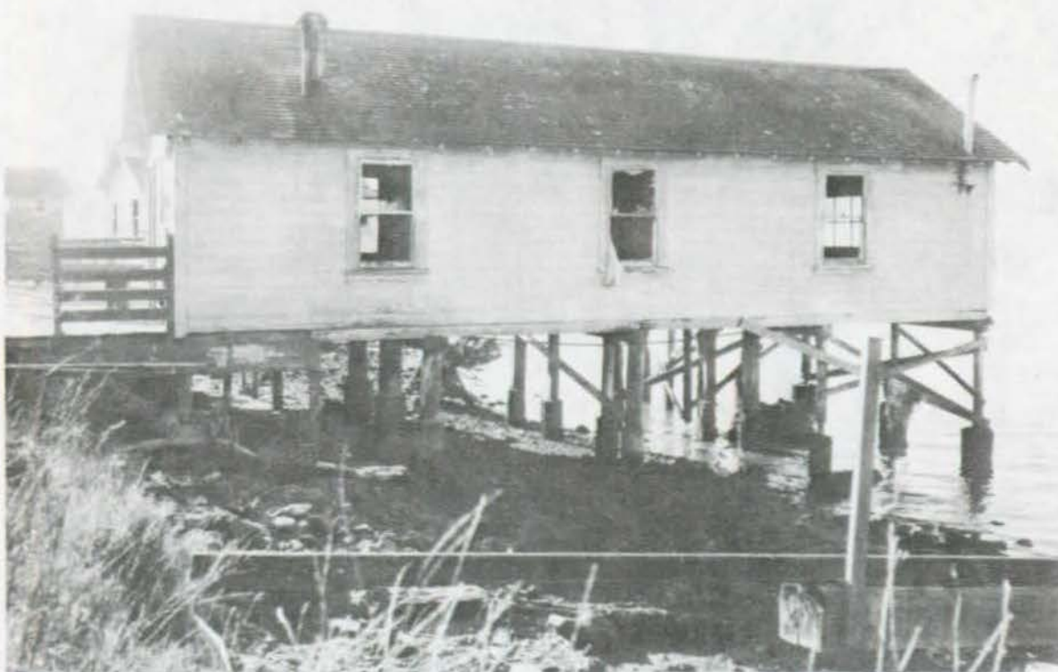
Figure 8 - Structure 5, Bean cabin, north side.
