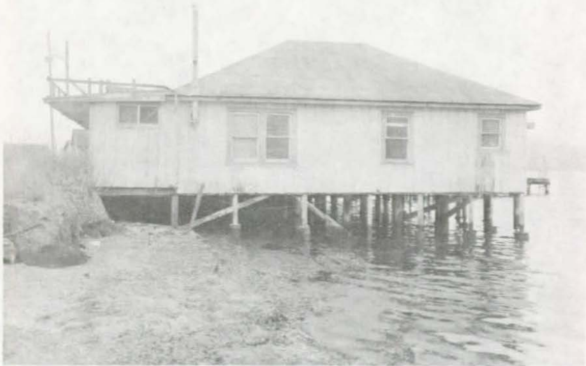
Figure 18 - Structure 10, Jensen house, north side.
