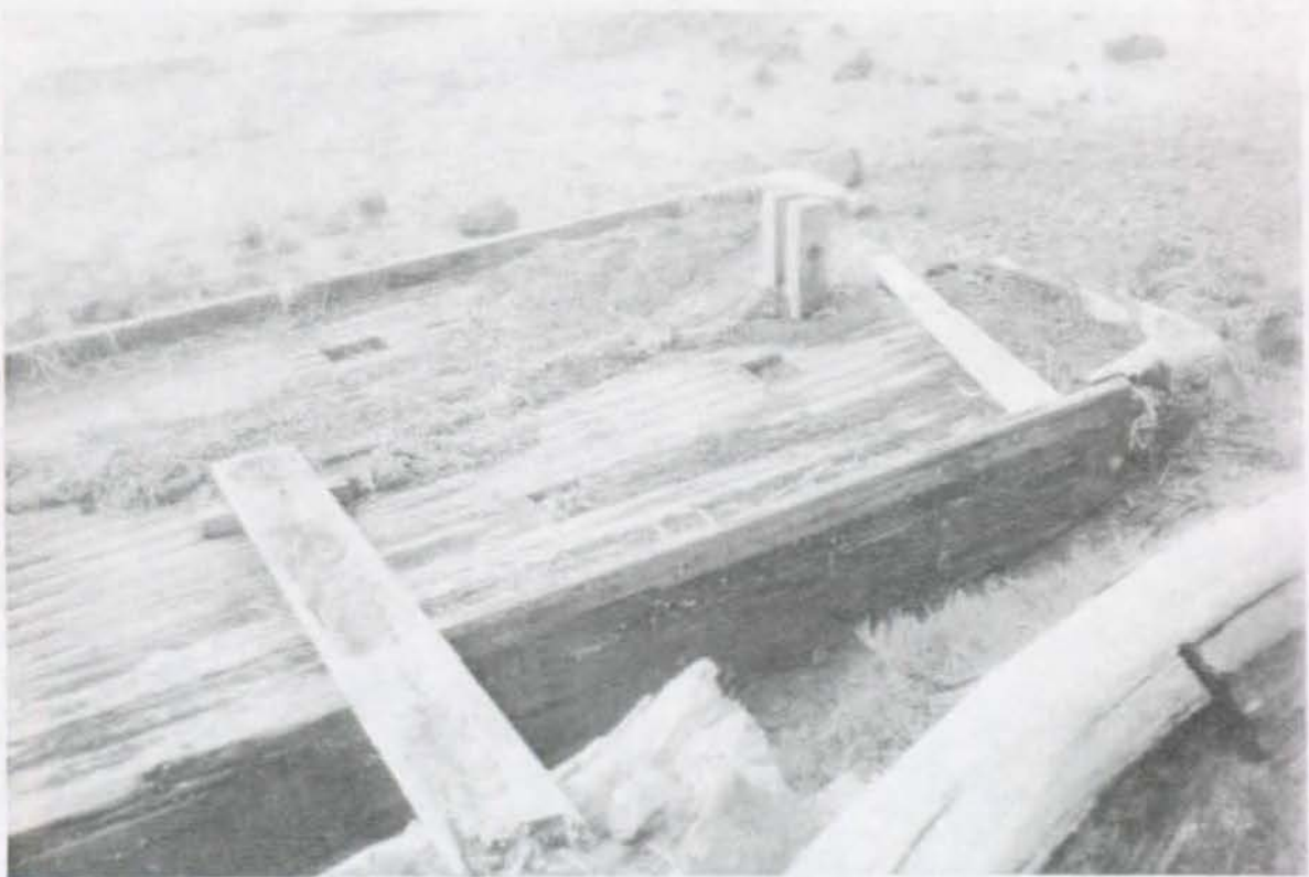
Figure 32 - Structure 20, oyster barge (detail), view to west.
