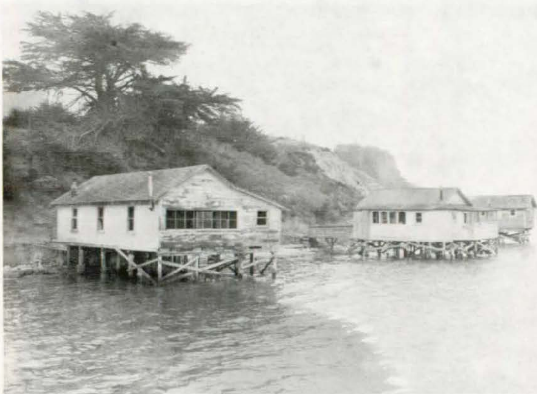
Figure 9 - Structures 5, 3, 2 from wharf, view to southeast.
