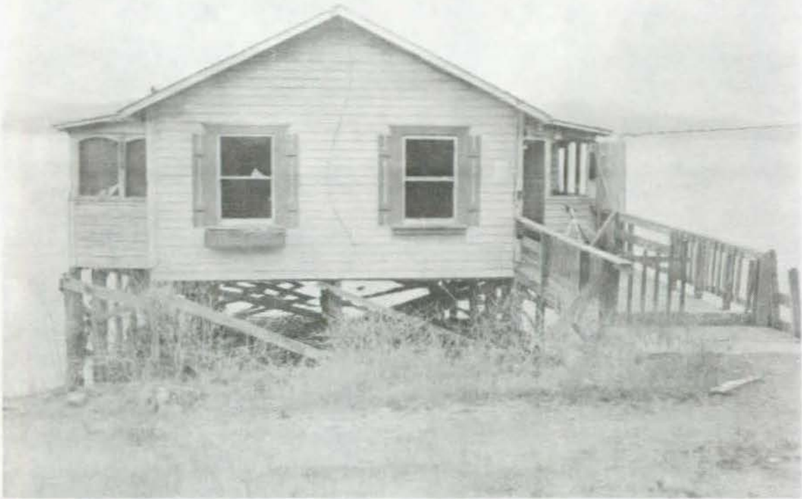
Figure 5 - Structure 3, Lacey cabin, east side.
