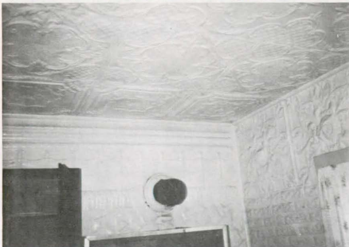
Figure 28 - Structure 17, Spiegel cabin, detail of pressed tin on kitchen walls and ceiling.
