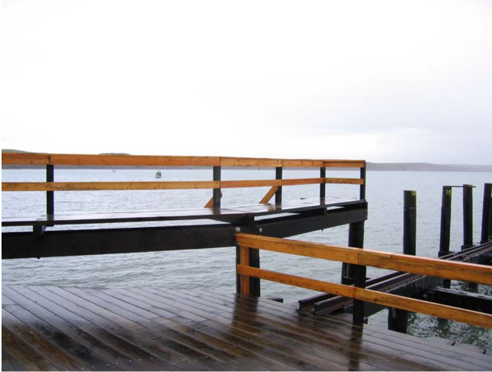
Buildings and Structures No. 3. Marine railway undergoing restoration (PWR Staff 2006).
