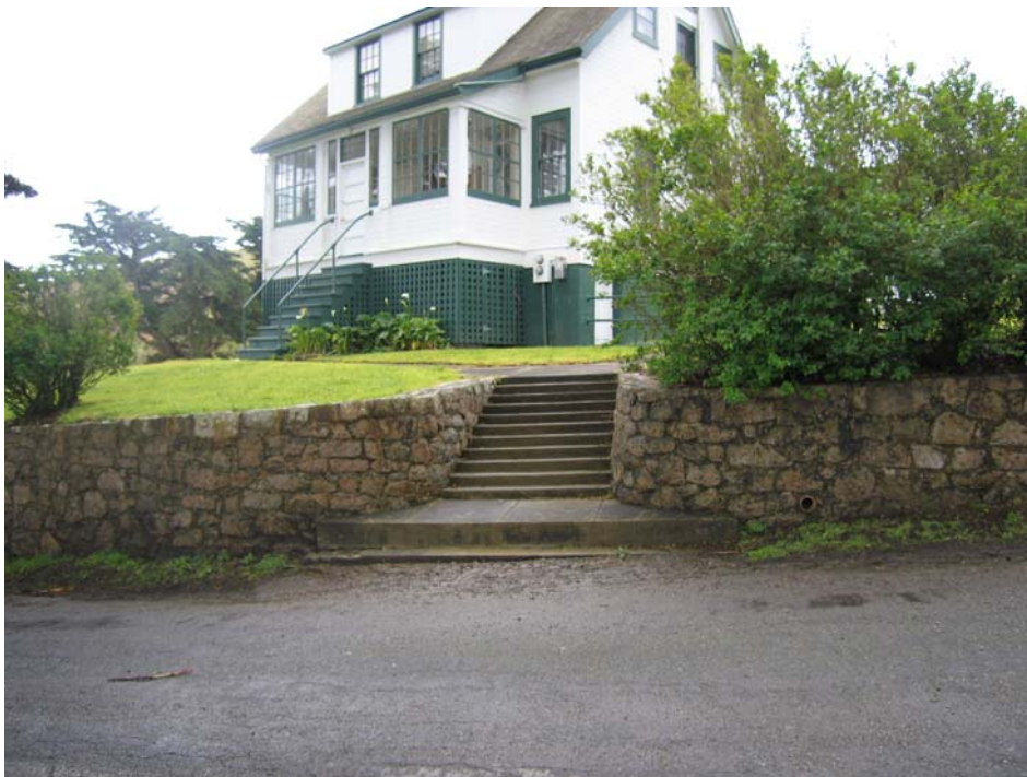
Circulation No. 2: Concrete stairway leading from Boathouse Road to front of Officer-in-Charge quarters. (PWR Staff 2005).
