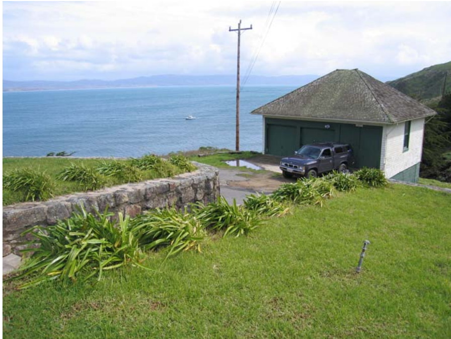
Buildings and Structures No. 1. Front of three-stall garage. Officer-in-Charge quarters' lawn and stairway in foreground. Drake's Bay in background (PWR Staff 2006).
