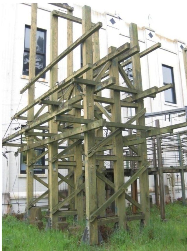
H-Frames leading to the Transmission Line Dead End Structure (Termination Frame) at the back of the Receiving Building. (PWRO 2010)
