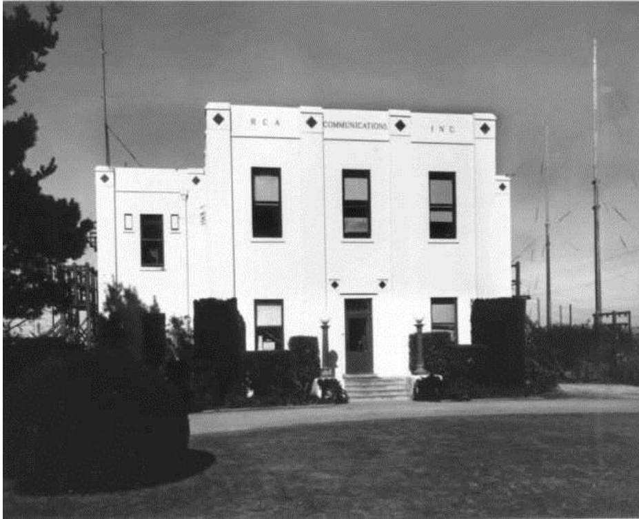
1940s-era photo showing the RCA receiving building and surrounding antennas, looking northwest. (Courtesy of PORE).
