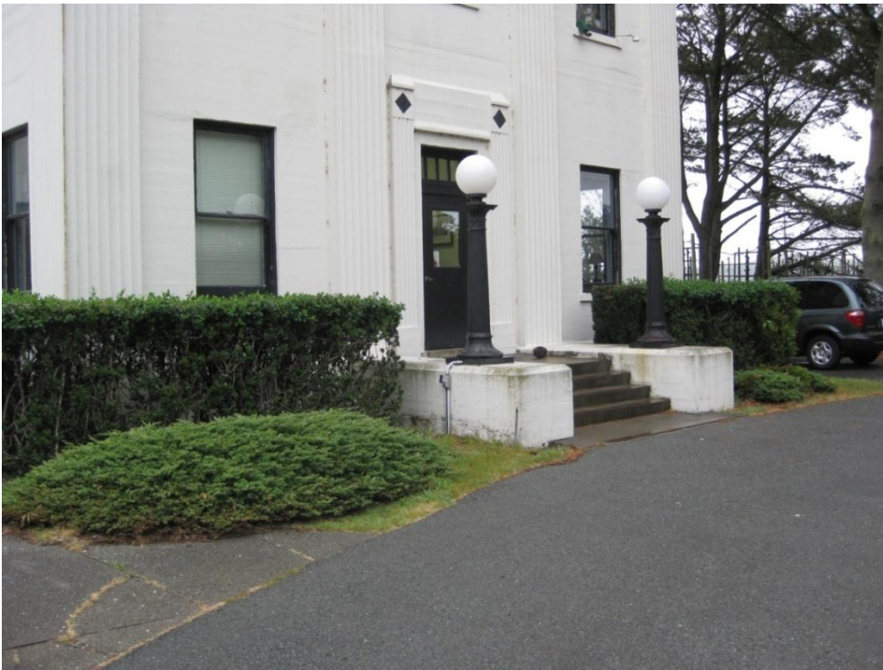
Clipped hedges and juniper groundcover on front side of RCA Receiving Building. The vegetation is non-historic, but the symmetrical plantings and formal clipped evergreen hedges are compatible with the historic character of the site. (PWRO 2009)
