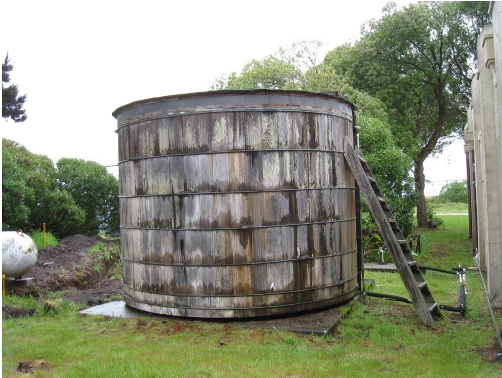
RCA Redwood Water Tank, looking northwest. (PWRO 2010)
