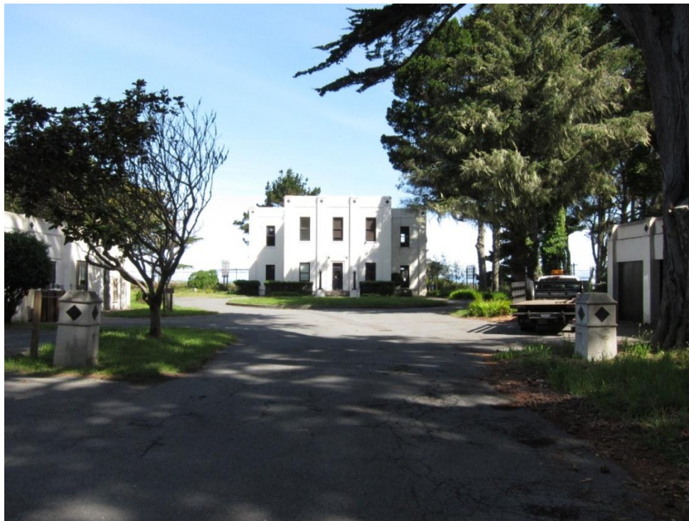
View of the building core that shows the symmetrical layout of the buildings and the foundation plantings around the Receiving Building (center). (PORE 2010)
