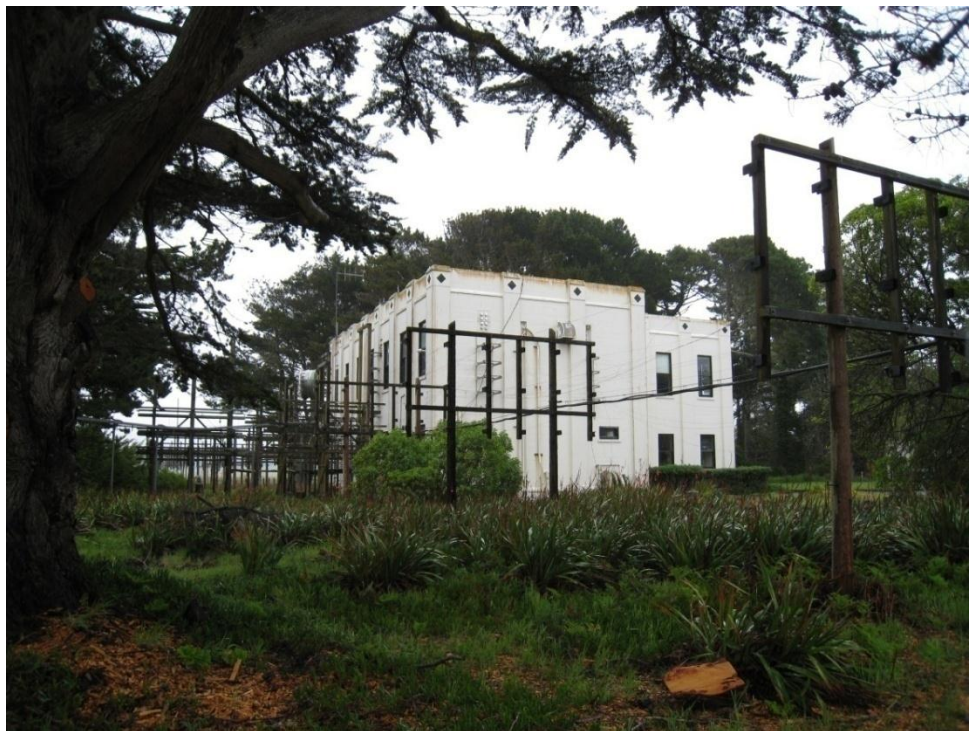
H-Frames leading to the Transmission Line Dead End Structure (Termination Frame) at the back of the Receiving Building. (PWRO 2010)
