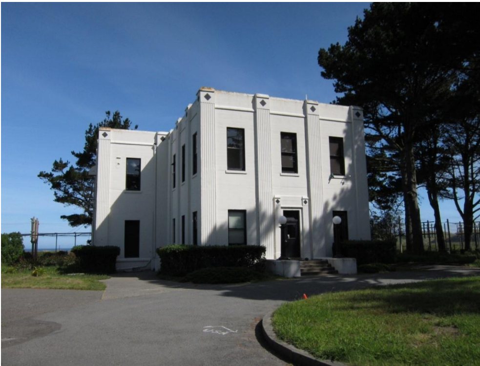
RCA Receiving Building, looking north. (PORE 2010)
