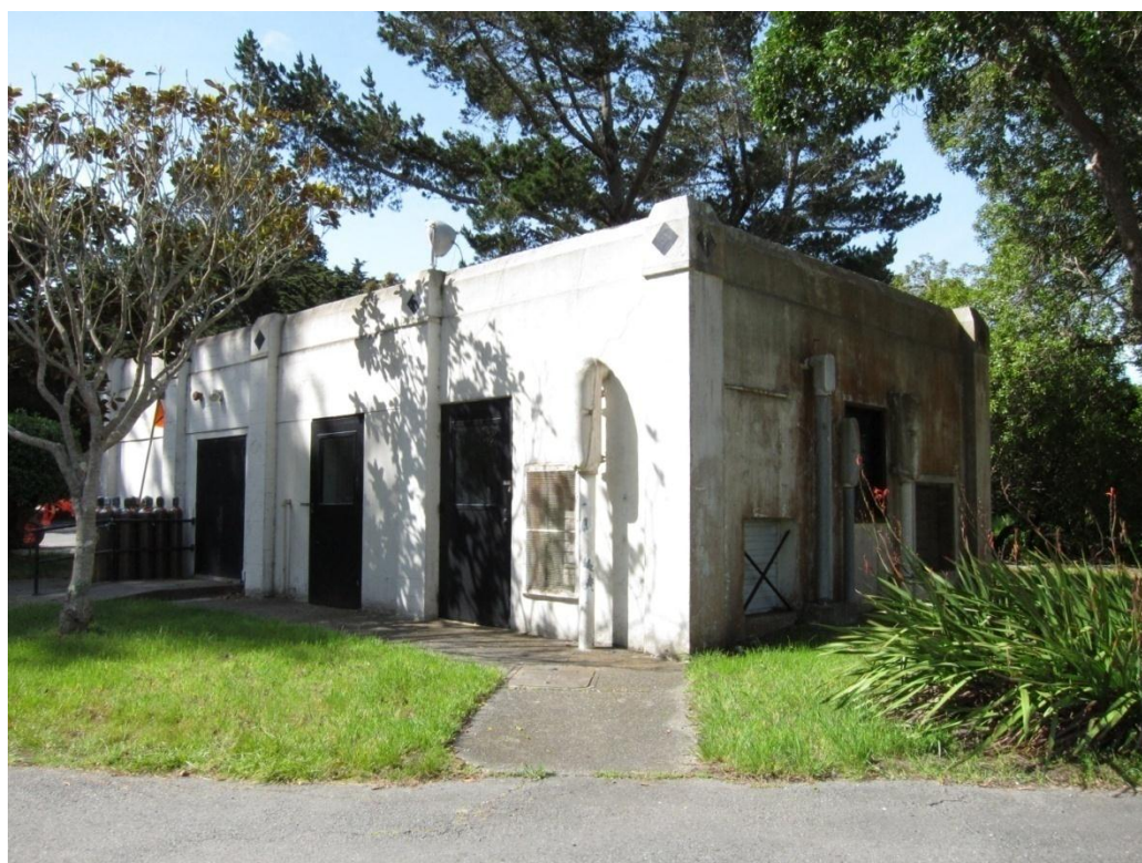
RCA Utility Building, looking south. (PORE 2010)
