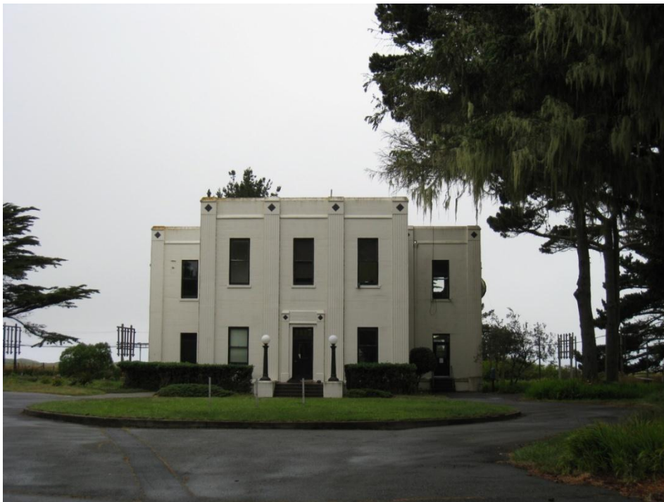
Looped drive at terminus of entrance road in front of the RCA Receiving Building, looking northwest. (PWRO 2010).
