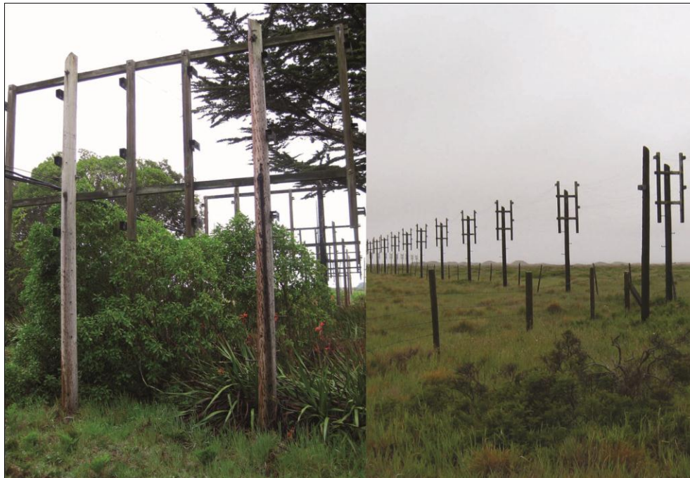
Examples of an H-Frame (left) and T-Poles (right) in the antenna field. (PWRO 2010)
