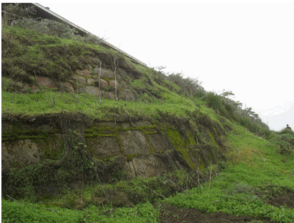
Figure 11. View of two tier retaining wall below Multi-Unit Residence
