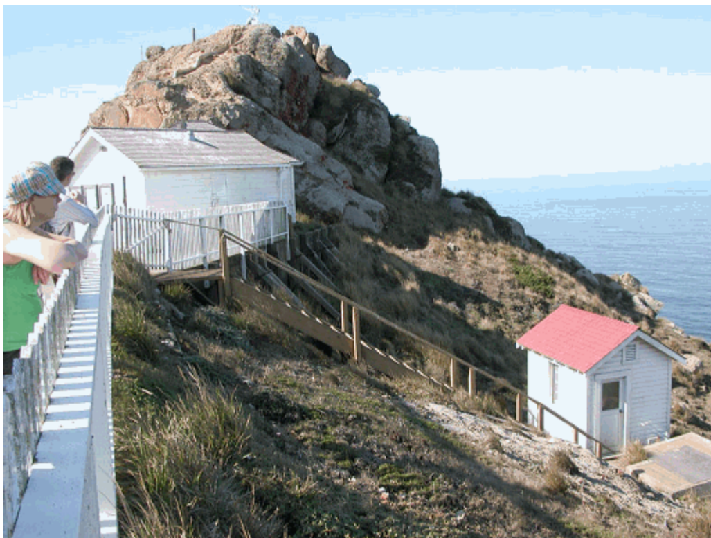
Figure 8. View of the 1934 Pump House with Multi-Purpose Building visible to the left
