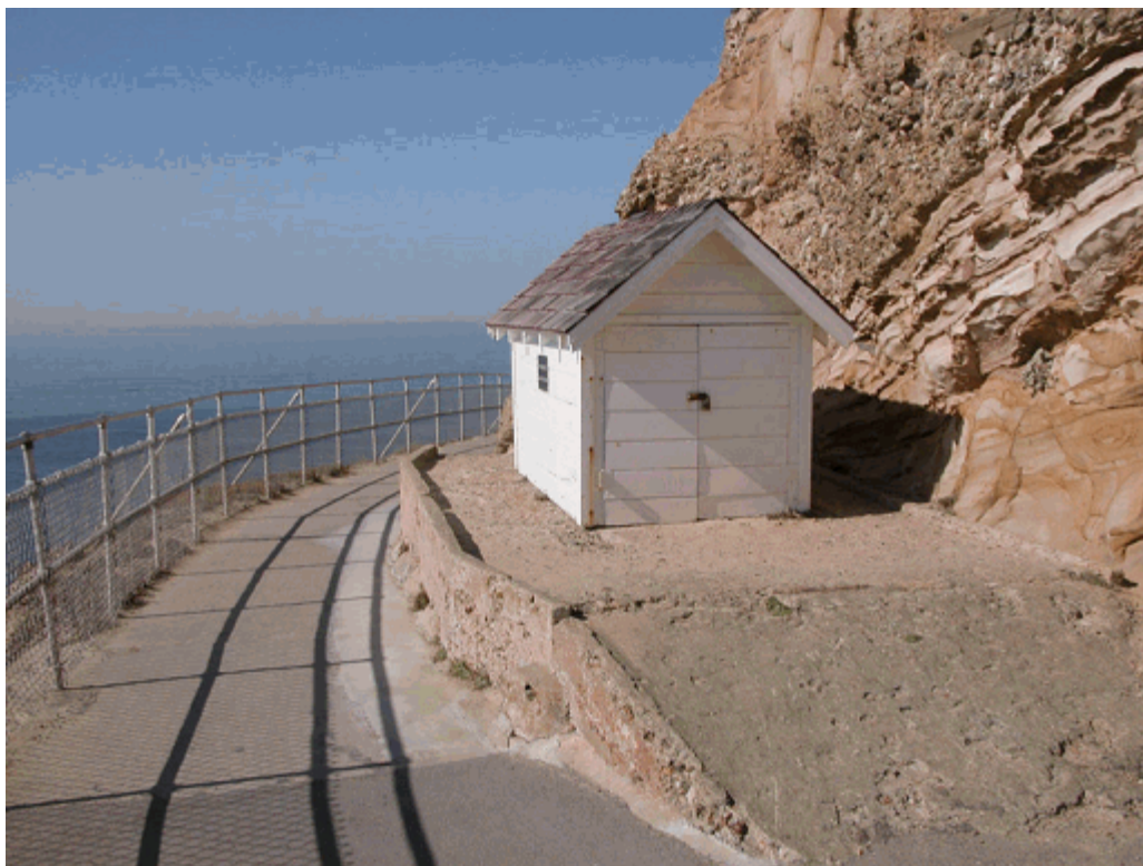
Figure 17. View of westernmost Pump House, near top of Concrete Stairway
