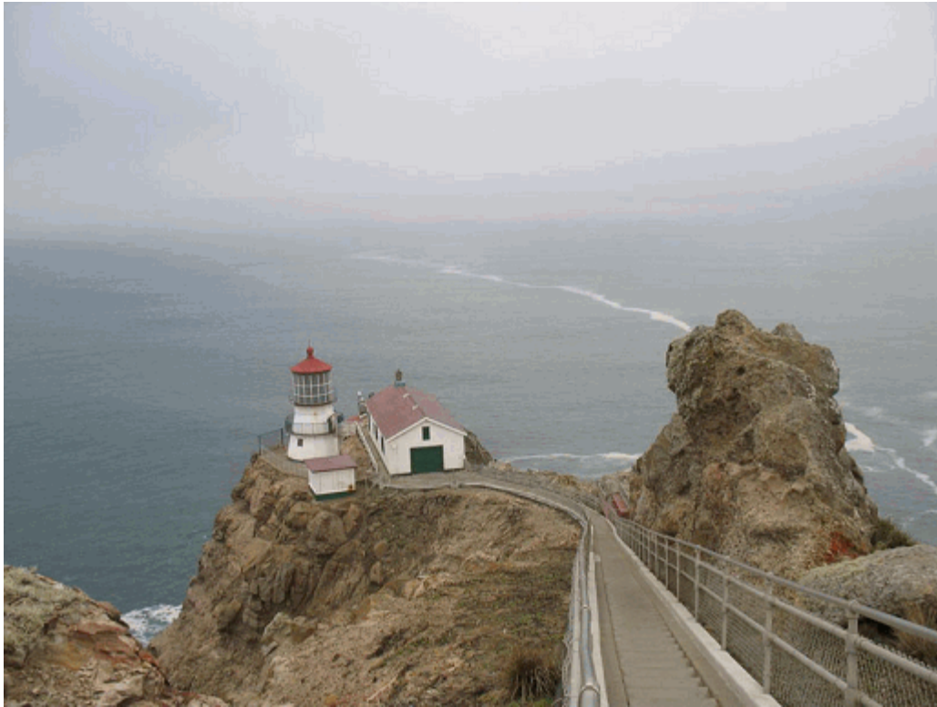
Figure 3. View from the Overlook of the cluster of buildings at the Lighthouse, the rocky outcropping at right is a remnant resulting from intensive blasting at the site
