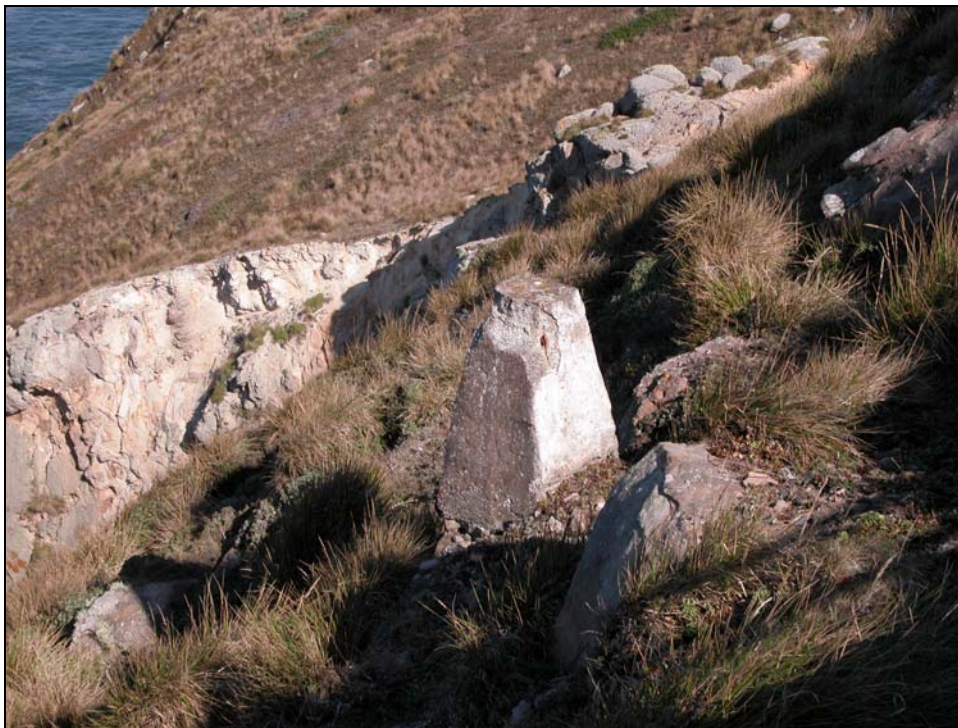
Figure 14. View of concrete pier remnant
