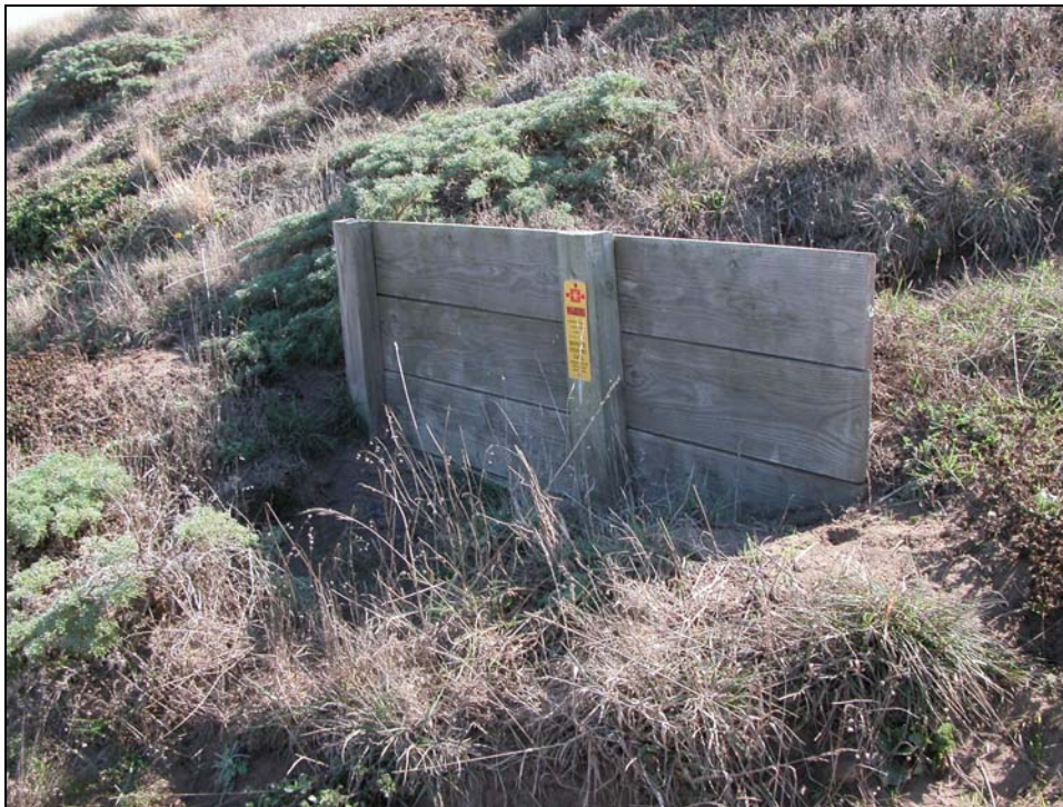
Figure 16. View of modern erosion feature
