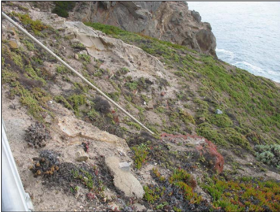
Figure 17. View of brick steps at Wash House site
