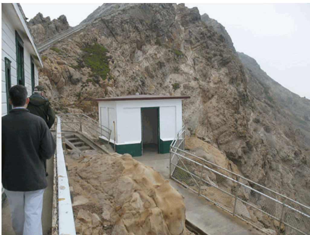
Figure 6. View of the Transformer Building, the Equipment Building is visible at the left and the Concrete Stairway is in the background
