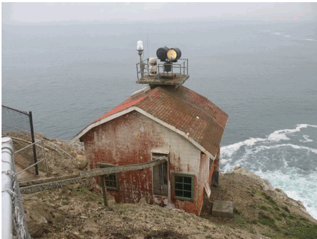
Figure 15. View of the Navigational Aids Building
