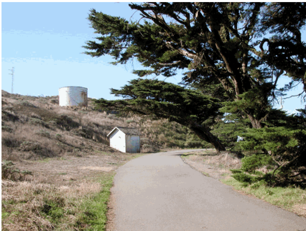
Figure 16. View of easternmost Pump House, with wood Water Tank visible in background
