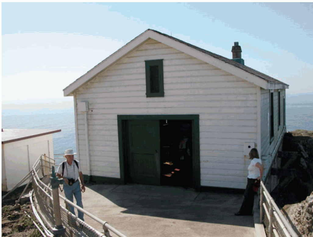
Figure 5. View of the Equipment Building, the Transformer Building is visible at the left
