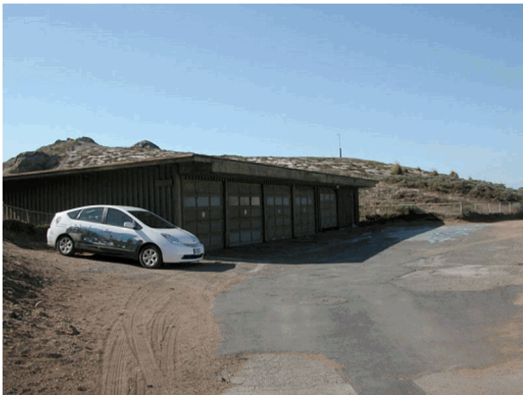
Figure 14. View of the Garage / Shop Building
