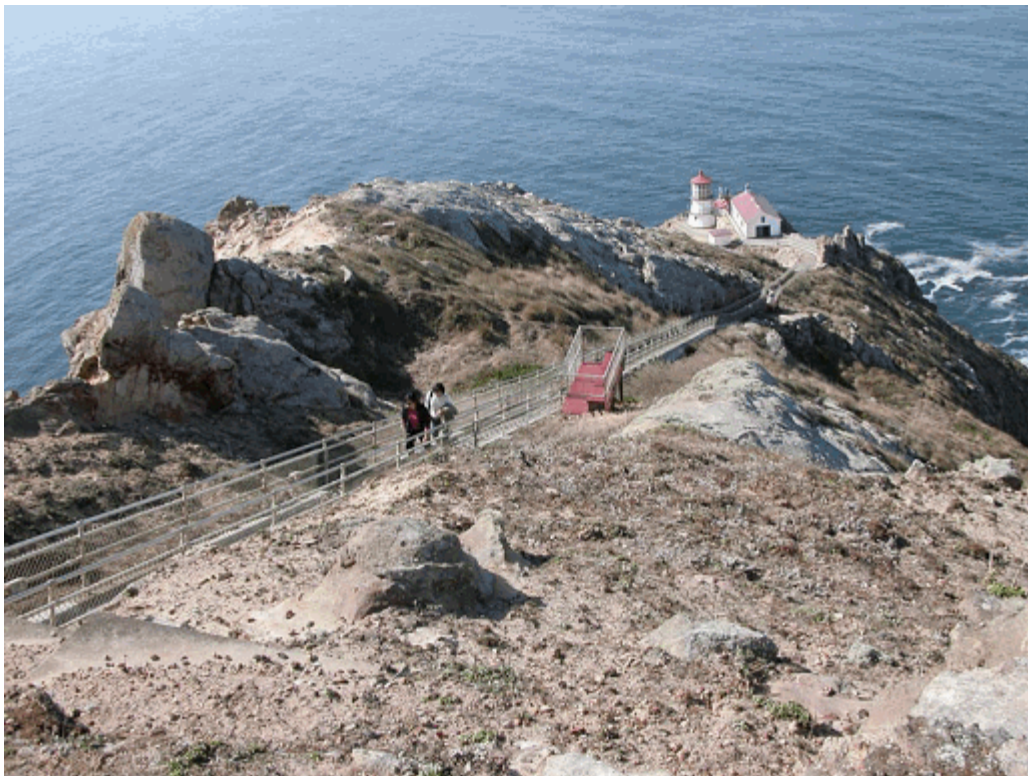
Figure 1. View of linear path down to the Lighthouse, the Equipment Building and the Transformer Building also visible in the distance
