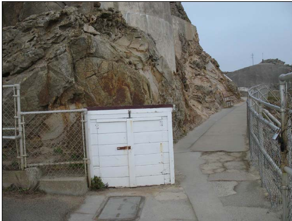
Figure 7. View of Wood Locker, with concrete walls and catchment system in background
