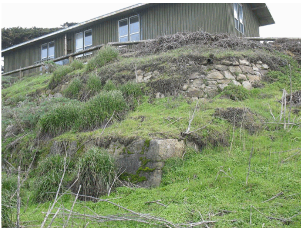
Figure 10. View of two tier retaining wall below Multi-Unit Residence
