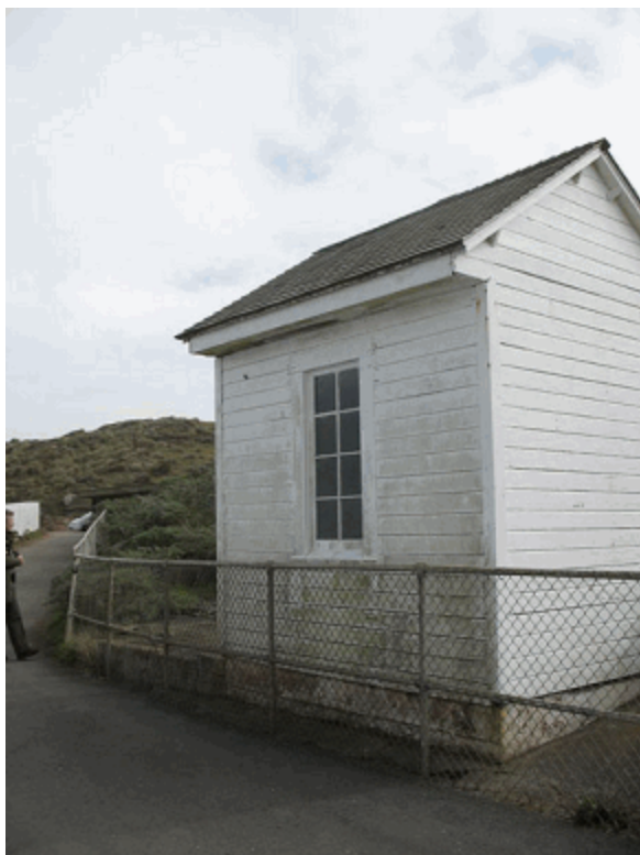
Figure 7. View of Fuel and Paint Storage Building
