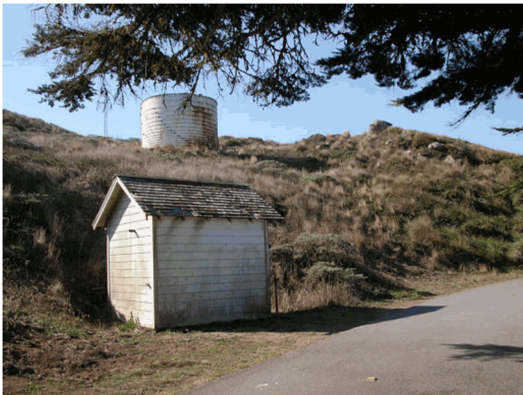
Figure 12. View of wood Water Tank, with Pump House visible in the foreground
