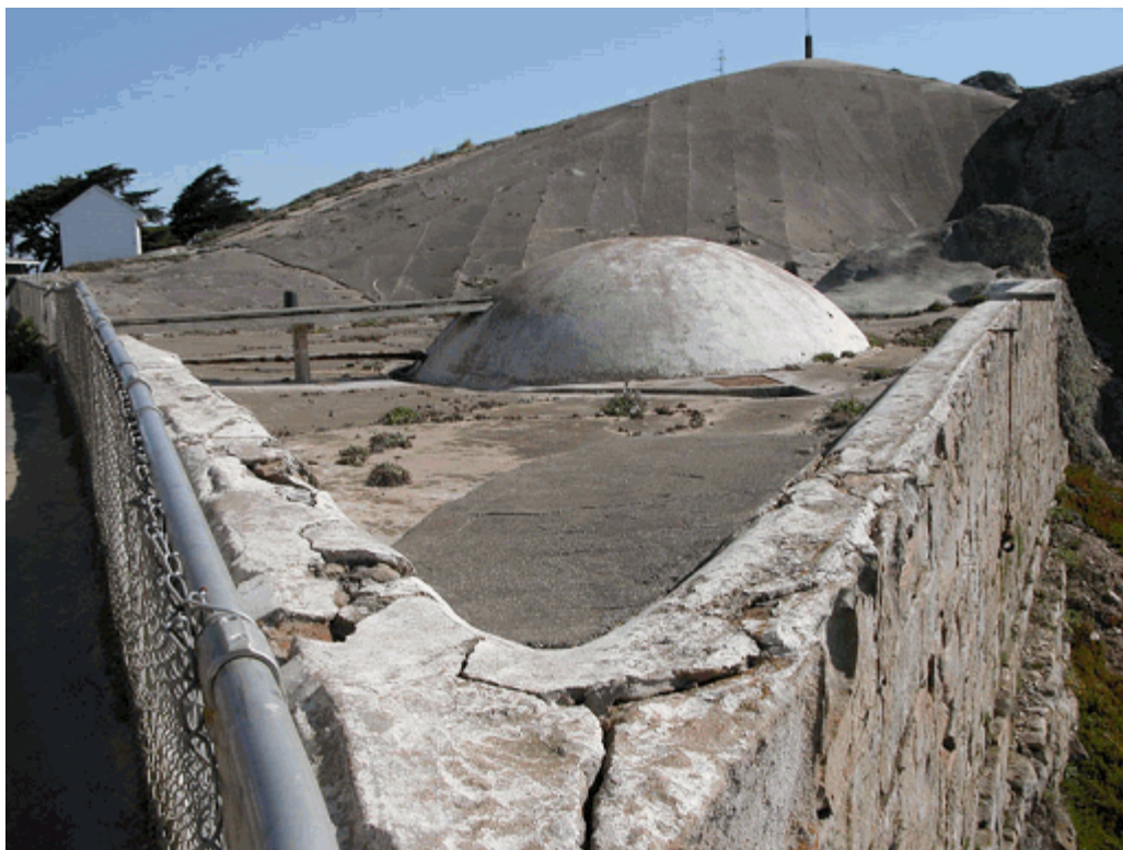
Figure 9. View of 10,000 sf Watershed and Cistern with dome visible in the center
