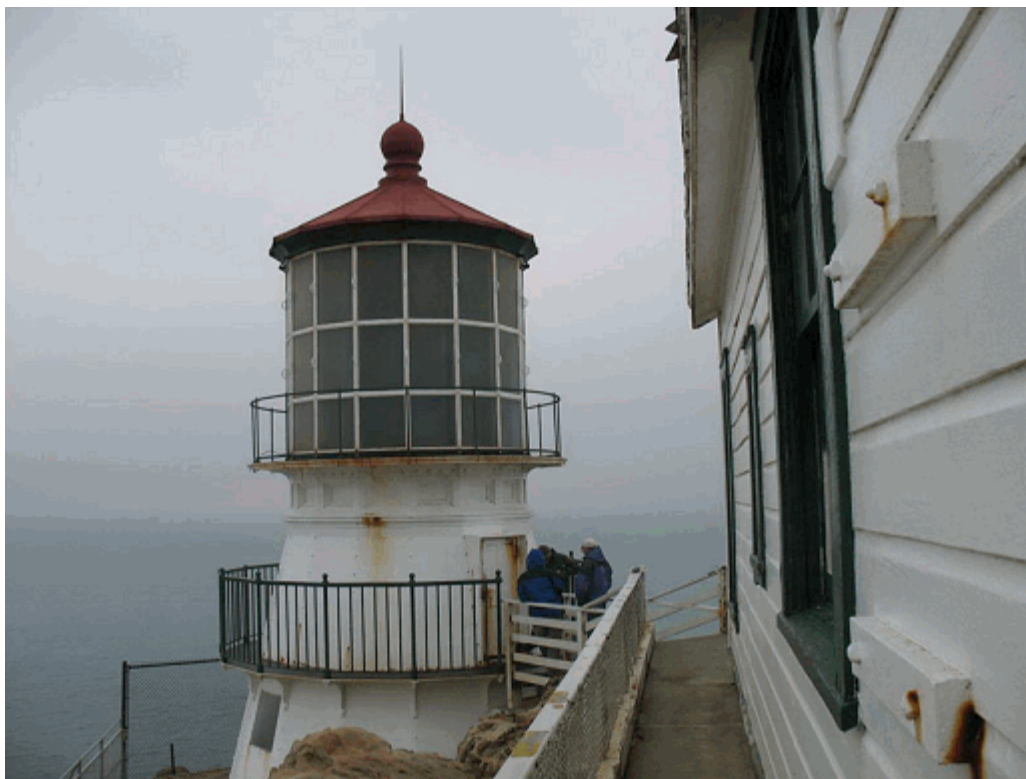
Figure 4. View of the Lighthouse Tower, the side of the Equipment Building is visible at the right
