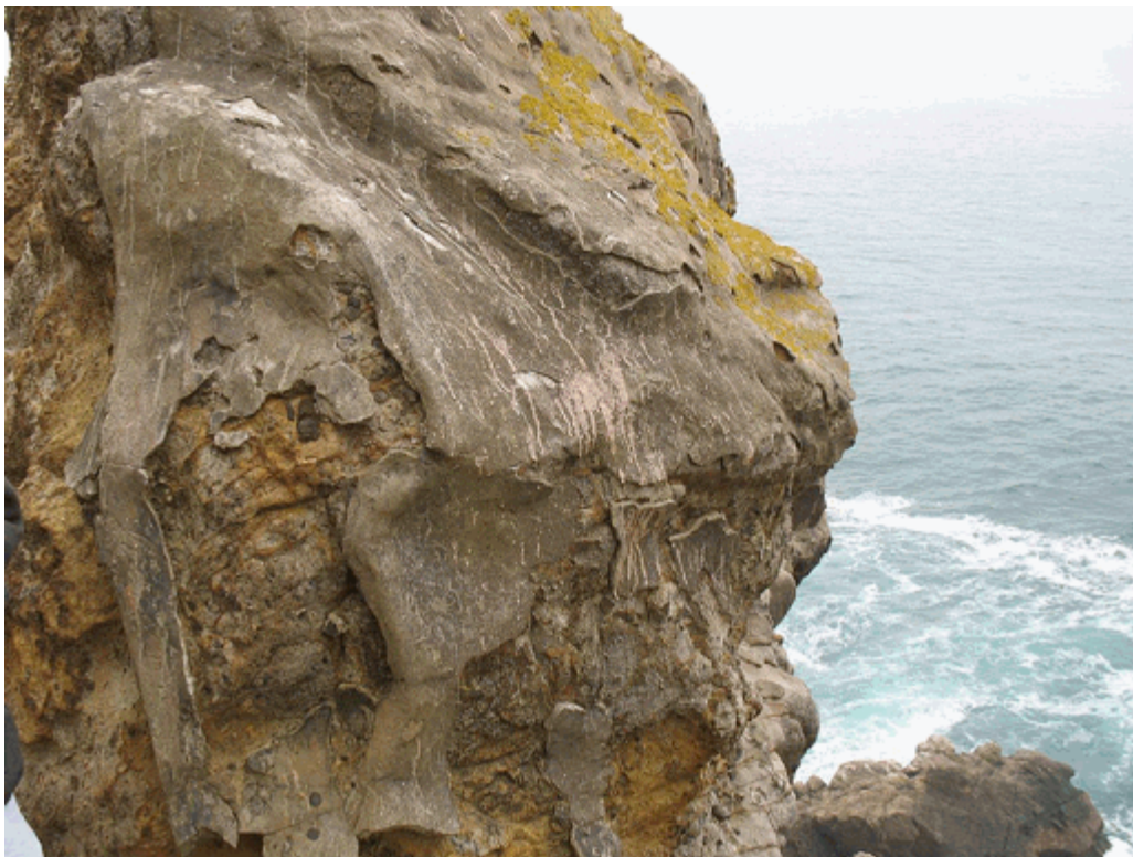
Figure 19. View of cementitious coat used as erosion measure
