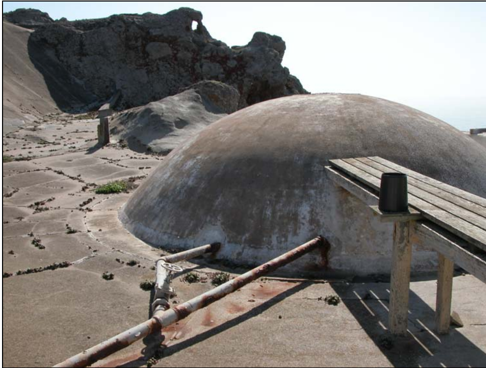
Figure 5. View of the Water Catchment System
