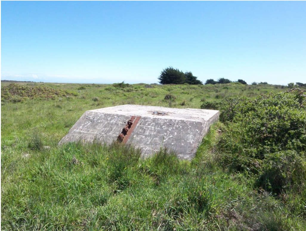
Marconi Antenna Tower guy wire base. (PWRO 2010)
