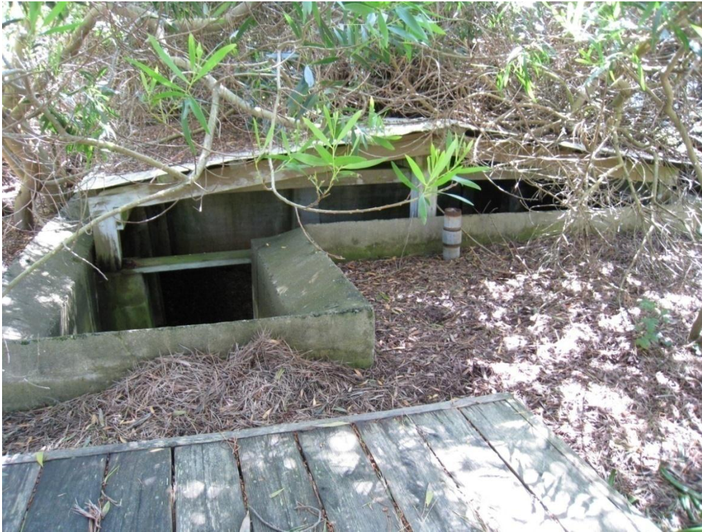
The southwest Cooling Tower Foundation/Reservoir, the northeast reservoir is under the deck seen in the foreground. (PWRO 2010)
