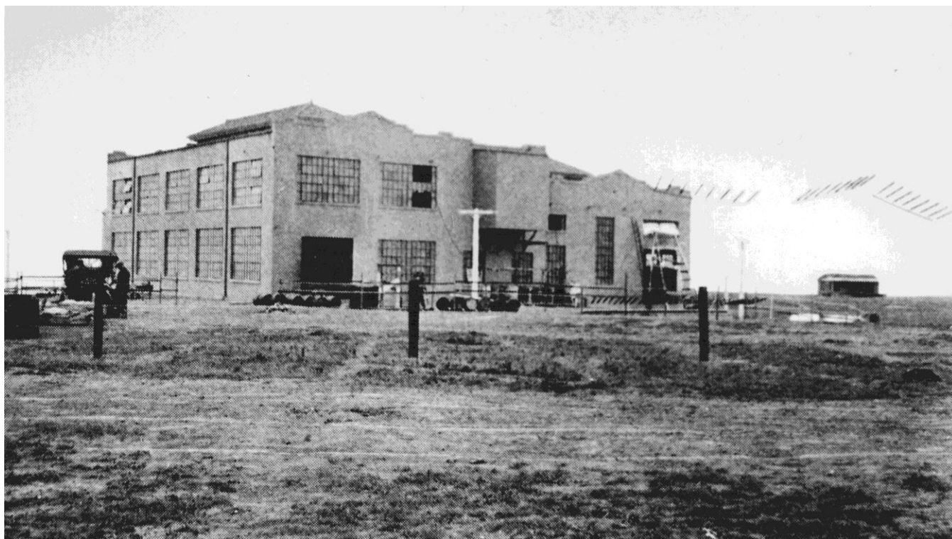
1920s photo of the Marconi Transmitting Building, looking west. (Courtesy of PORE).
