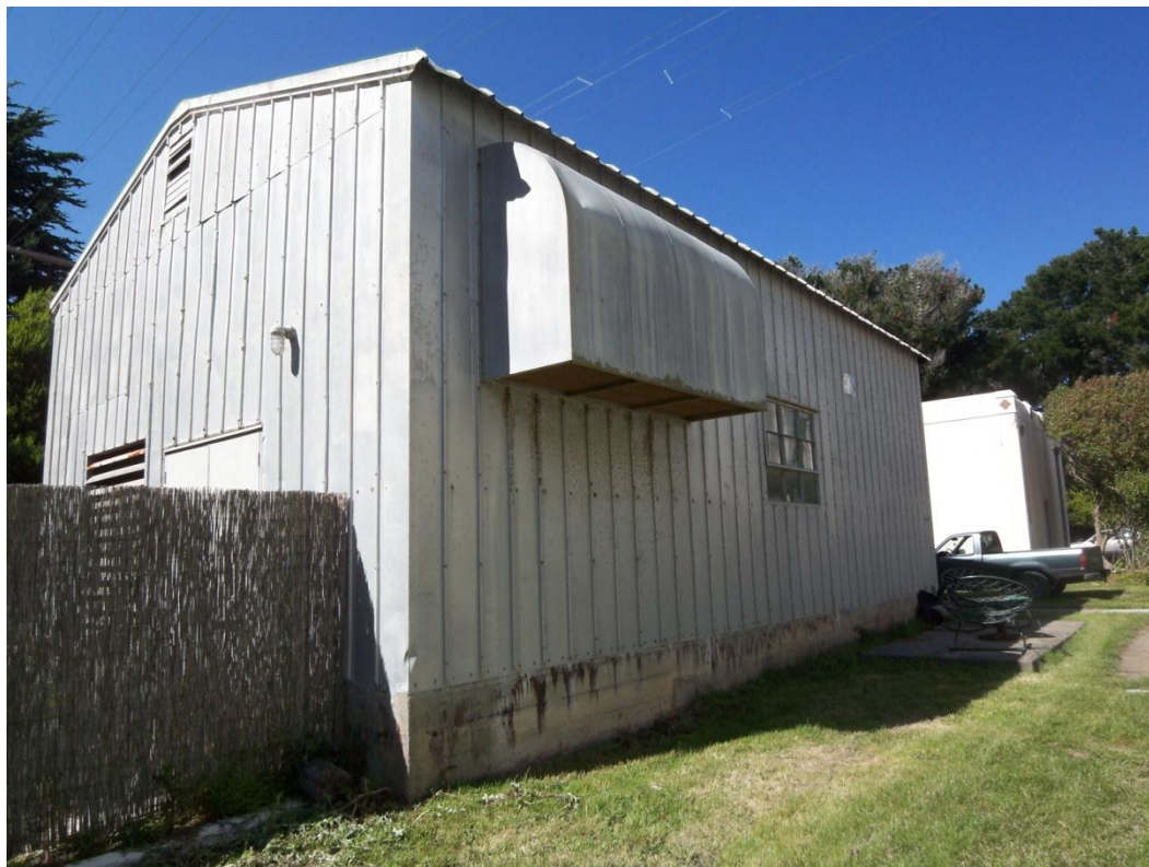
RCA Generator Building, looking northeast. (PWRO 2010)
