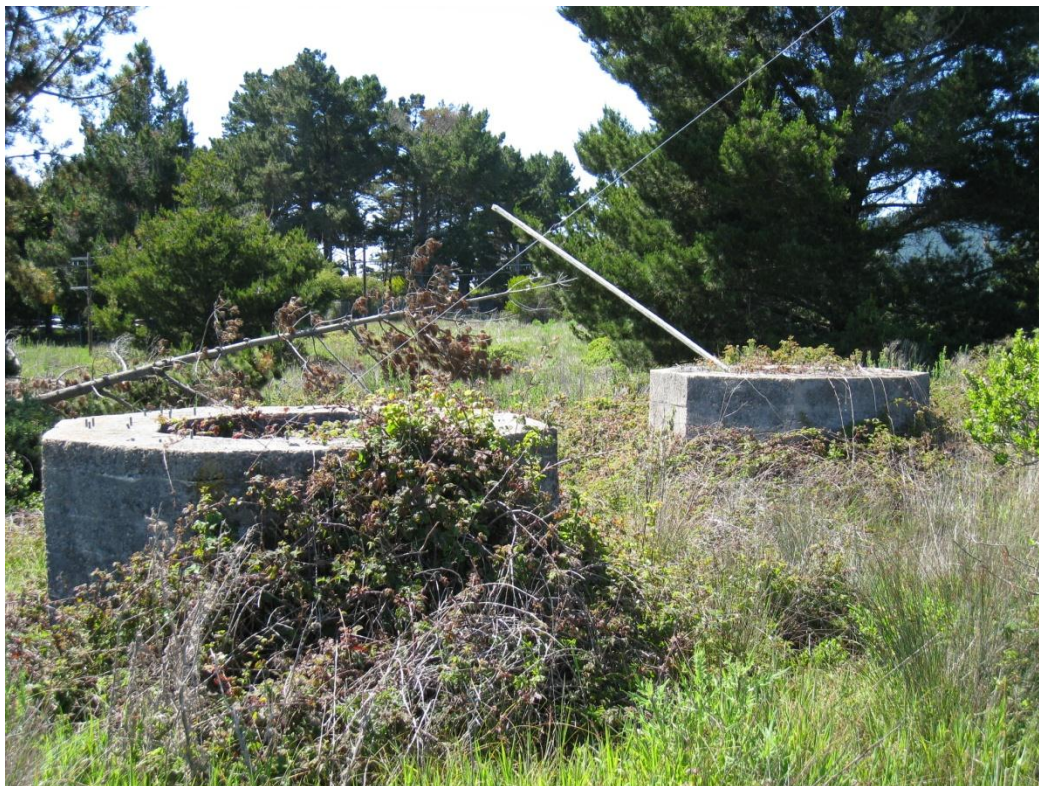
Concrete antenna tuning coil bases located within the antenna field. (PWRO 2010)
