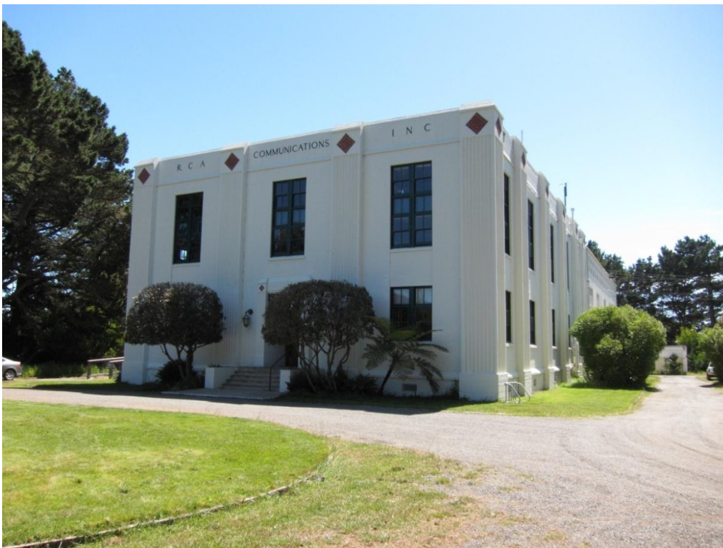
RCA Transmitter Building, looking southwest. (PWRO 2010)
