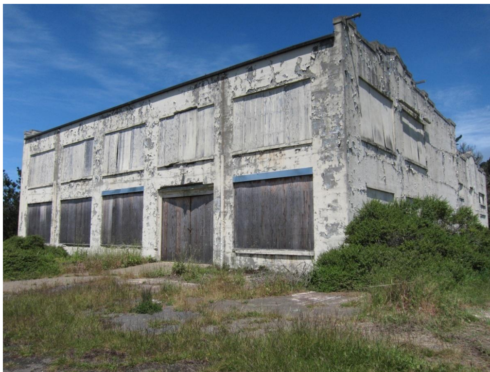
Marconi Transmitter Building, looking northwest. (PWRO 2010)
