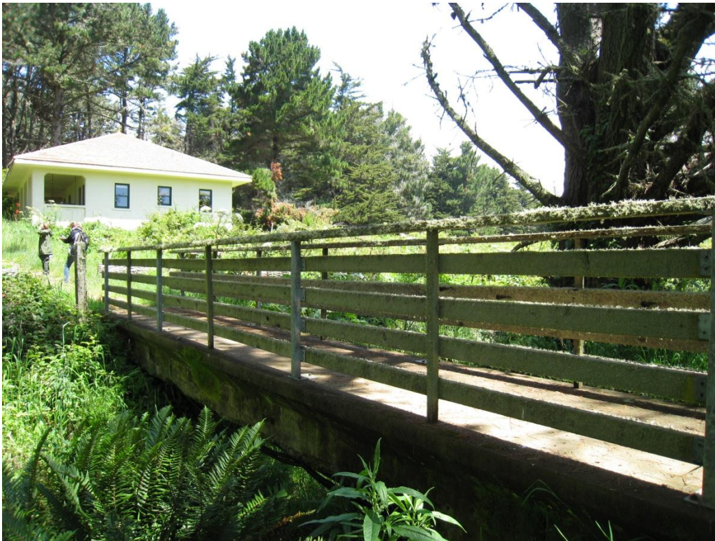
Marconi Pedestrian Bridge, looking northwest. (PWRO 2010)
