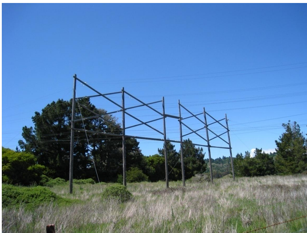
H-frames located within the antenna field. (PWRO 2010)
