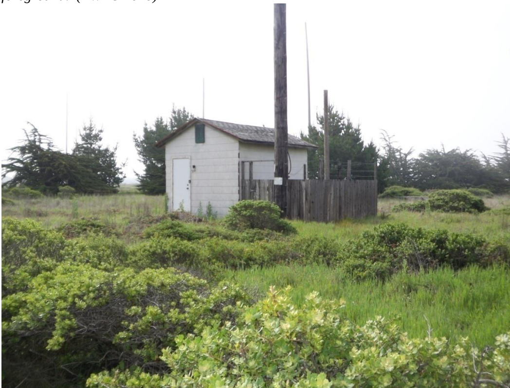
RCA Antenna Tuning Building, looking southwest. (PWRO 2010)
