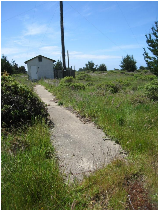
Concrete pathway to the RCA Antenna Tuning Building. (PWRO 2010)
