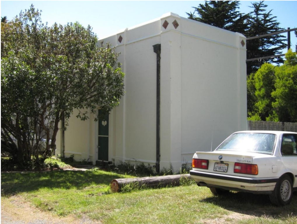
RCA Switching Building, looking west. (PWRO 2010)
