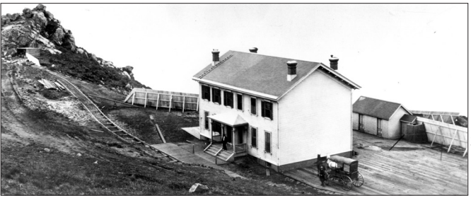
The lighthouse keepers quarters were completed in 1870 and the first keeper, John C. Bull, his wife and family arrived in November 1870.
