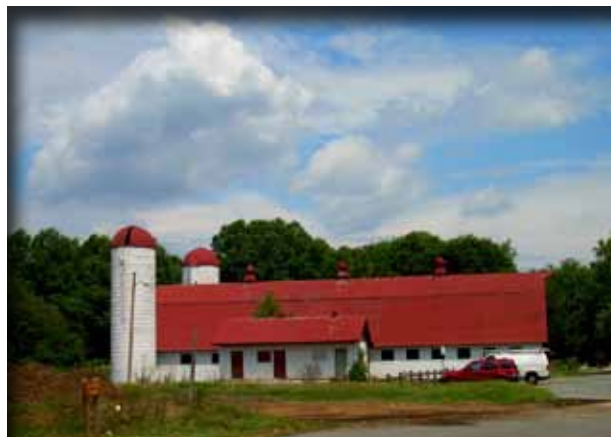
Grist Mill Park Barn, Fairfax County
