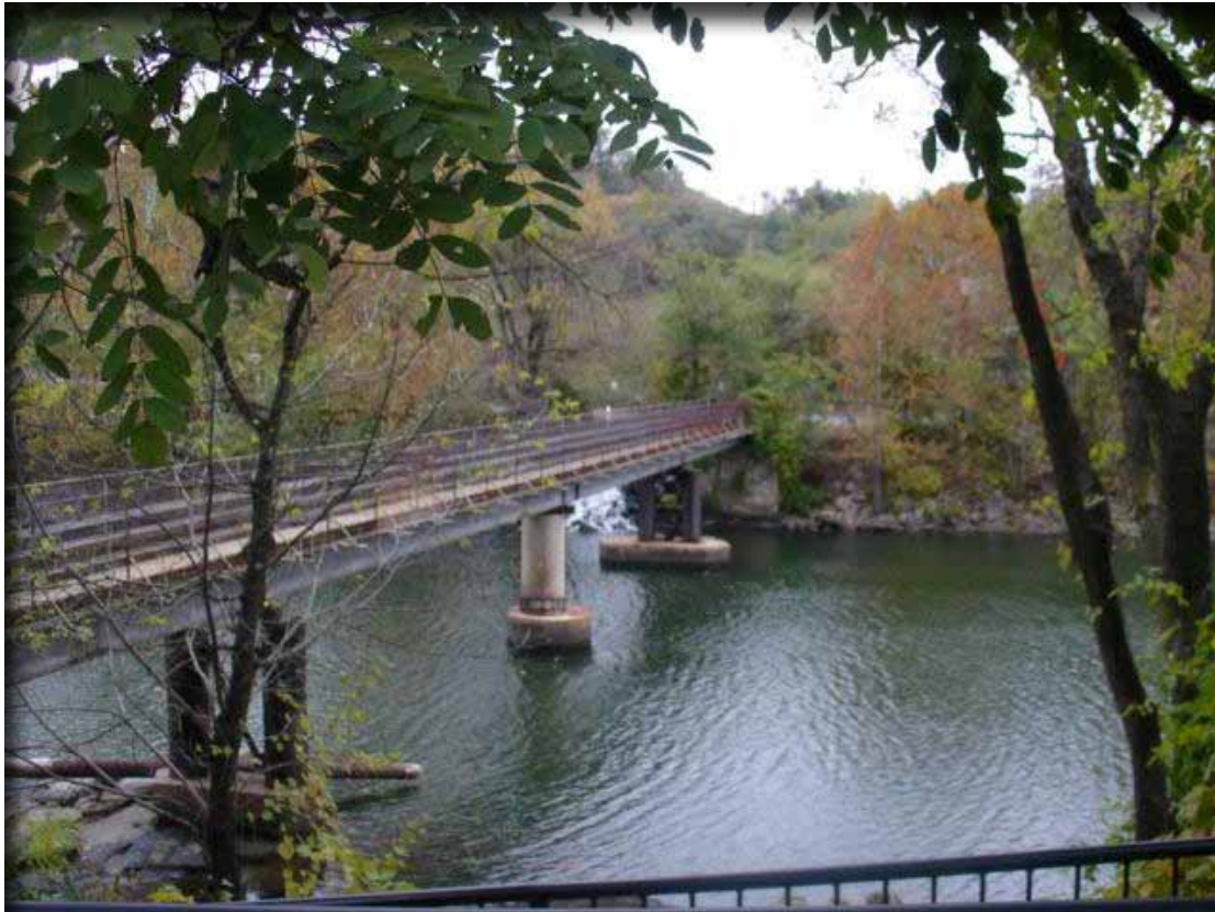
Pedestrian bridge, Town of Occoquan
