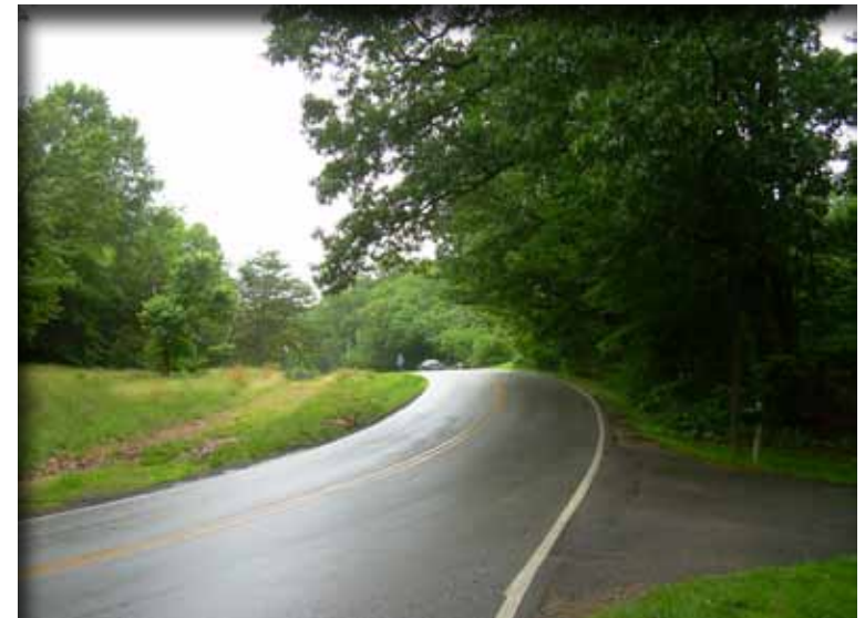
Lorton Road near Ox Road
