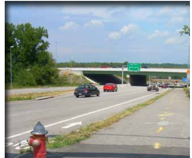
Lorton Road I-95 Underpass, Fairfax County
