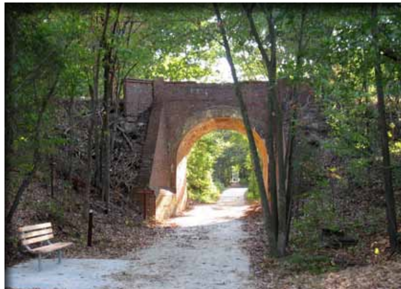
Laurel Hill Greenway Barrel Bridge, Fairfax County
