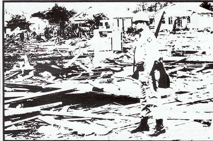
structures (above right). Below are examples of damage on the Naval Magazine.
