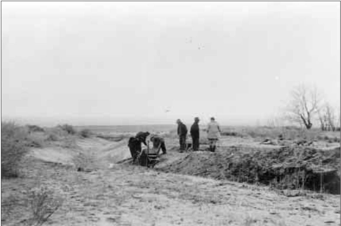
75. Diversion ditch under construction by CCC enrollees to prevent flooding of campground, probably 1936 ( Photograph by Leonard Heaton, Pipe Spring National Monument, neg. 165 )
