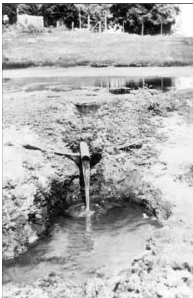
61. Overflow pipe at upper meadow pool, September 1933 ( Photograph by Robert H. Rose, courtesy National Archives, Record Group 79 )
