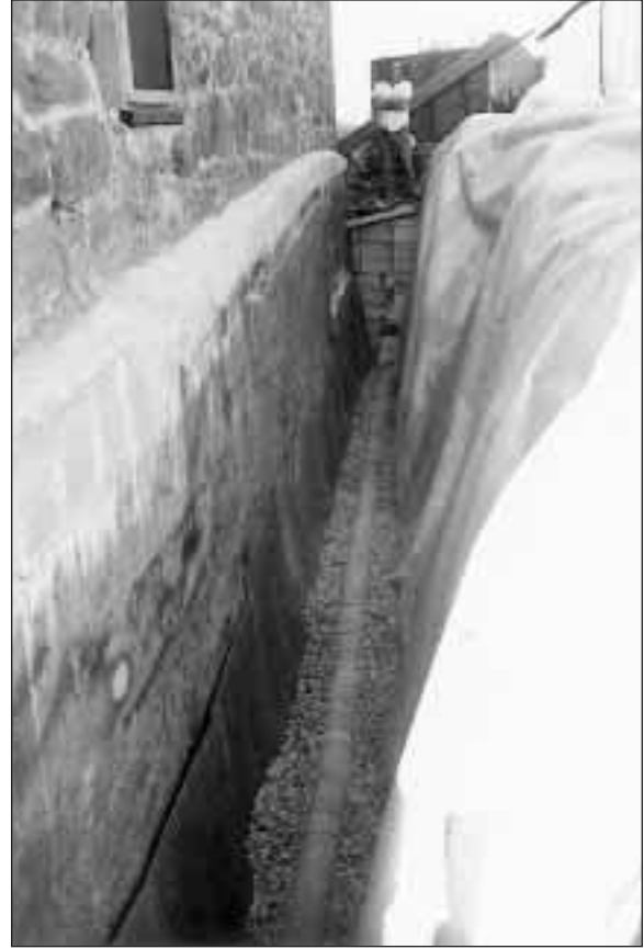
143. Work in progress on the fort's underground drainage system along the north wall, June 1980 ( Pipe Spring National Monument )
