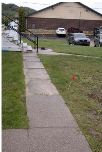
Walkway around rear of dwelling (NPS/Edwards 2019)
