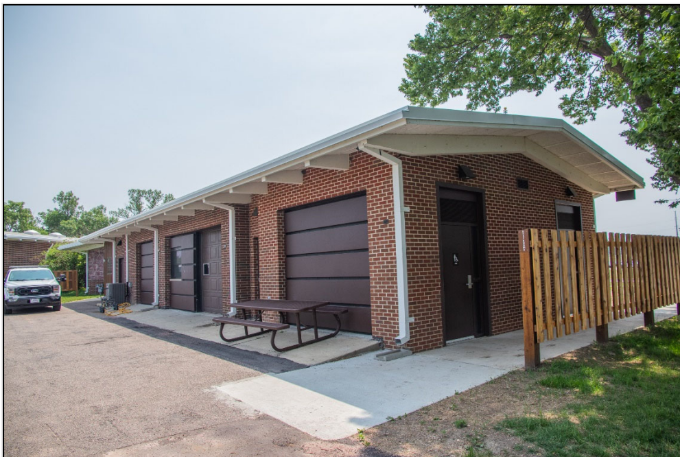
Fig 36. North/northeastern elevation of Visitor Center showing Maintenance Area (NPS 2023)
