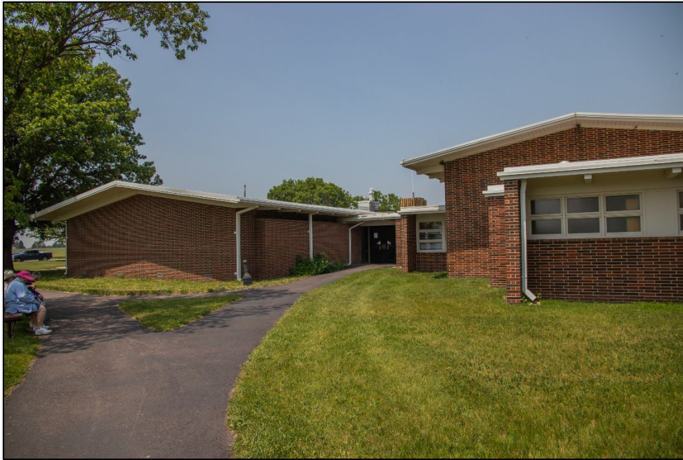
Fig 39. South elevation of Visitor Center and Cultural Center (NPS 2023)
