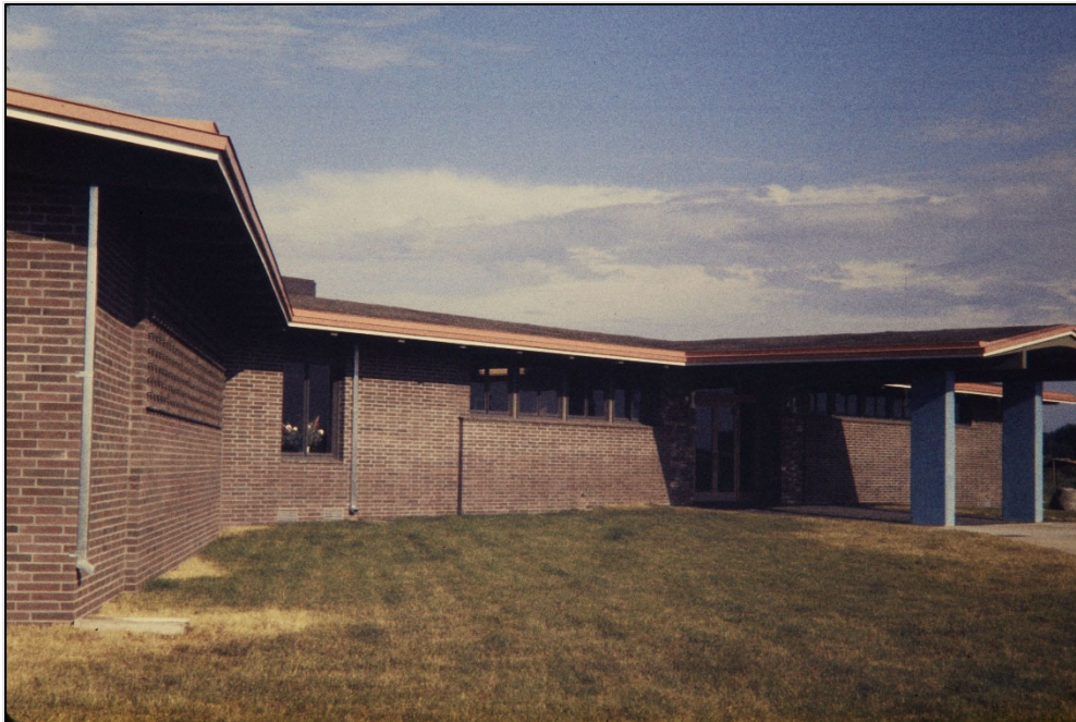
Fig 34. West/northwestern profile of the Visitor Center ca. late 1950s (NPS)
