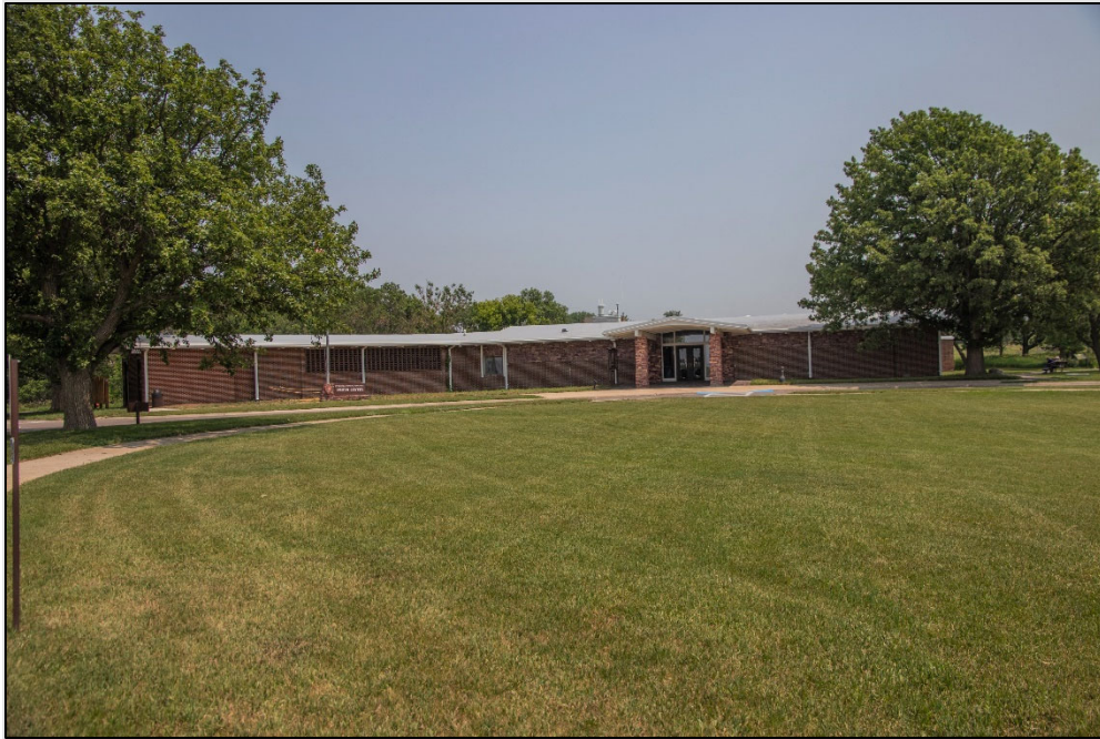
Fig 35. West elevation of Visitor Center (NPS 2023)
