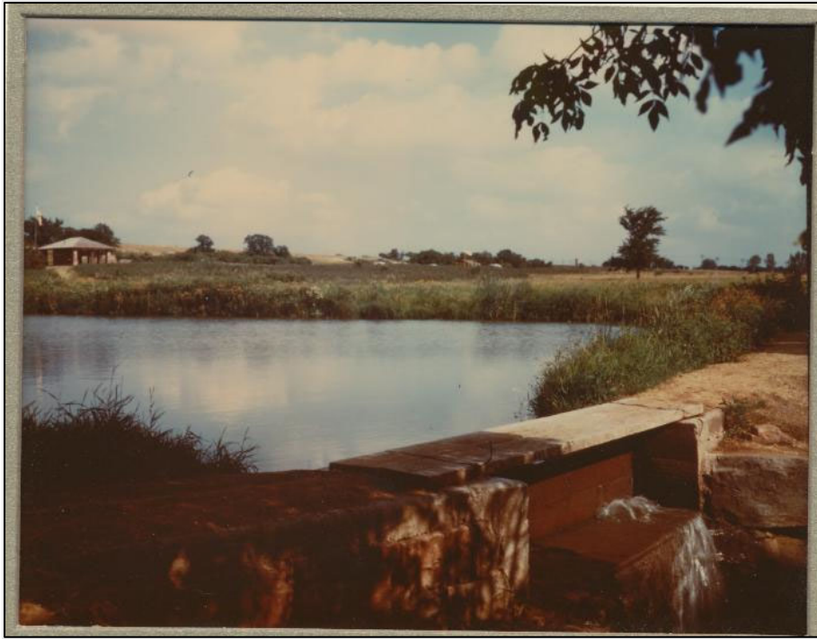
Fig 30. Lake Hiawatha/1963 Dam ca. early 1960s (NPS)
