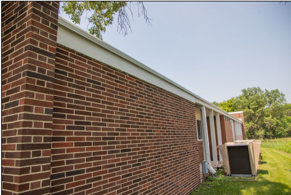
Fig 38. East elevation of Cultural Center (NPS 2023)
