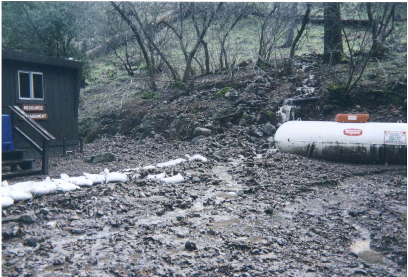
Figure 28. Photograph of mass wasting damage at headquarters building. This photograph shows an example of the damage to facilities that slope movements can cause, especially when combined with water as in this debris flow in 1998. Photograph from Troost (2003, figure 1).
