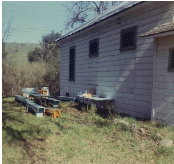
Physical History #6 Photo at left shows north wall of schoolhouse viewed from northwest corner, ca. 1915. Photo at right shows same wall, ca. 1960. Note that two of three original double-hung, four-over-four window have been shortened to accommodate blackboard inside. [Both photos from private collection of Jane Lausten.]
