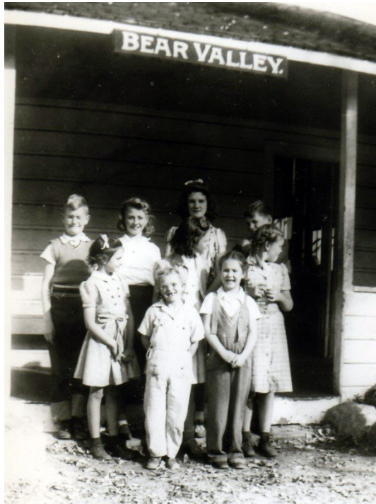
Physical History #7 View from northwest showing detail of front porch, 1942. Note that porch has been modified sometime between 1923 and this date. It is now lower, with only a single step, and has enclosed toilets on either side. The open railing has been replaced with a solid half-wall, and the boxed pillars with an unadorned four-by-four post. [Private collection of Bernice D'Arcy.]
