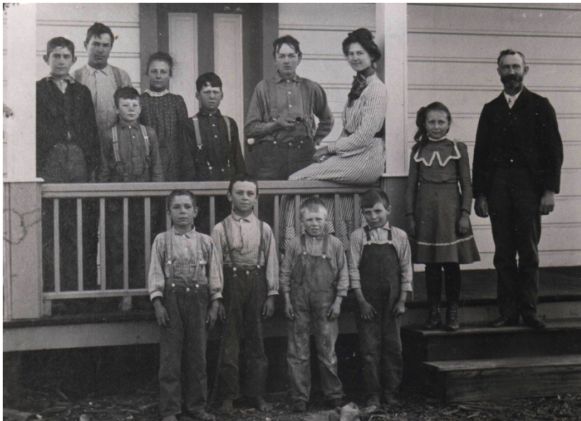
Physical History #4 View from west showing detail of front porch, ca. 1905. [Private collection of Jane Lausten.] Note open railing and square pillars. Horace G. Bacon is the older man standing at the far right.
