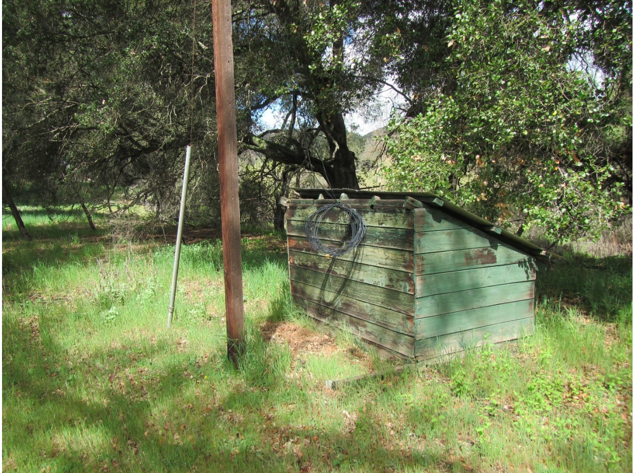
Buildings and Structures #5 Electric Pump/Wooden Shed-Style Pump House, view north. (NPS, March 2020)
