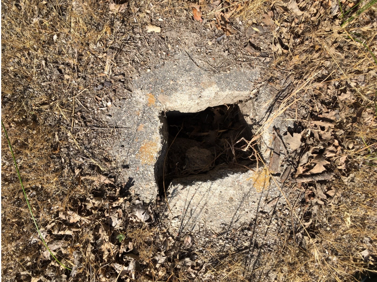
Buildings and Structures #9 Concrete socket of 1940s flagpole, located in front of the Bear Valley Schoolhouse. (NPS, June 2020)
