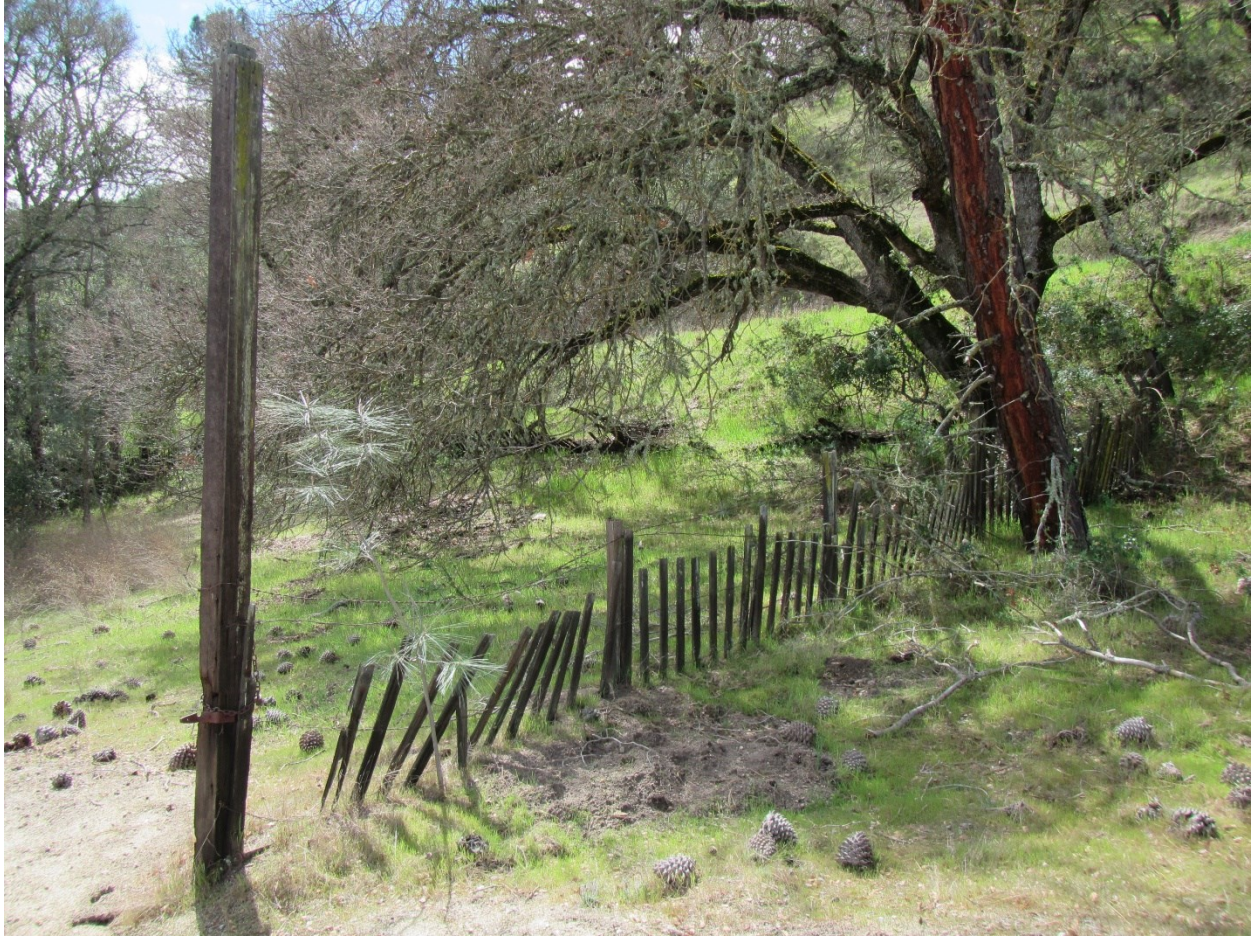
Buildings and Structures #4 1895 Redwood stave and wire perimeter fence, view north. (NPS, March 2020)
