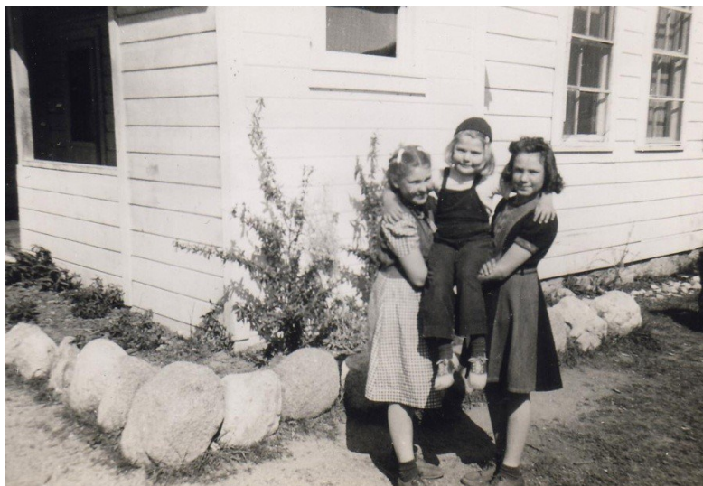
Physical History #8 View from southwest showing detail of porch and portion of south wall, 1942. Note enclosed toilet (girls on the south end, boys on the north). The window on the exterior wall of the toilet room will later be replaced with a louvered vent. Note also the foundation plantings and river stone border. The border is no longer present. [Private collection of Bernice D'Arcy.]
