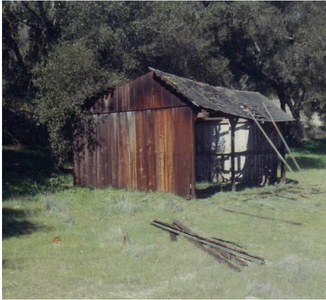
Physical History #11 Old storage shed seen from southeast (rear) corner of schoolhouse just prior to demolition, ca. 1960. This building was constructed during 1890s of redwood lumber salvaged from original 1873 schoolhouse. Demolition was carried out by local 4H volunteers as part of annual clean-up day. The debris was later burned. [Private collection of Jane Lausten.]
