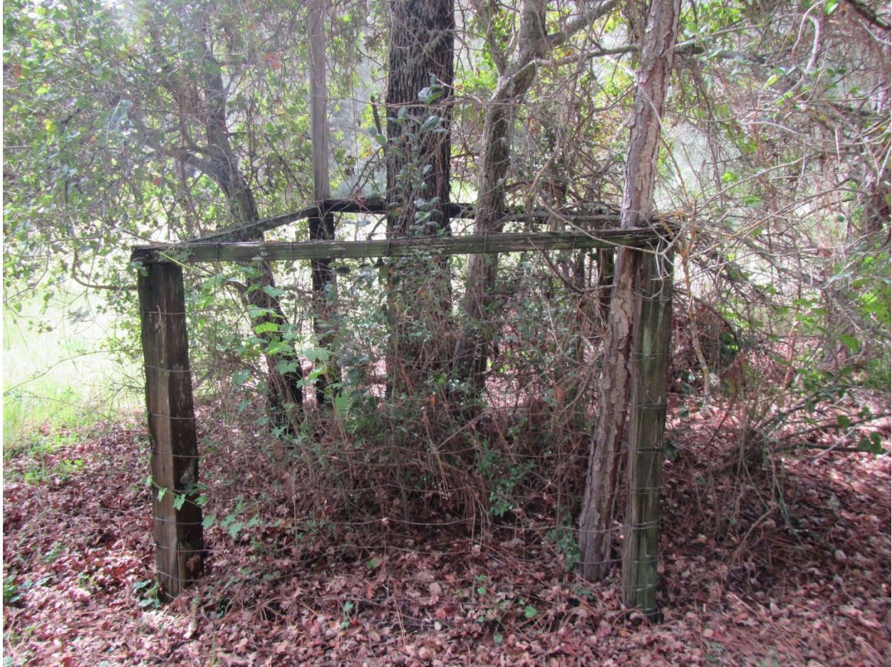
Buildings and Structures #2 Horace Bacon Commemorative Tree Exclosure, view southwest. (NPS, March 2020)
