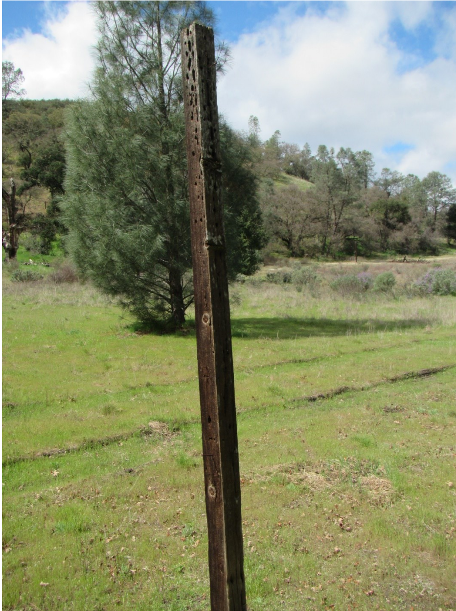
Buildings and Structures #8 Wood pole, view southeast. (NPS, March 2020)
