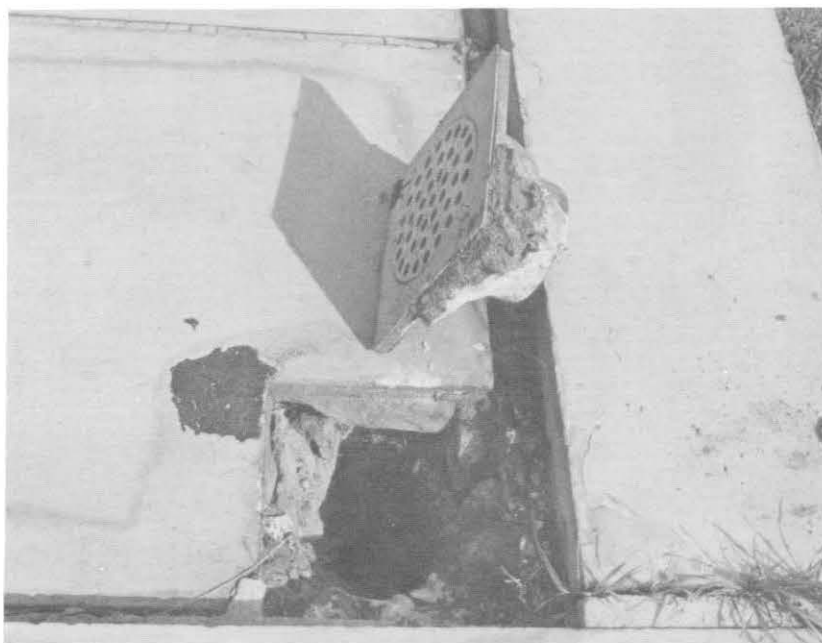
ILLUSTRATION 132. View of drain at corner of planter at south end of upper plaza. Note that drain is not connected to any pipe system. Water simply falls to basement space below upper plaza.
