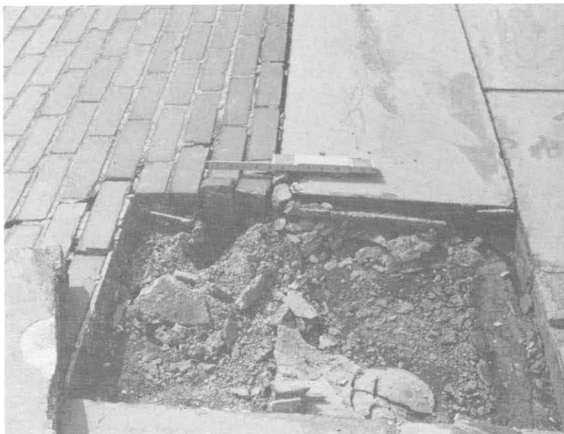
ILLUSTRATION 129. Detail view of condition of concrete fill slab and setting bed below sandstone and brick pavers of upper plaza.
