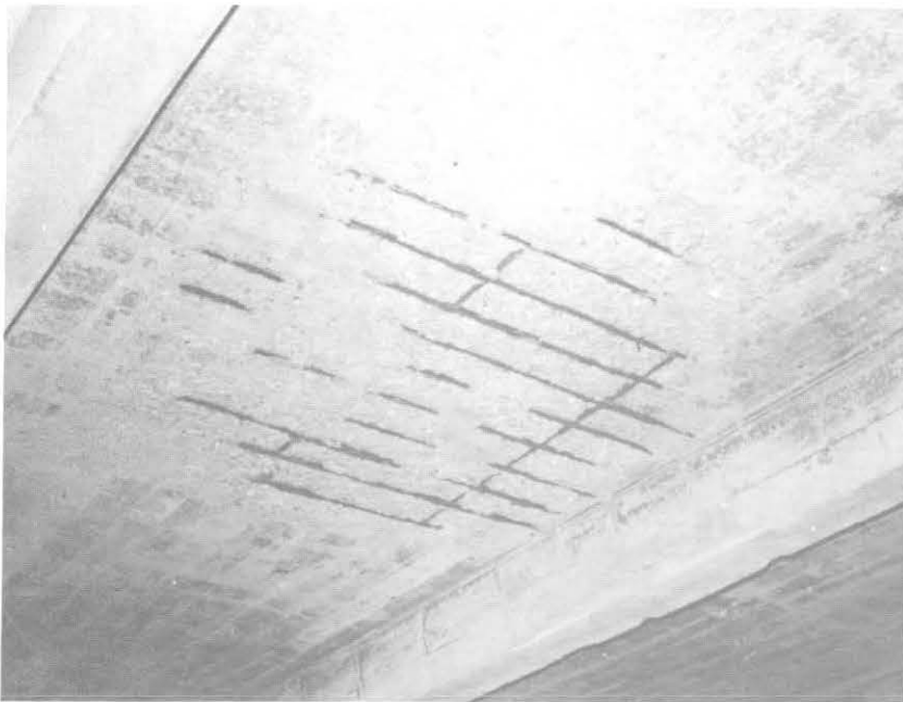
ILLUSTRATION 111. View of underside of upper plaza slab showing rusting condition of steel and spalled concrete.
