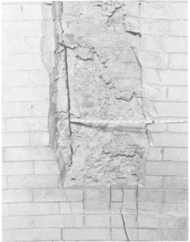
ILLUSTRATION 47. Detail view showing structural concrete with major crack; brick and mortar with wire loop, minimum depth of crack.
