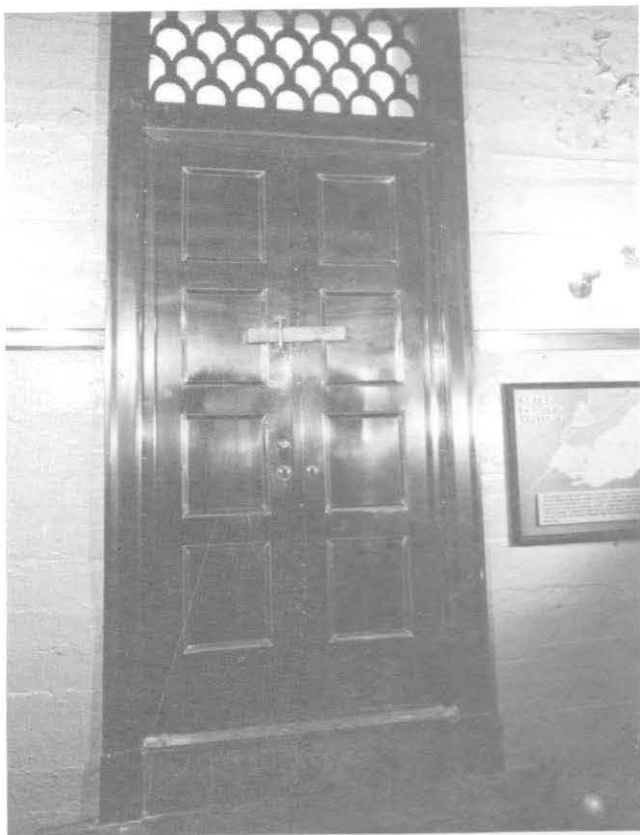
ILLUSTRATION 89. View of bronze door from observation gallery indicating faulty or missing hardware, lack of weather-stripping and dissimilar finish of bronze.
