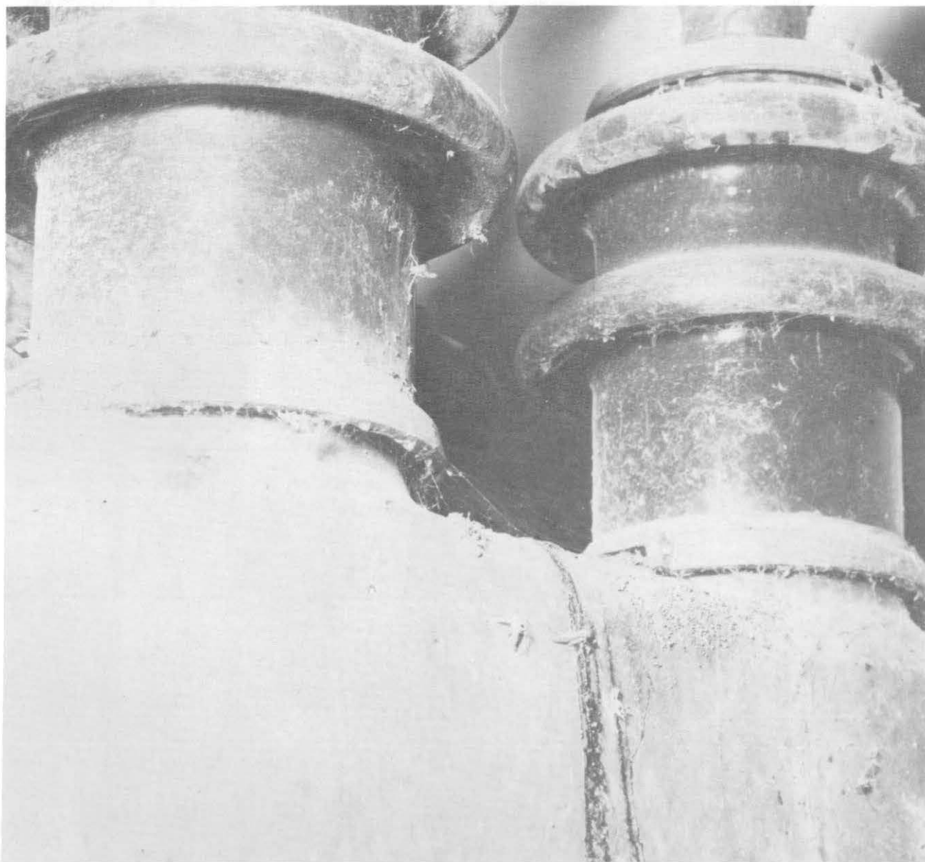
4d. MAIN OIL CIRCUIT BREAKER The extremely dirty bushings should be cleaned, and the connections tightened and insulated.
