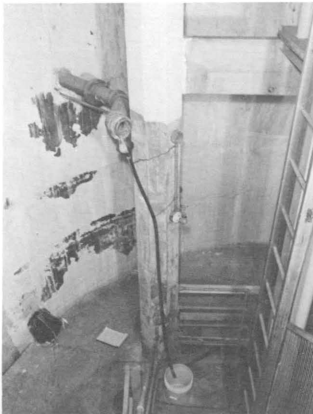
ILLUSTRATION 77. View of interior of penthouse at the southwest column showing pipe from original floor drain of observation gallery. Peeled paint is the result of moisture penetration.
