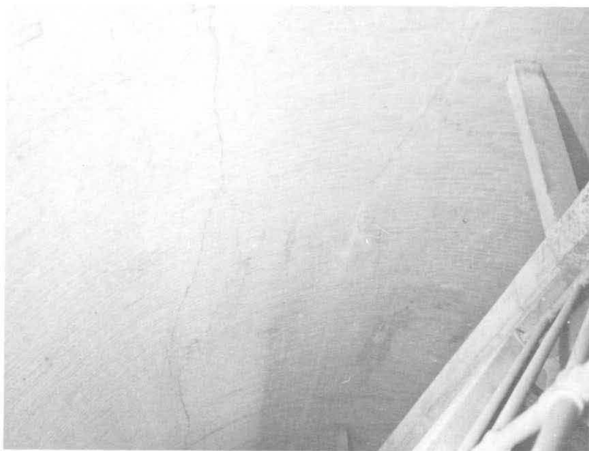
ILLUSTRATION 55. General view of brick crack in north quadrant of column shaft at approximately level 5.
