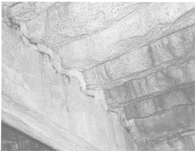
ILLUSTRATION 144. Detail view at underside of granite stair showing sloped and stepped support beam.
