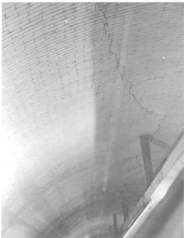
ILLUSTRATION 42. Typical view looking down column shaft showing octagonal column and column bracing into brick wall.
