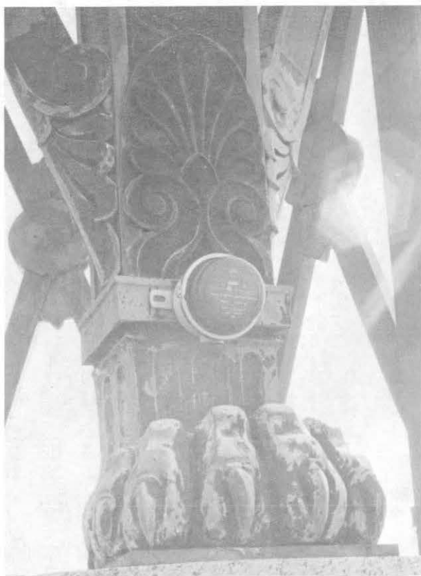
ILLUSTRATION 95. Detail of lion's foot at base of bronze lantern. Round item attached to foot is a photoelectric cell which activates navigational lights.
