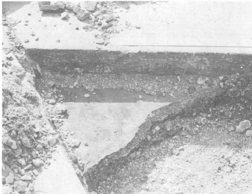
ILLUSTRATION 109. Detail view of sandstone paver, setting bed, fill slab and top of structural concrete slab.
