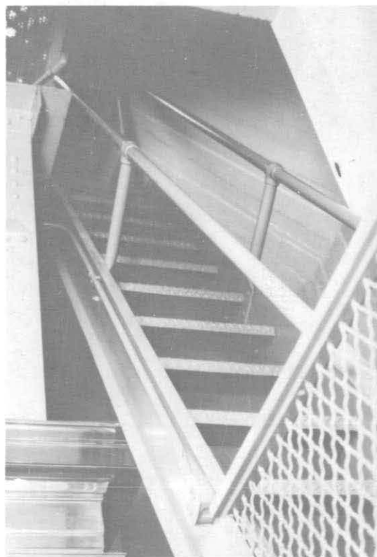
ILLUSTRATION 91. View of ship-ladder stair from upper elevator landing up to elevator machine platform above.
