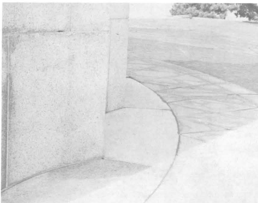
ILLUSTRATION 138. View of oil-type stain in granite paver at east side of column. Cause of stain unknown.
