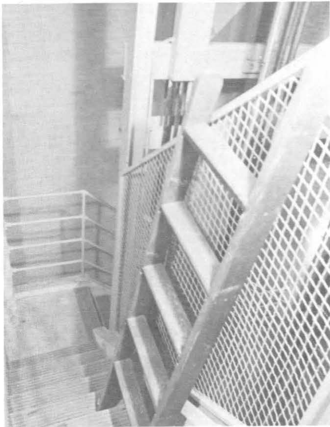
ILLUSTRATION 36. View of typical stair run and platform showing original safety treads. Mesh screen panels separate the stair run from the elevator shaftway.
