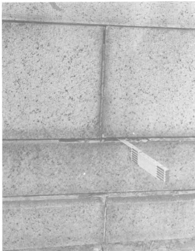
ILLUSTRATION 155. Detail view of typical mortar joints in granite retaining walls indicating poor condition of joints.
