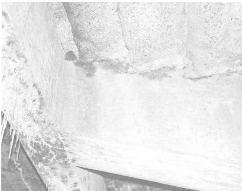
ILLUSTRATION 121. Detail view of granite steps from underside showing stepped beam supports for granite steps.
