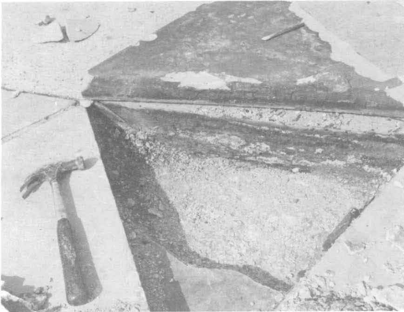
ILLUSTRATION 108. Detail view of edge of granite paver at foot of column. Note lack of waterproofing on the top of the slab.
