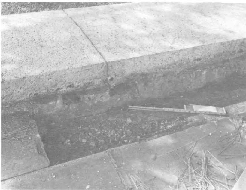
ILLUSTRATION 150. Detail view showing granite curb at the top of a concrete grade beam. Note that the top of the paver is about 2" below its original level, indicated by the line of rough to smooth granite.
