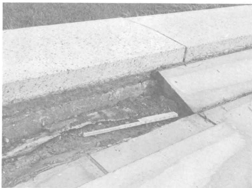
ILLUSTRATION 151. Detail view showing how the sandstone paver edge rests upon rough granite and/or concrete edge of grade beam.
