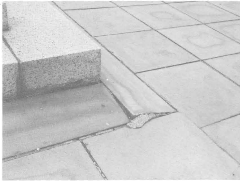
ILLUSTRATION 148. Detail view at east end of granite steps showing inclined pavers due to settling of lower plaza.
