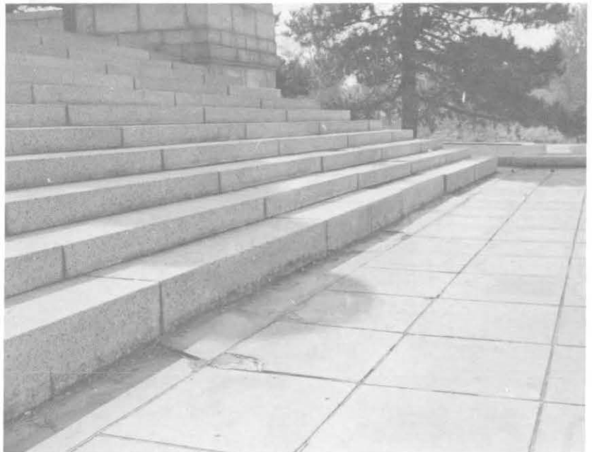
ILLUSTRATION 142. View along lower risers of granite steps looking toward the west. Note settling of lower plaza and misaligned steps.
