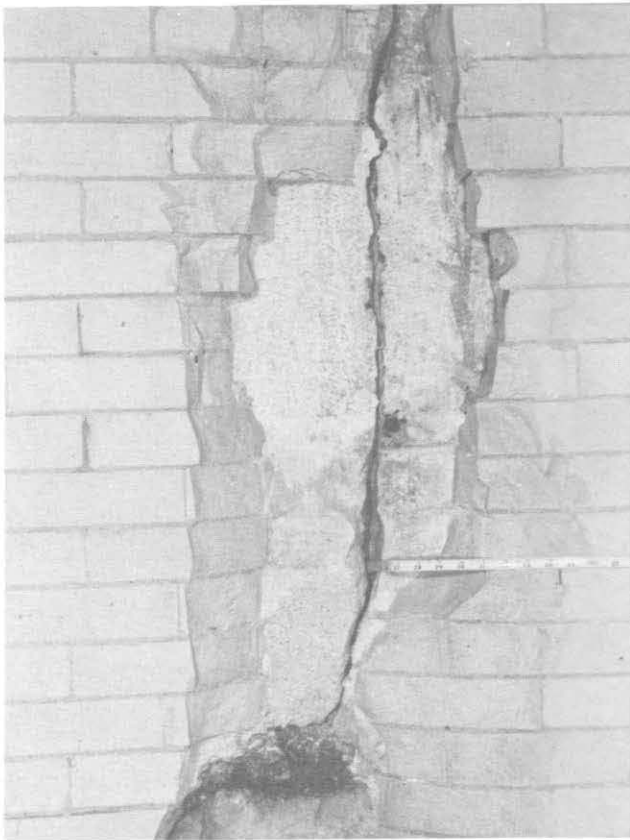
ILLUSTRATION 48. Detail view similar to Illustration 47, above, but also showing chunk of wood embedded in concrete which is an example of foreign matter which may be a cause of brown stains.
