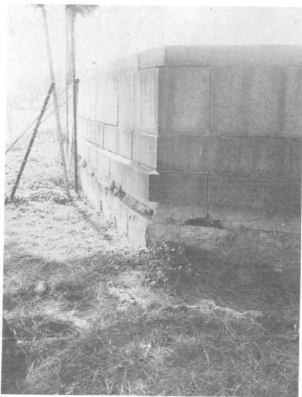
ILLUSTRATION 164. View of southeast corner of retaining wall showing concrete deterioration and lowered grade.
