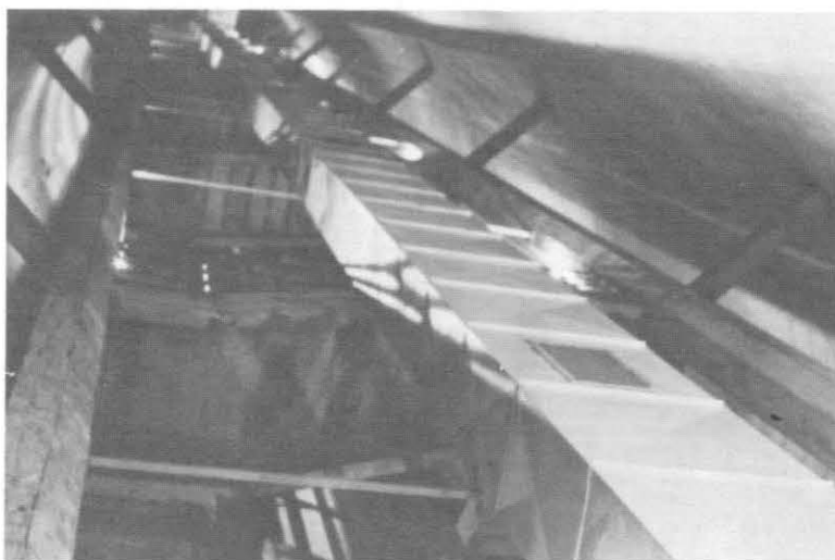
ILLUSTRATION 190. View of the return air duct within the column shaft looking up.
