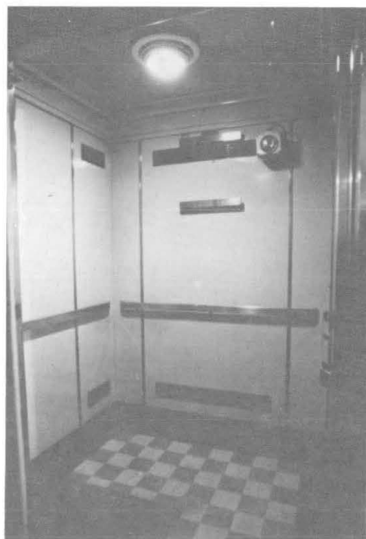
ILLUSTRATION 260. Existing elevator. Note emergency battery lighting unit in rear.
