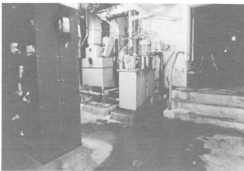
ILLUSTRATION 203. Kathene solution leaking from the tank keeps the floor continually wet.
