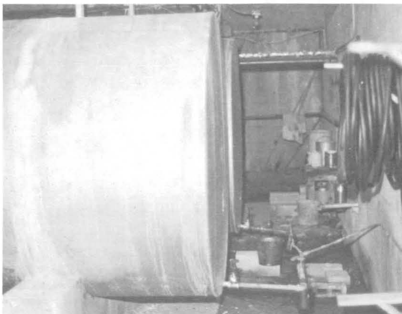
ILLUSTRATION 205. View of the fuel oil storage tanks. Note the pipe stubbed out from the wall immediately below the coiled hose is the discharge pipe from the sump pump in the equipment room located behind this wall.
