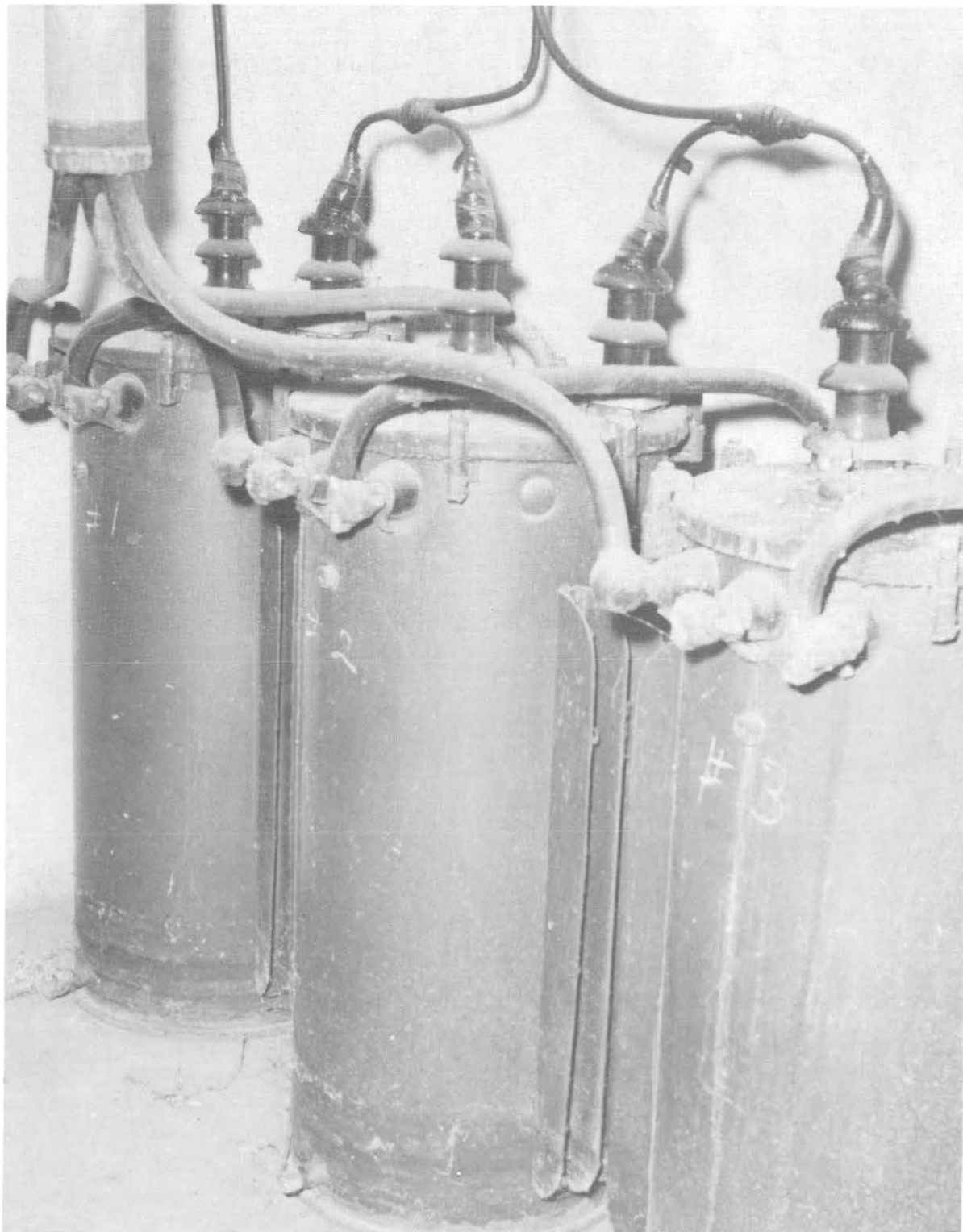
5a. 3-PHASE TRANSFORMER BANK These transformers should be cleaned, rust removed, and painted with a rust resistant transformer paint. The right side transformer tested fair. We recommend a re-test in one year.
