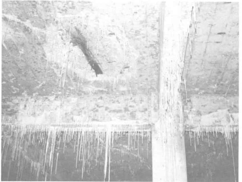
ILLUSTRATION 114. Typical condition of stalactites at underside of upper plaza slab and beams.
