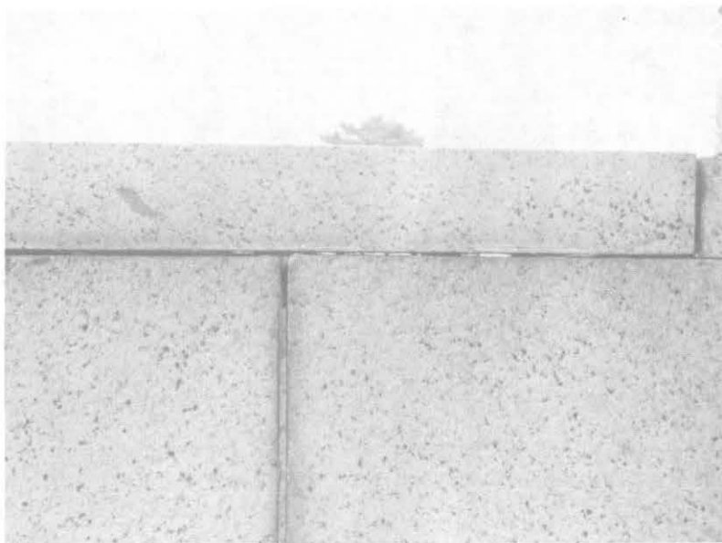
Illustration 156. Detail view of typical mortar joints in retaining walls. Note that daylight may be seen through horizontal joint indicating a lack of mortar.
