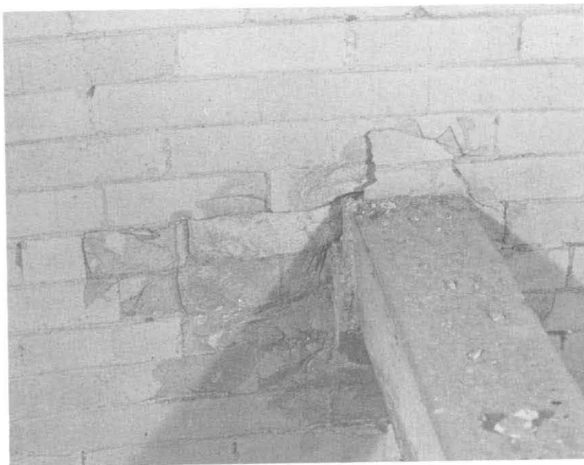
ILLUSTRATION 51. Detail of spalled brick at 6" by 6" concrete column brace and face of brick.
