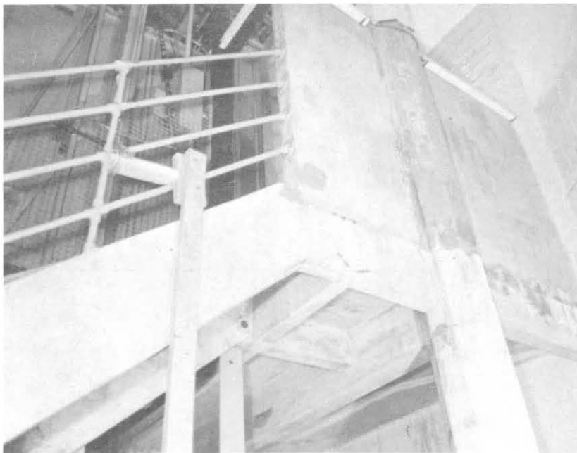
ILLUSTRATION 41. View of underside of upper elevator landing showing typical octagonal column and backside of concrete wall at landing level.
