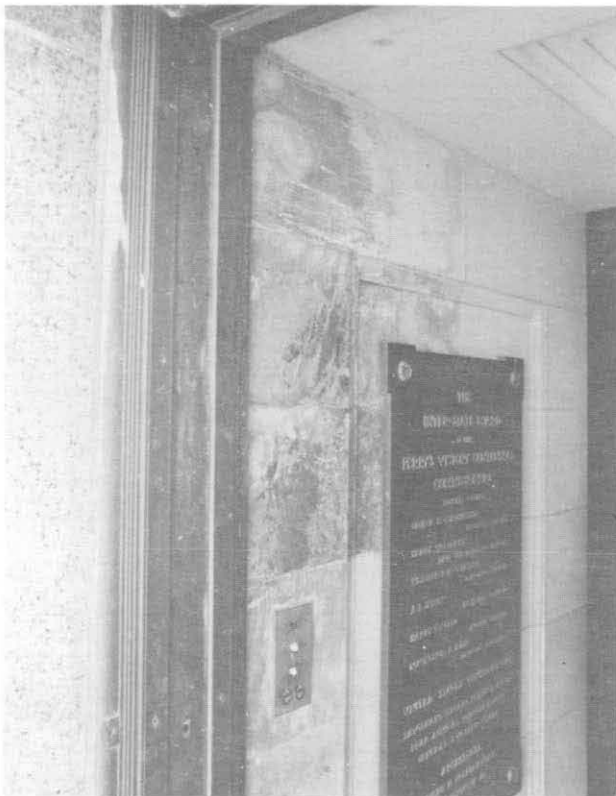
ILLUSTRATION 181. Detail view of north door frame showing corrosion and missing frame screws.
