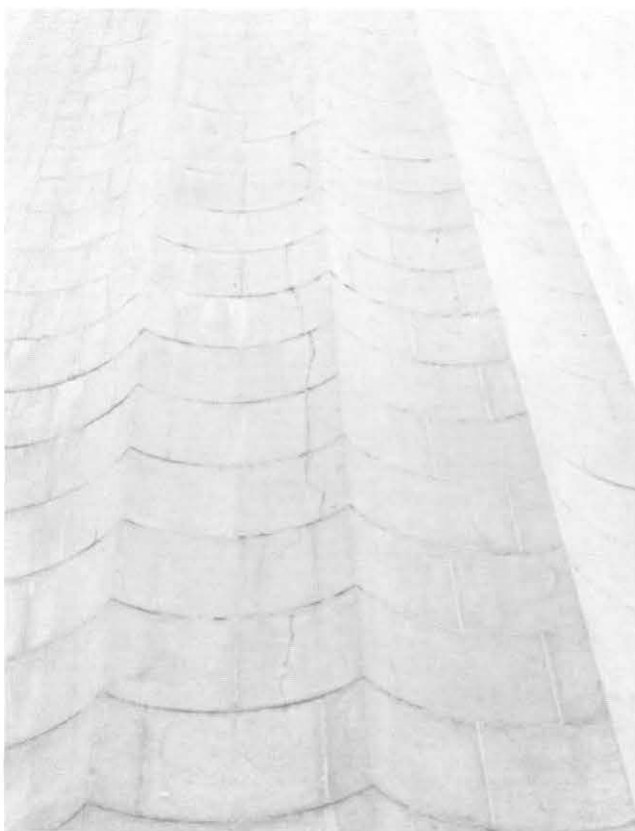
ILLUSTRATION 31. Overview of lower part of southwest side of column showing extent of major crack at flute M, courses 10 through 23.
