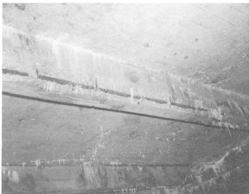
ILLUSTRATION 128. View of a typical beam after rust has caused concrete to spall.
