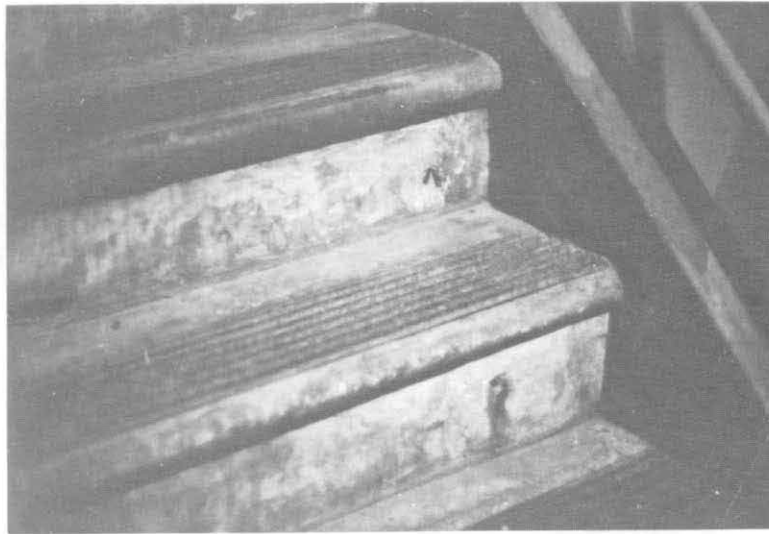
ILLUSTRATION 38. View of stair tread and riser showing the typical existing safety tread with round nosing in good condition.
