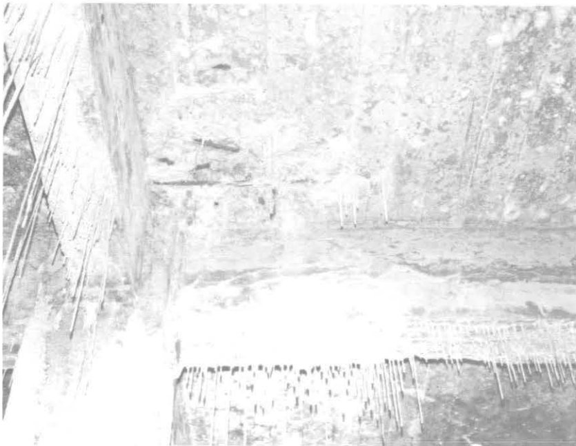
ILLUSTRATION 115. Detail view of typical beams to column intersection showing stalactites at various stages of formation.
