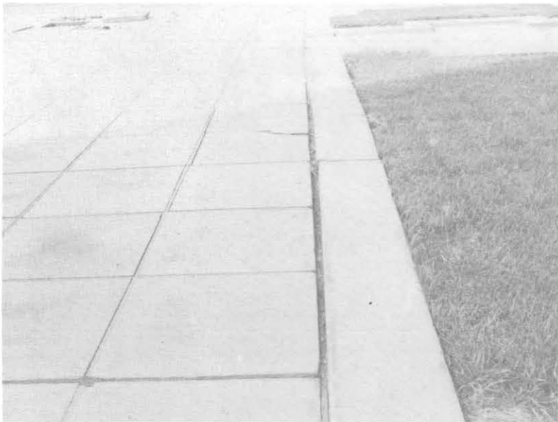
ILLUSTRATION 170. General view of upperside of a typical planting box. Note poor joints between sandstone pavers and sandstone curbstones. See Illustration 171 for section through planting box and recommended waterproofing.
