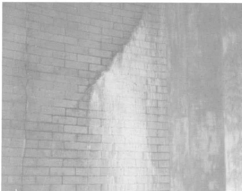
ILLUSTRATION 50. Detail of a major efflorescent stain, located in west quadrant at level 3.
