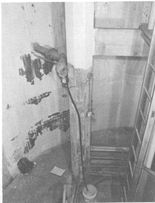
ILLUSTRATION 216. View of interior rainwater conductor serving the observation deck. The floor drain on the deck has been reworked for a free fall to the outside. However, during heavy rains, water will flow from this pipe into the bucket.
