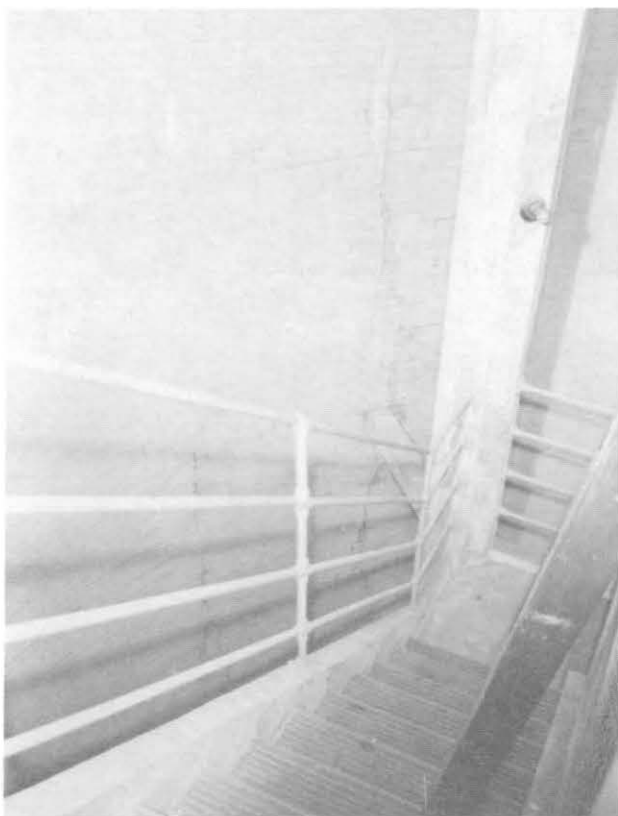
ILLUSTRATION 43. Typical view of stair run showing handrails and original lighting fixture for general illumination of shaft interior.
