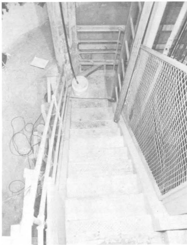
ILLUSTRATION 37. View of uppermost stair run and platform showing replacement safety tread and treads with cement wash only.
