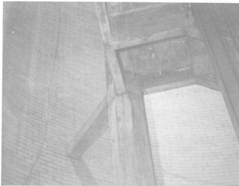
ILLUSTRATION 56. General view of brick crack in north quadrant of column shaft at approximately level 7.
