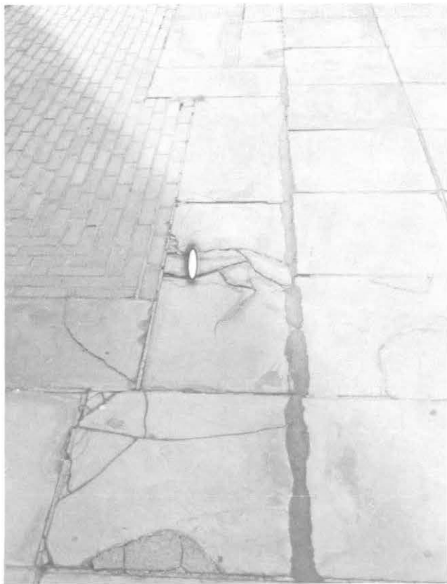
ILLUSTRATION 130. General view at northeast quadrant of upper plaza showing deteriorated joints, cracked and spalled sandstone pavers and brick paving inlay pattern.
