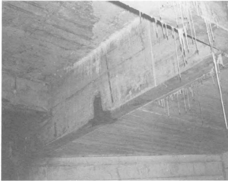
ILLUSTRATION 169. General view of underside of a planting box slab which is typically in the same plane as the bottom of the beam. Note that no drains were evident. Dark stain is probably seepage through bottom of box.
