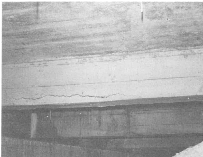
ILLUSTRATION 127. View of a typical beam with crack formed by rusting steel bars behind.
