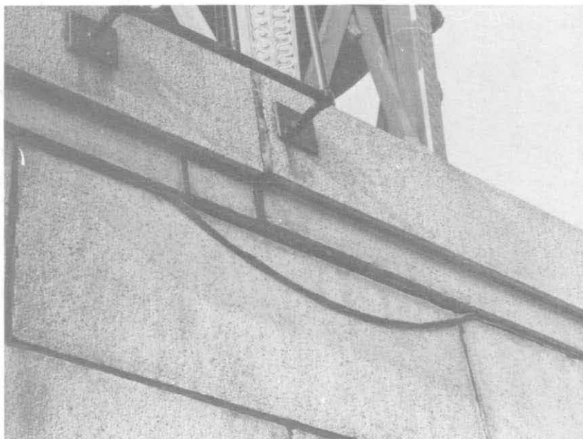
ILLUSTRATION 78. Detail at cornice of penthouse indicating sealant failure. Pipe railings were added with navigational lights at later date.
