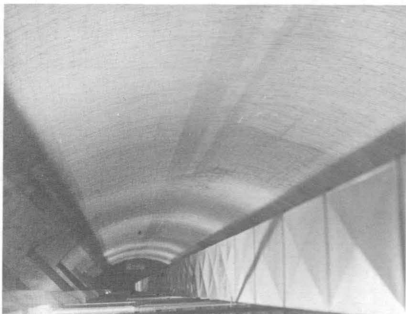
ILLUSTRATION 189. View of supply air duct within the column shaft. Photo taken from an upper level looking down.
