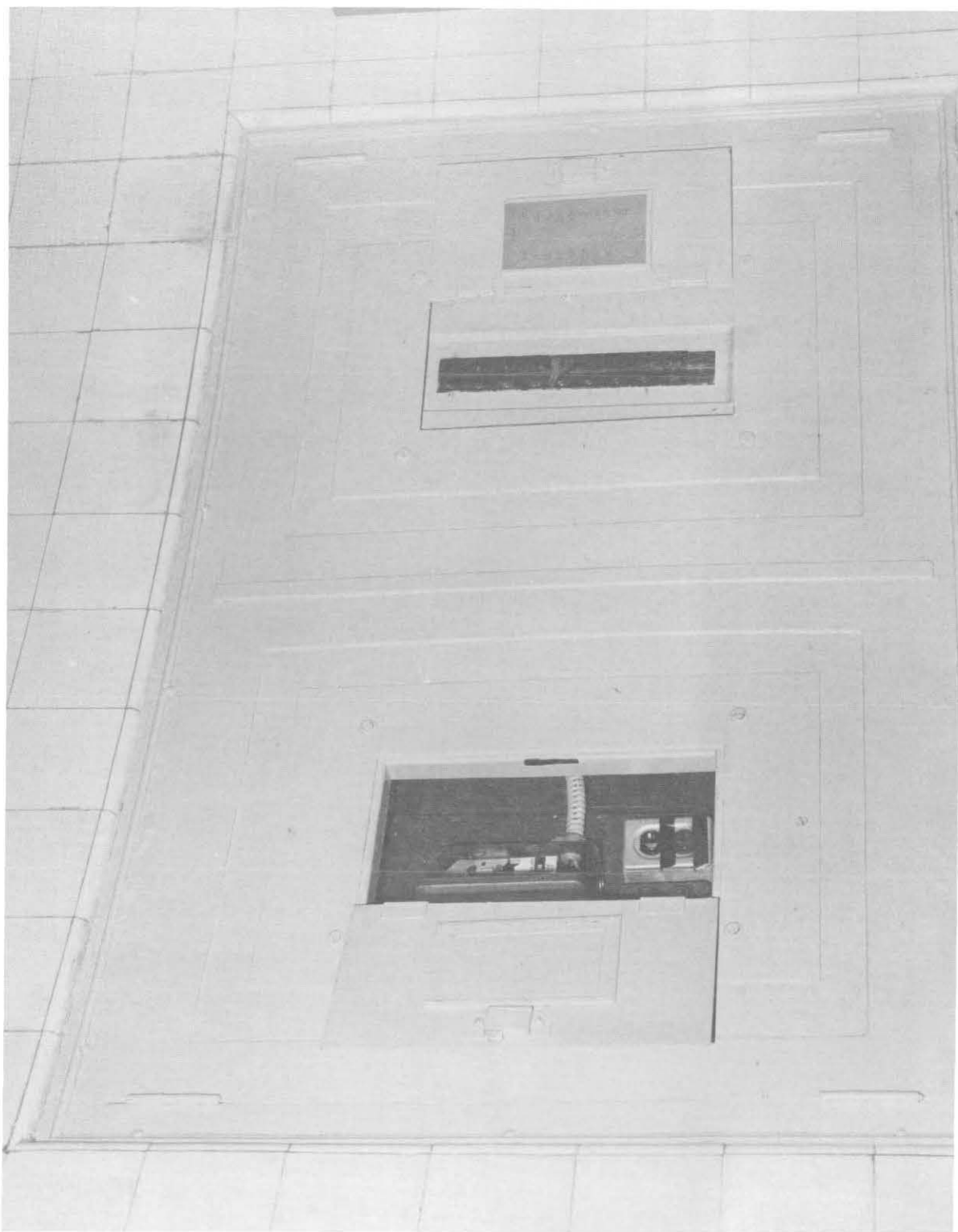
11. LIGHTING PANELBOARD This lighting panelboard is adequate for its present use. Possible future parts replacement problems may suggest the installation of a new panelboard during any present electrical modernization program.
