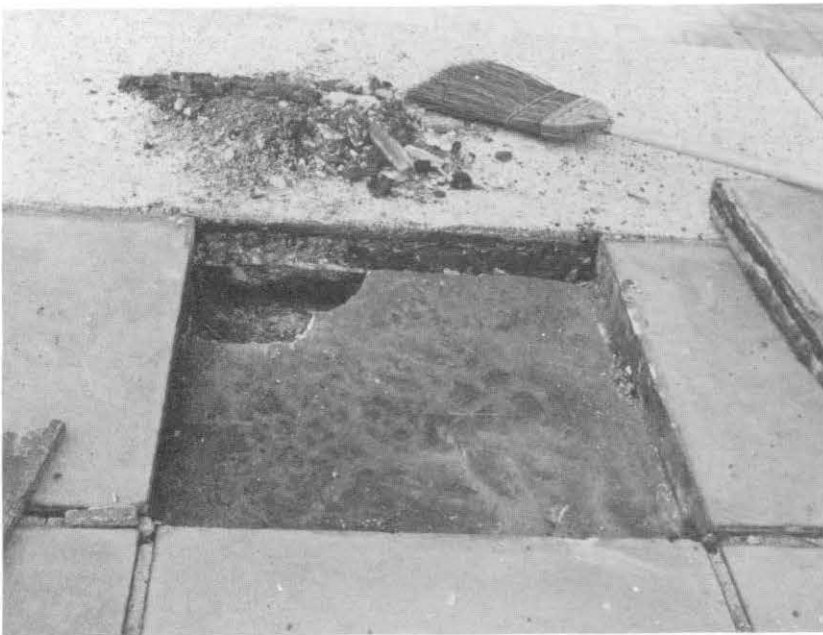
ILLUSTRATION 140. Detail view of top tread of granite steps at upper plaza and typical setting bed condition under sandstone paver.
