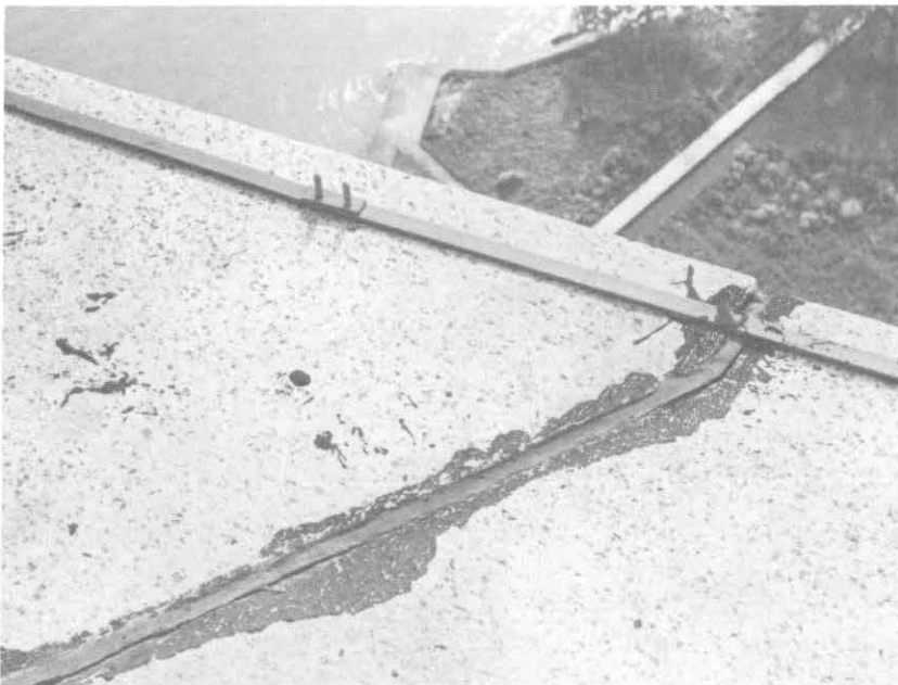
ILLUSTRATION 85. Detail of typical joint indicating improper removal of previous sealant prior to installation of new sealant. Metal bar is part of the lightning grounding system.
