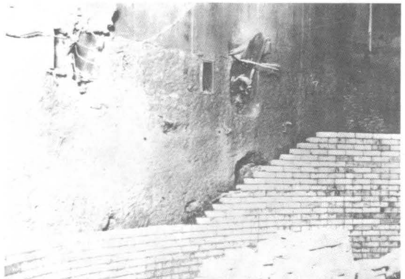
ILLUSTRATION 11. Scars remaining on the inner surface of concrete walling the column well from placing and removing the derrick support system, and partially set brick veneer for the interior finish of the column interior.
