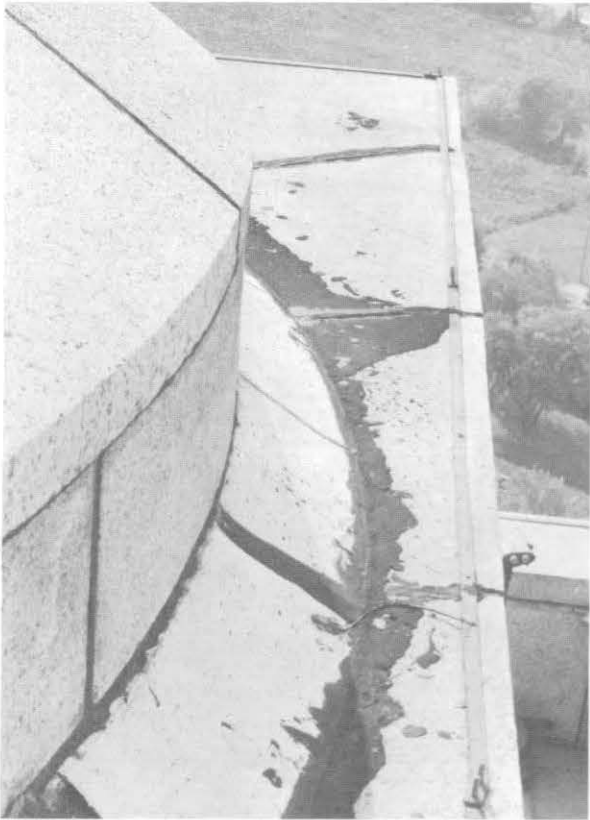
ILLUSTRATION 246. Typical lightning bus at elevator penthouse.
