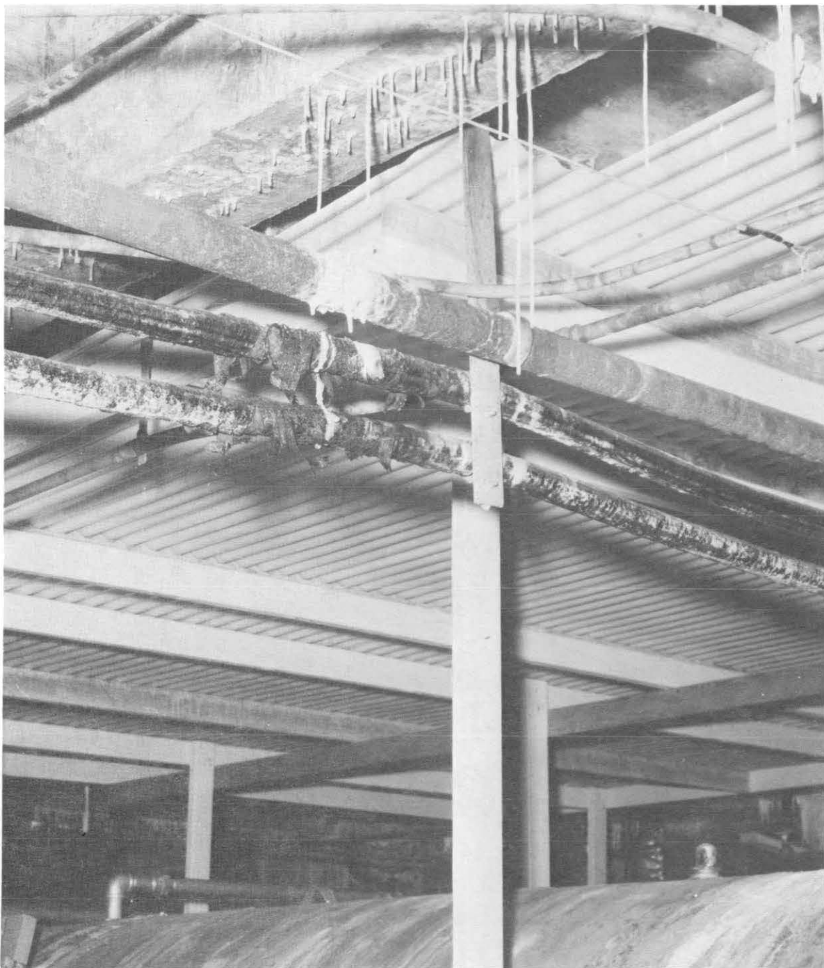
9a. BASEMENT CABLE The cables for floodlighting, elevator, and interior lighting are inadequately supported and exposed to damage and high stress concentrations at the support point. A cable tray and conduit system should be installed to continuously support these circuits. As an alternative, a stress spreading support plate should be installed at all attachment points. The outer jacket should be repaired with vinyl type tapes where the severe jacket damage and rotting are noted.
