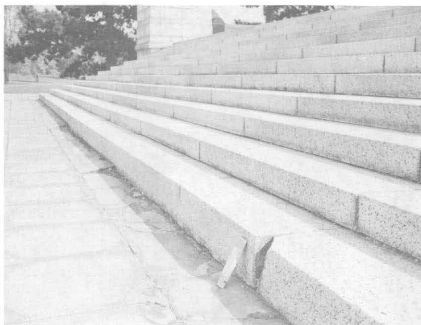
ILLUSTRATION 143. View along lower risers of granite steps looking toward the east. Note chipped stone and poor joints.
