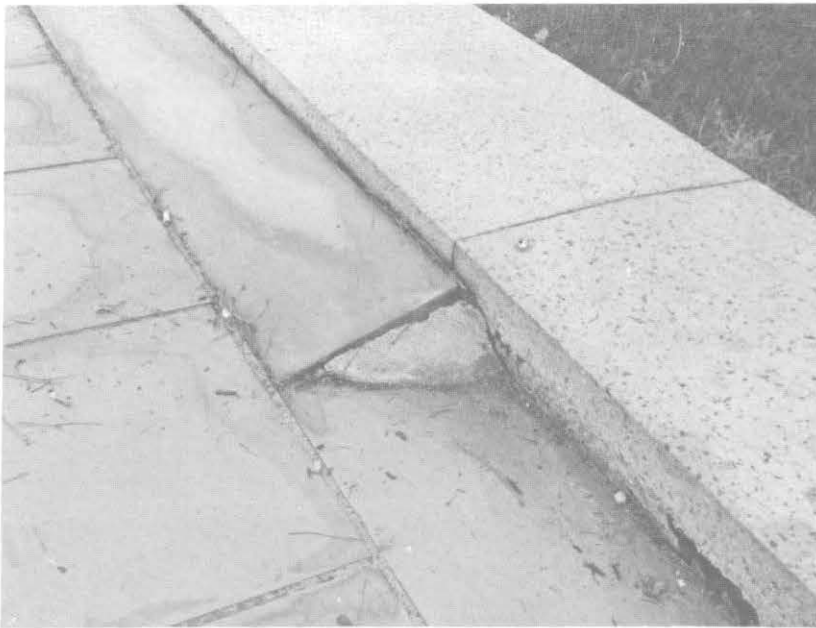
ILLUSTRATION 149. Detail view at east edge of lower plaza showing inclined pavers and flat pavers. Note rough cut of bottom edge of curbstone.
