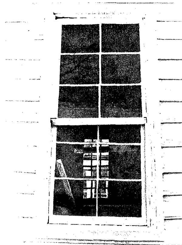
Illustration 79 Outside west elevation, north window
