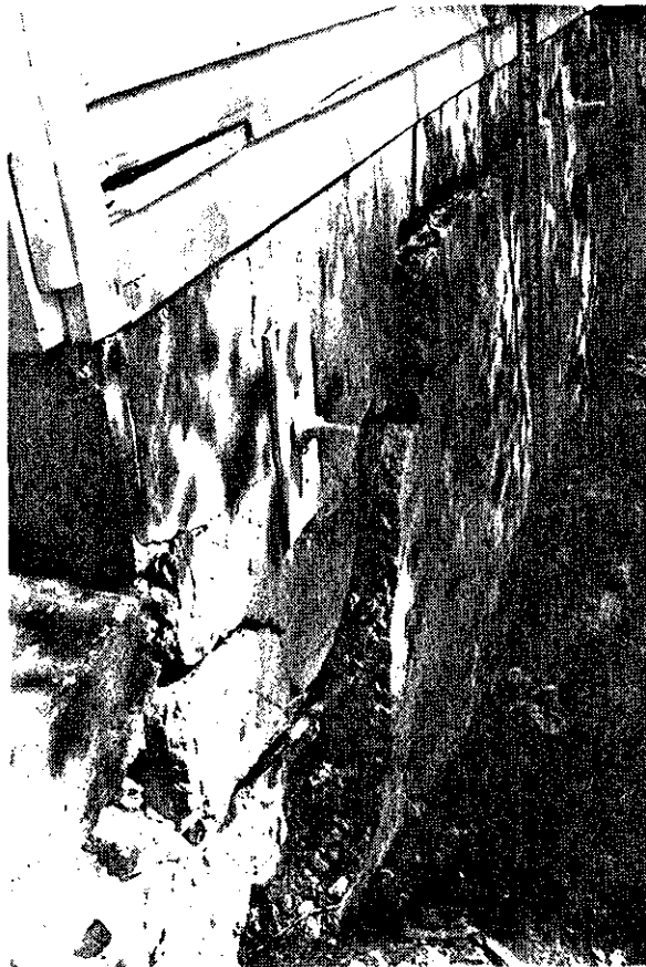
Illustration 92 Carriage House West elevation Foundation failure
