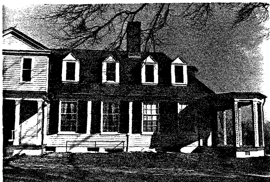
Illustration 39 Manor House South elevation (partial) East end
