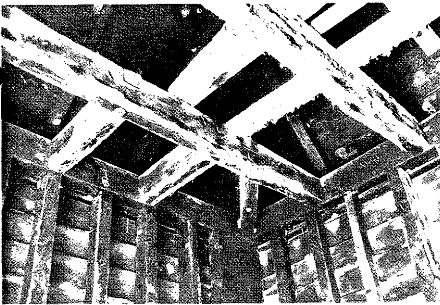
Illustration 112 Smokehouse Interior, framing Northwest corner
