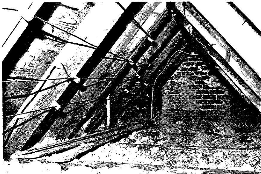
Illustration 70 Manor House Interior, above Room 213 from south
