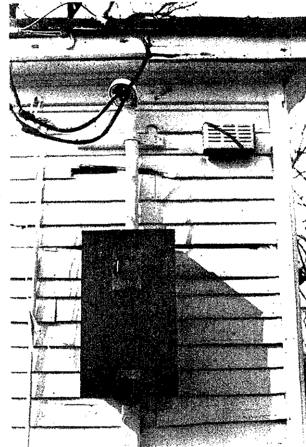
Illustration 93 Carriage House East elevation Damaged weatherboarding
