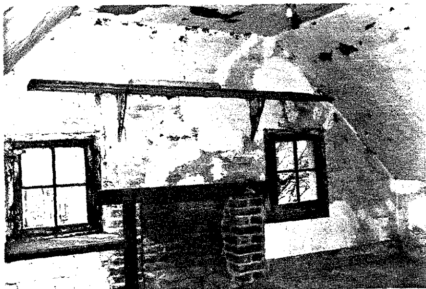
Illustration 83 Outside kitchen Interior, second floor North fireplace
