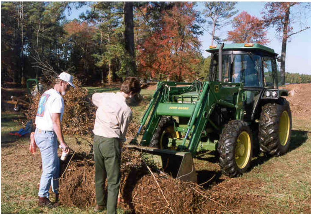
Removal of duff is easily handled at this point by a front-end loader. (Fort Wadsworth, 10/1994)
