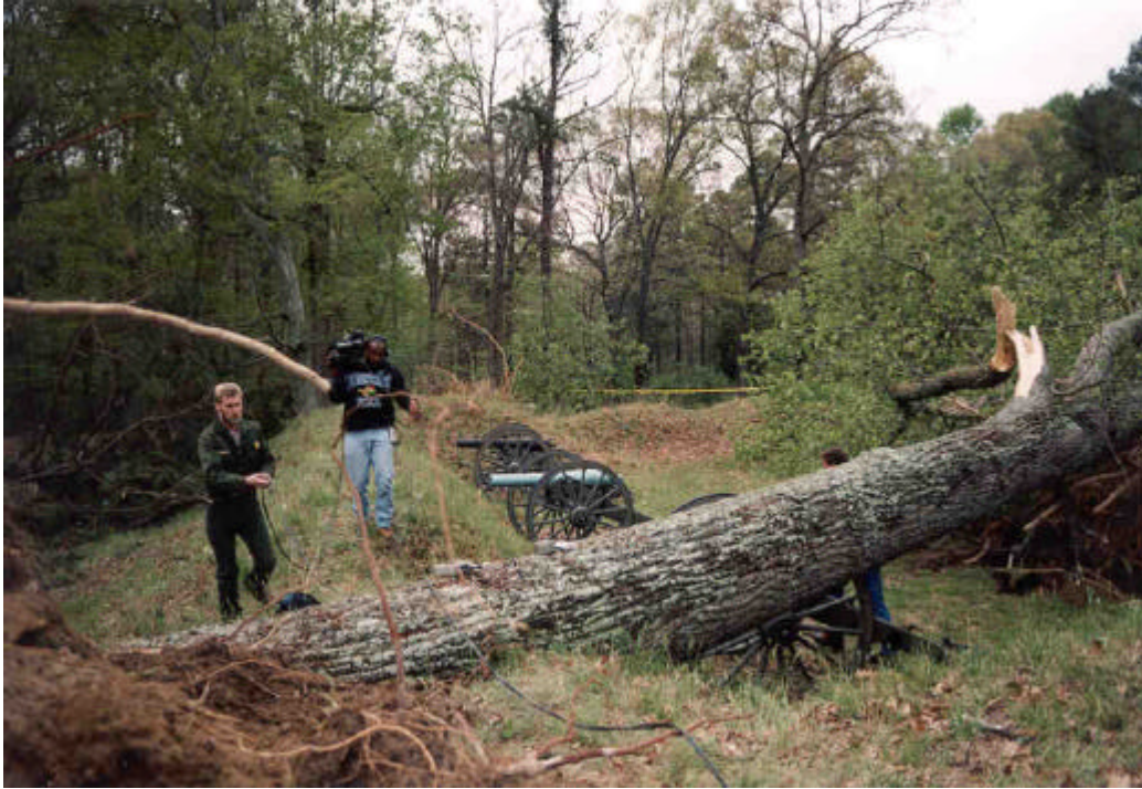
Uprooted trees also damage earthworks by crushing parapets upon impact. (Wind Damage at Battery XIII, 4/1998)
