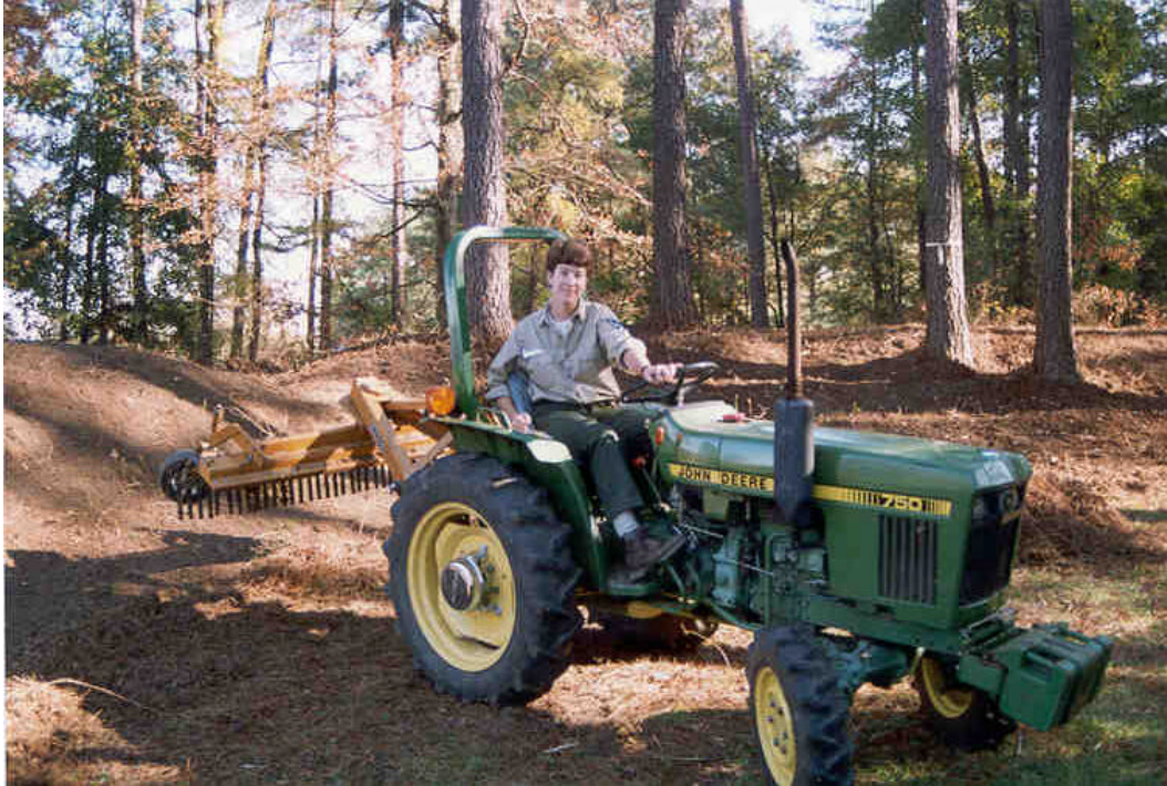
Once the duff is off the earthworks, mechanical means can be employed for raking into piles. (Fort Wadsworth, 10/1994)
