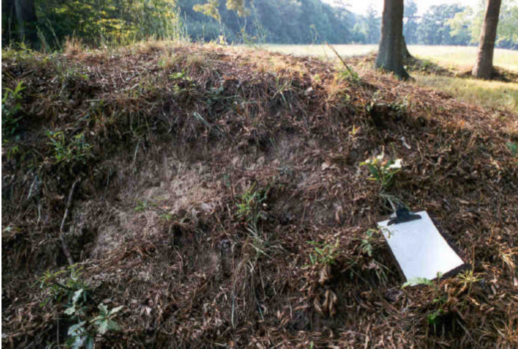
Steep slopes prevent leaf or forest litter from providing an adequate cover to prevent erosion (Battery XI, 7/1997)
