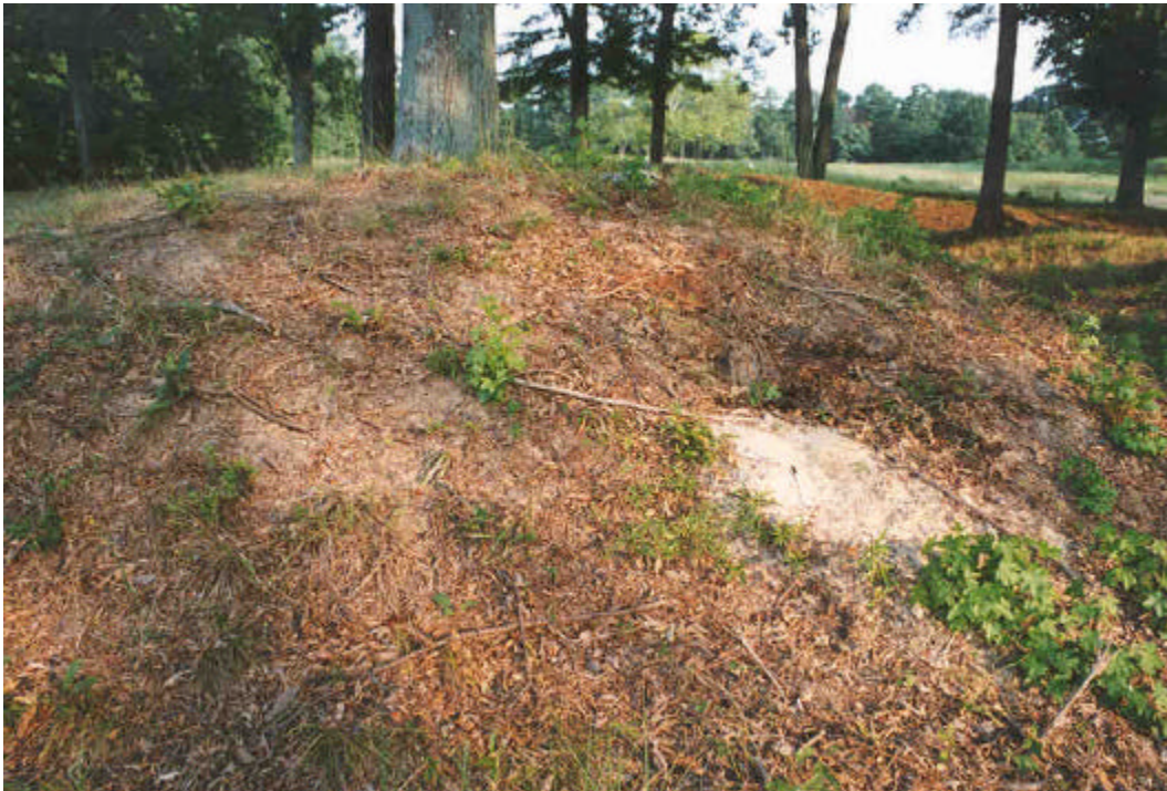
Groundhogs often burrow into earthworks and create additional erosion impacts. (Battery XI, 7/1997)
