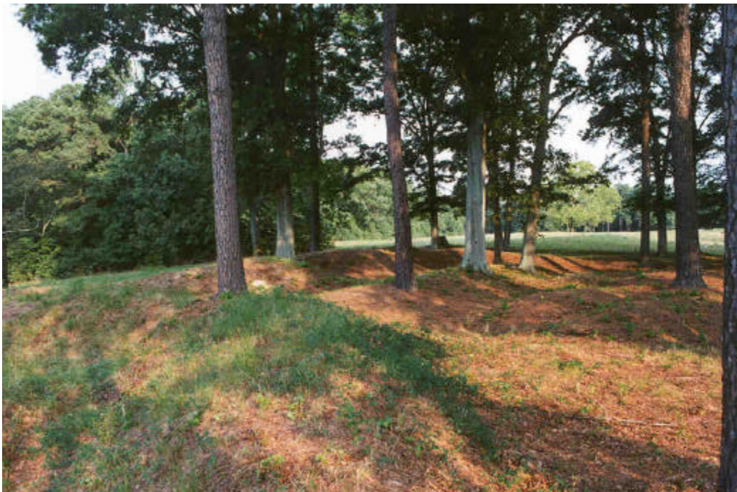
Limited ground vegetation, partially due to insufficient sunlight, does not provide adequate erosion protection. (Battery XI, 8/1997)
