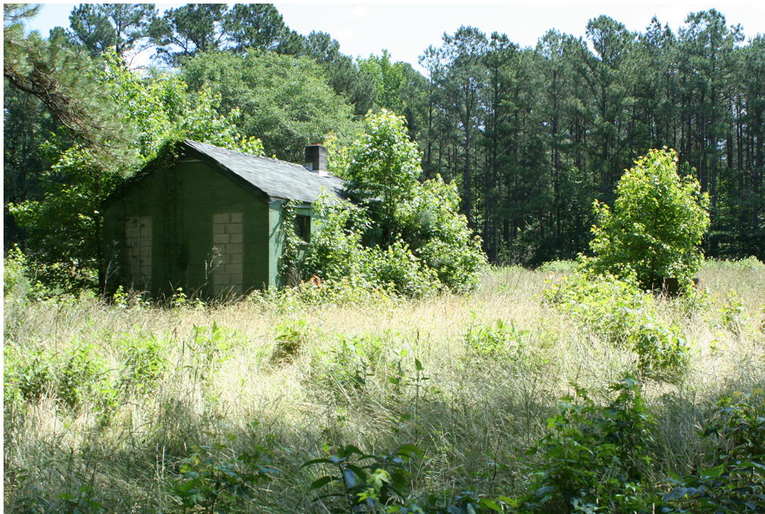
Figure 27. Pump House Tack Room, looking north. (OCLP, 2021)
