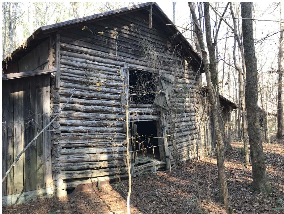
Figure 28. The barn structure associated with the unknown farm complex located off of White Oak Road. Despite a partial collapse, it is the largest of the six buildings at this site. (OCLP 2019, IMG-0653)
