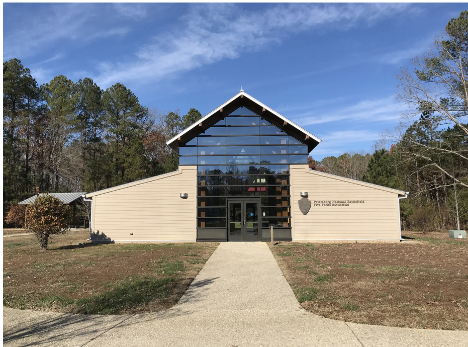
Figure 24. The Five Forks Visitor Contact Station, completed in 2009. (OCLP 2019, IMG-0710)
