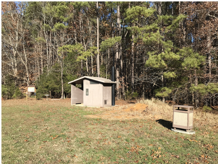
Figure 29. View of the comfort station at the end of the Access Loop Road. (OCLP 2019, IMG-0636)
