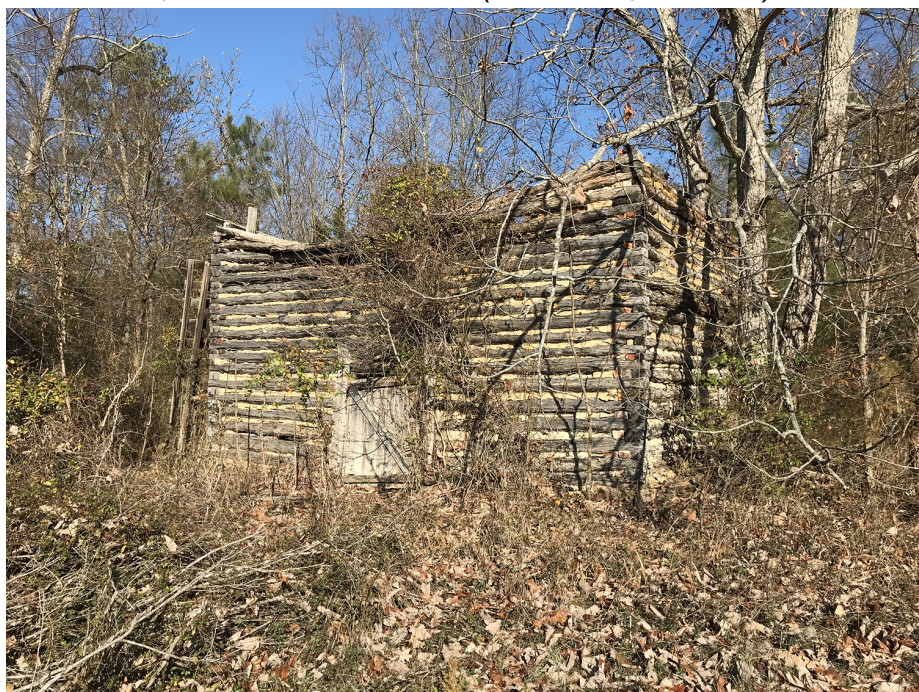
Figure 27. The Five Forks Tobacco Shed is located within a small tree stand just south of the Five Forks intersection. Much of the roof has been stolen, and the park plans to remove the non-historic structure. (OCLP 2019, IMG-0637)
