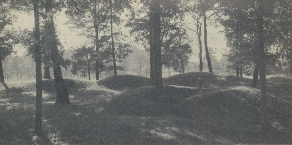
Earthworks at Fort Stedman.
