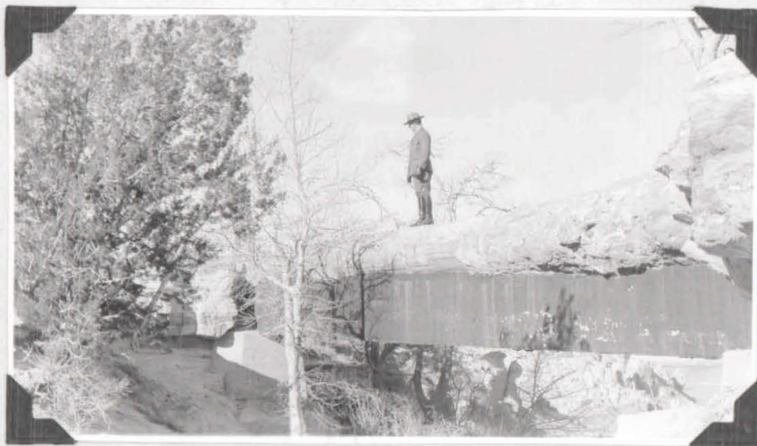
Figure 8. Park Naturalist Walker standing on Agate Bridge, formed of petrified log and reinforced with concrete.
