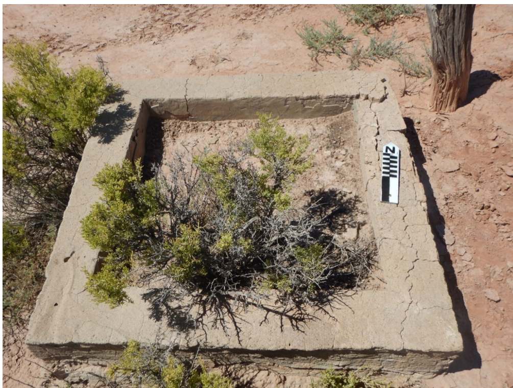
FIGURE 2. Poured concrete stock tank or 'drinker' (Feature 2).
