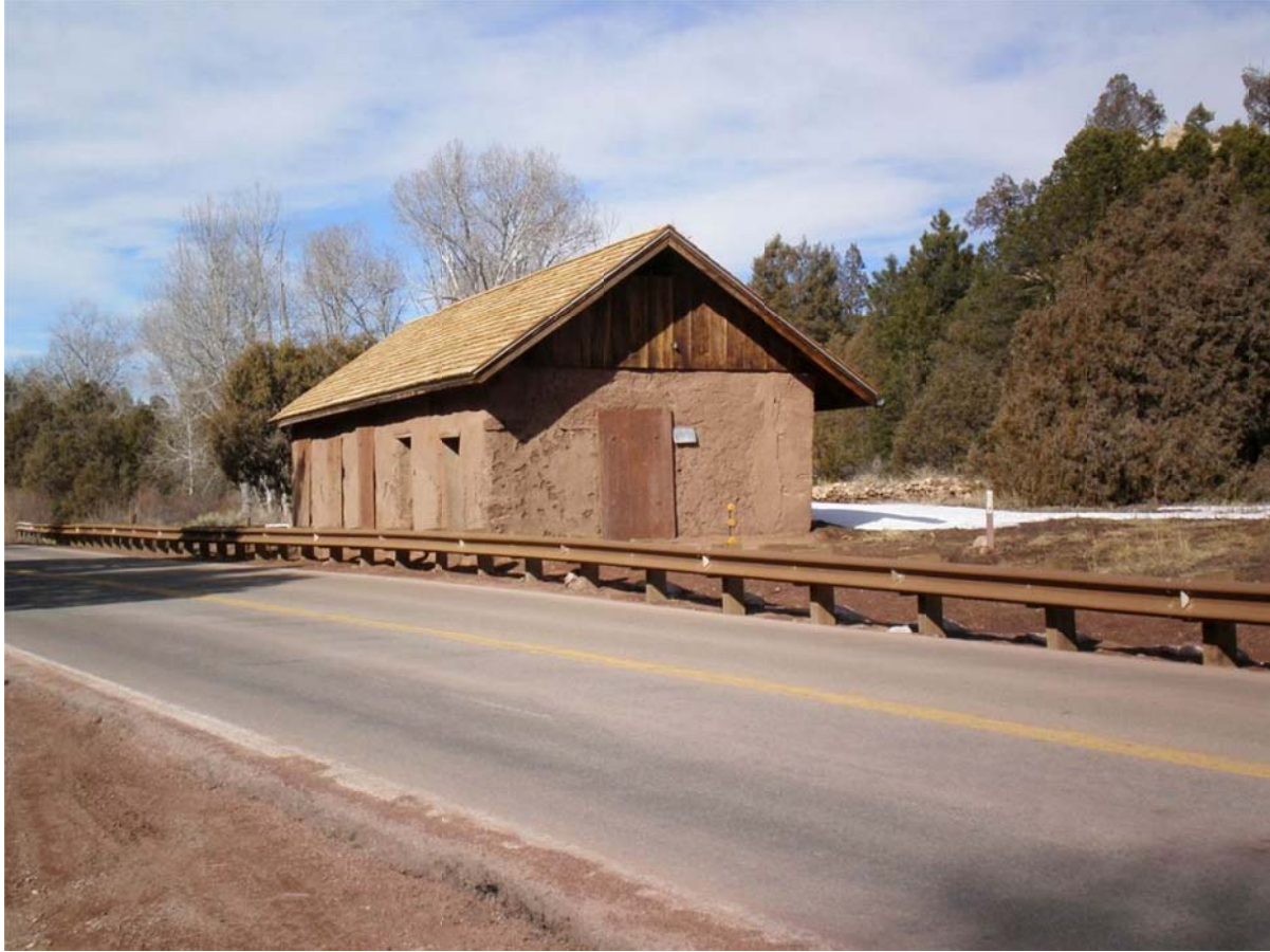
This adobe building is the last standing structure of Pigeon's Ranch, which served as a hostelry on the Santa Fe Trail and also figured prominently in the Civil War Battle of Glorieta Pass. Photo by Cori Knudten.
