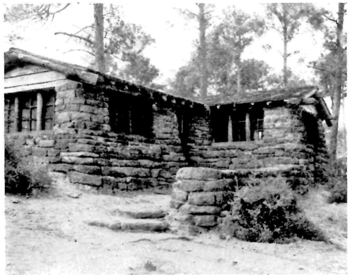
Cabin B, Bastrop State Park, Texas
