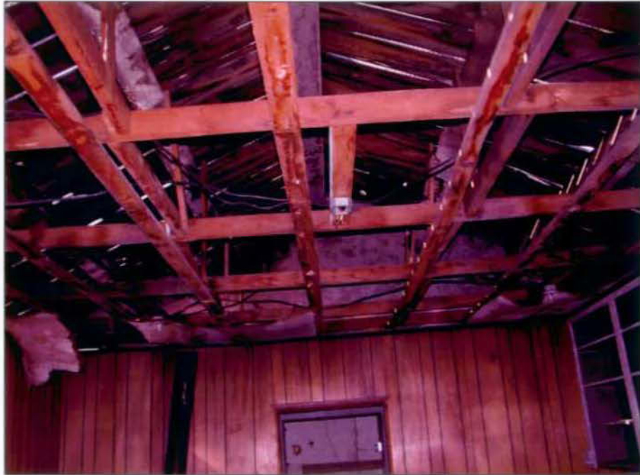
Detail of center room (room 2) roof/ceiling structure, looking south.
