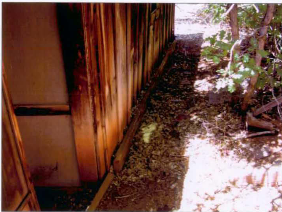
Detail of north wall. Note sedimentation, and protection boards at base of wall.
