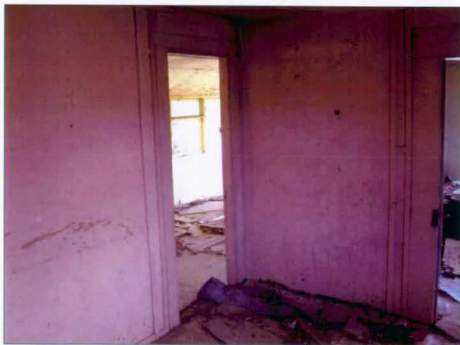
Interior of room 1, looking northeast towards room 3.
