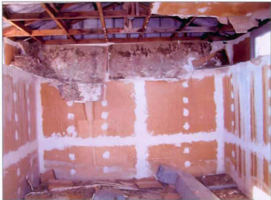
Detail of interior. Note gypsum board walls on furring, and trussed/framed roof structure.
