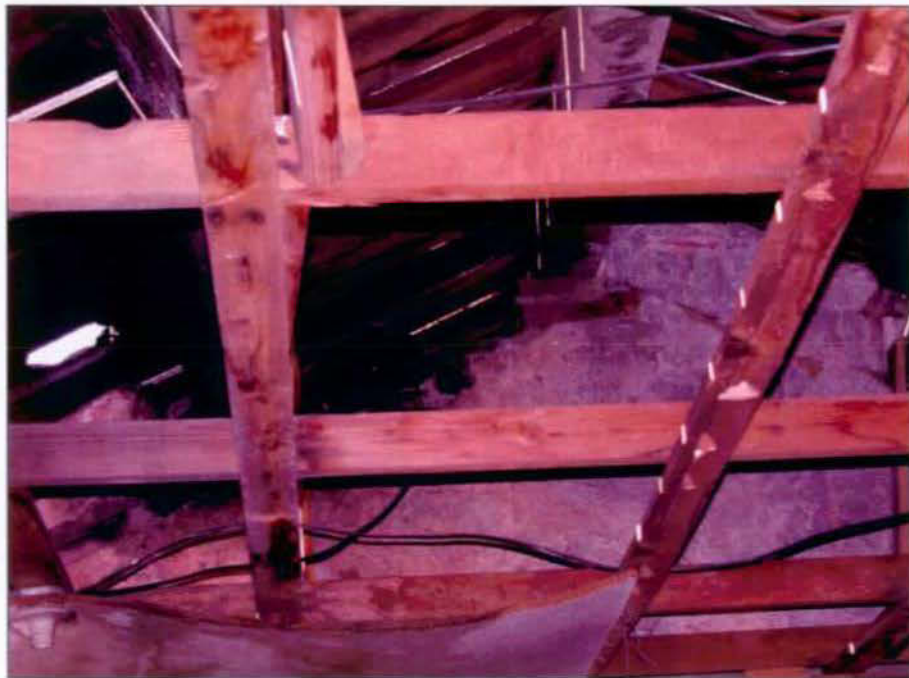
Detail of interior gable wall and roof/ceiling structure in center room (room 2), looking south.
