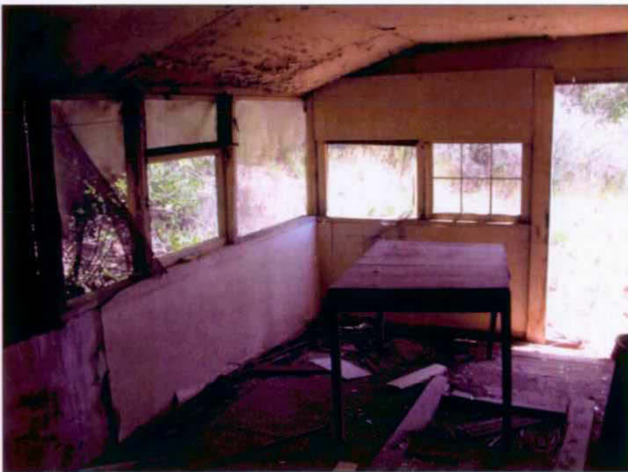
Interior of room 3, looking east.
