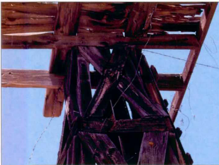
Detail of underside of platform near top of windmill.
