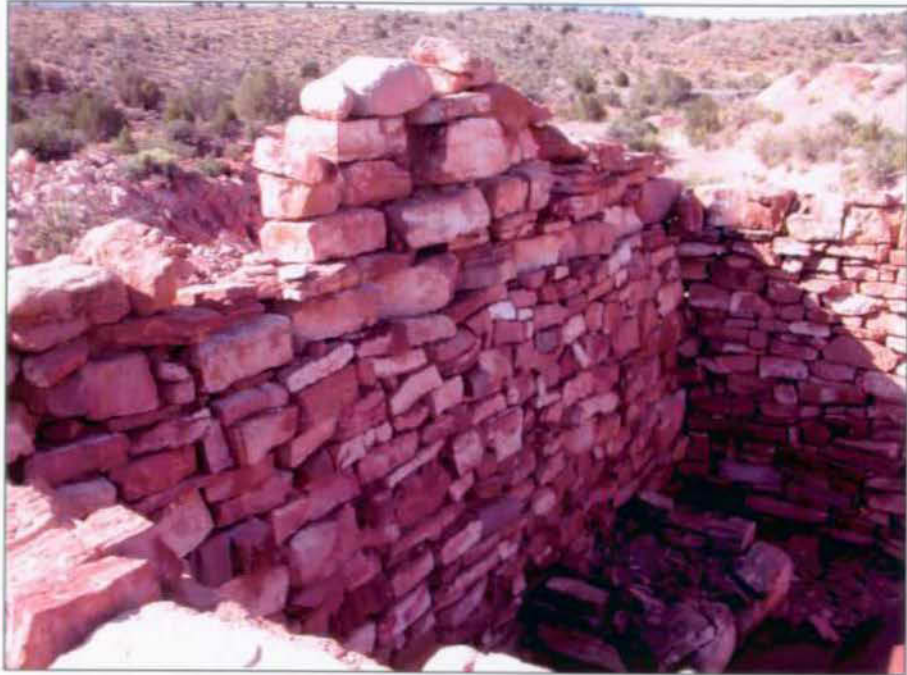
View of interior of east wall. Note header/bond course which runs at eave height.
