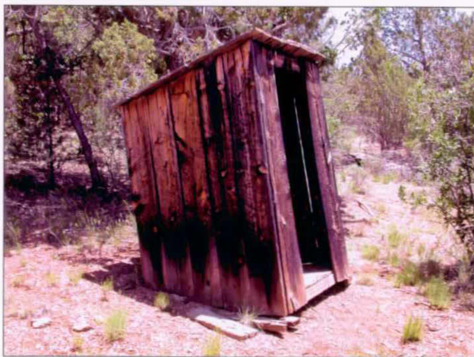
View from southwest. Note how structure is settling.
