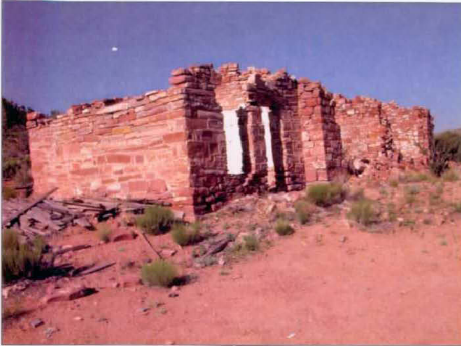
View from northeast, addition in foreground.
