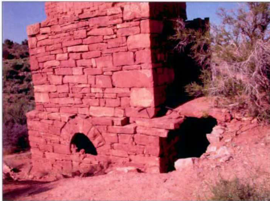
Detail of west elevation.
