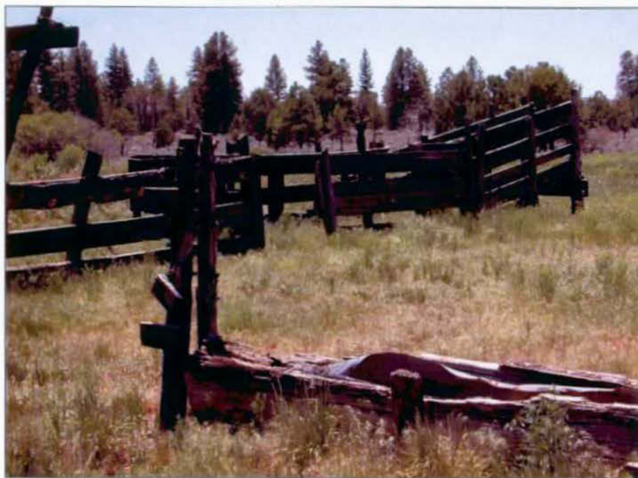
Loading ramp from west.
