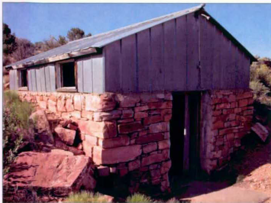
View from northeast. Note metal clad addition on top of stone walls.
