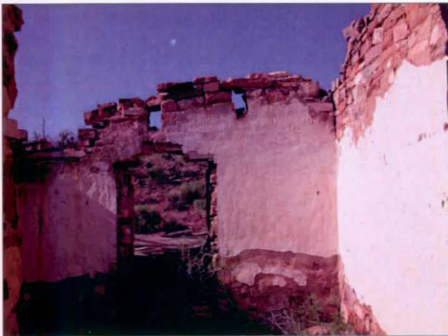
Interior of addition. Note plaster on walls, and beam pockets in south wall.
