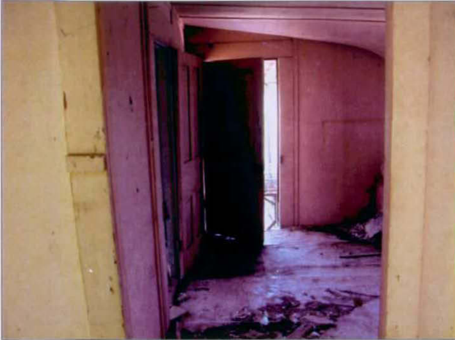
Interior of room 1, looking south from room 3.
