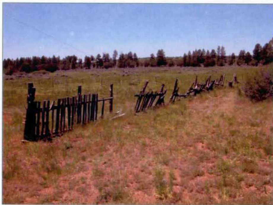
West portion of picket fence from northeast.
