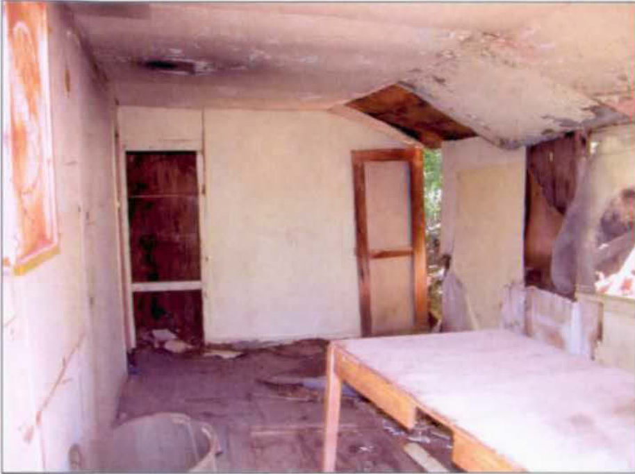
Interior of room 3, looking west
