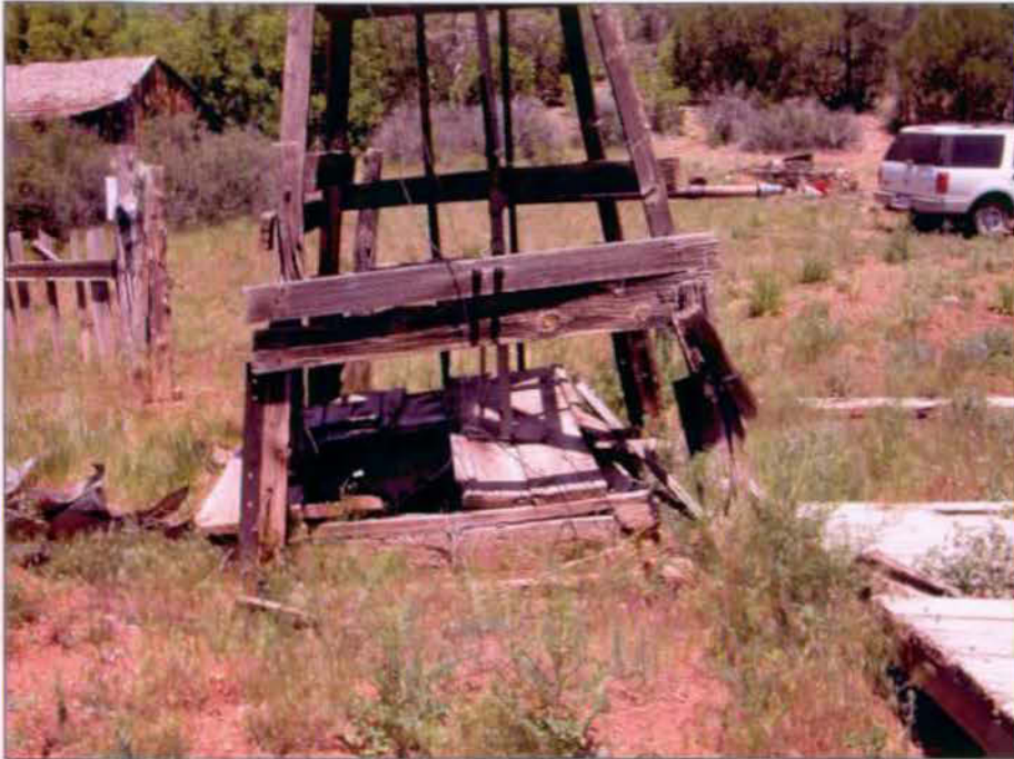
Detail of base of structure. Note well below.
