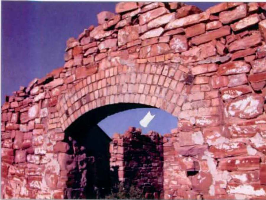
Detail of arch in wall between room 1 and room 2 (from room 2).
