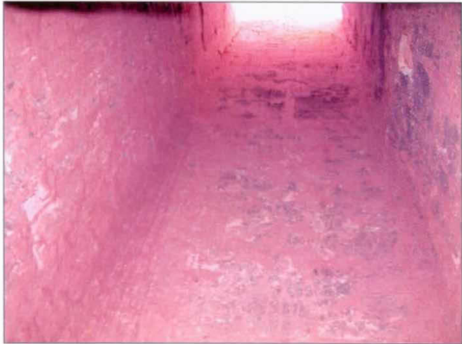
Looking up the chimney from platform on north.
