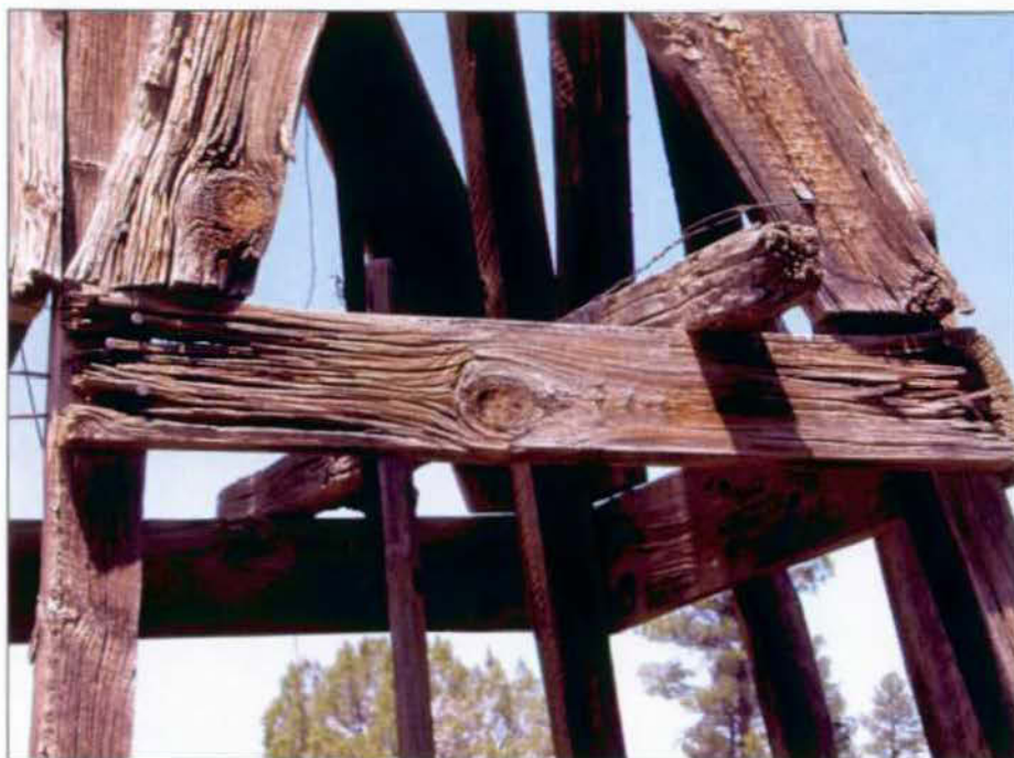
Detail of windmill structure.
