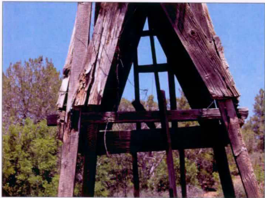
Detail of middle portion of structure.
