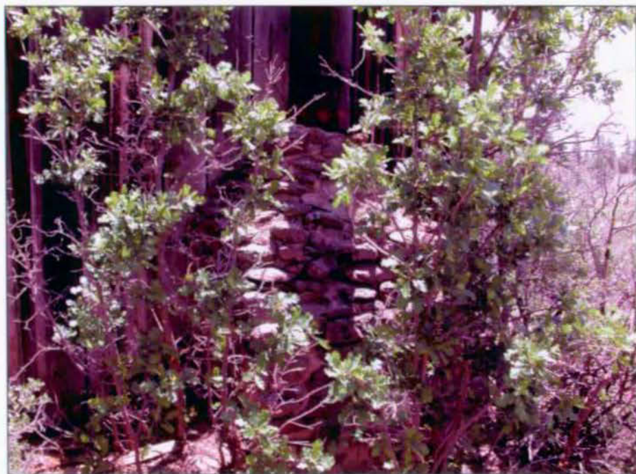
Detail of fireplace on west elevation. Note transition from stone to metal flue.
