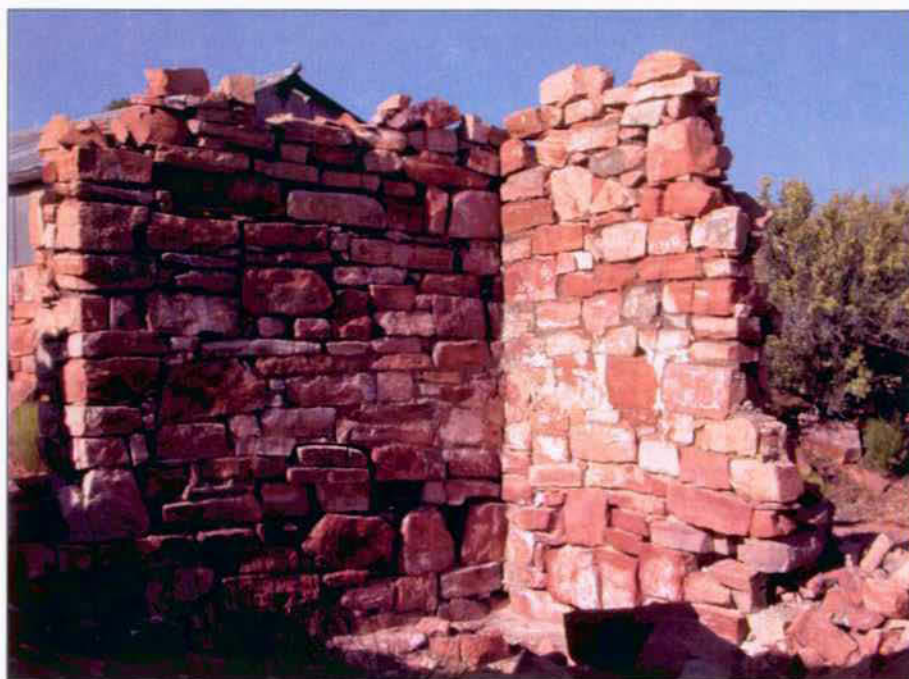
Detail of wall at southwest corner of room 1.
