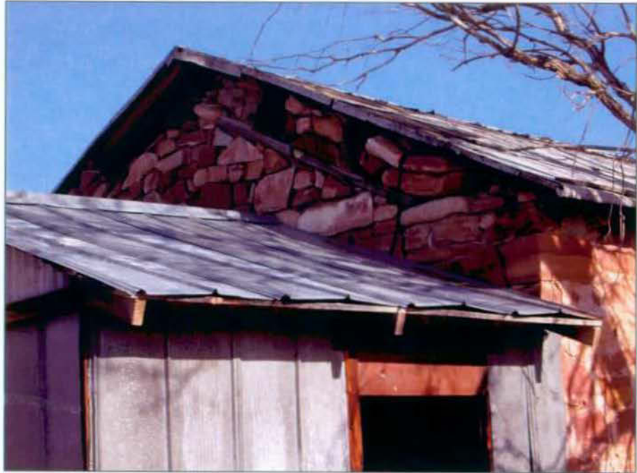
Detail of south gable end. Note stones piled between beams, on top of plate.
