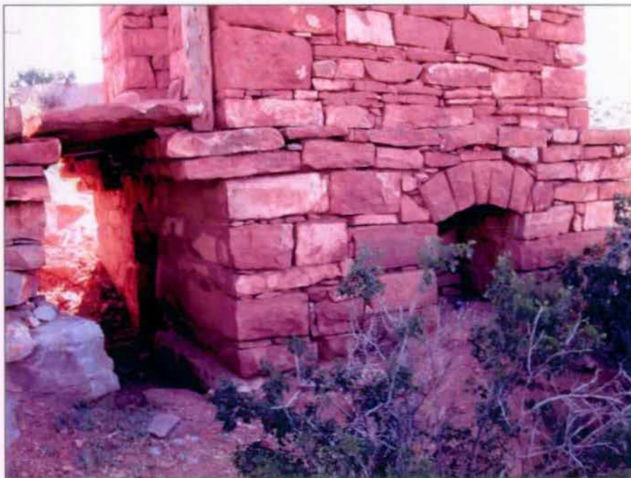
Detail of west elevation.
