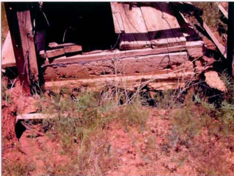
Detail of well underneath windmill. Note concrete enclosure, and wood cover.
