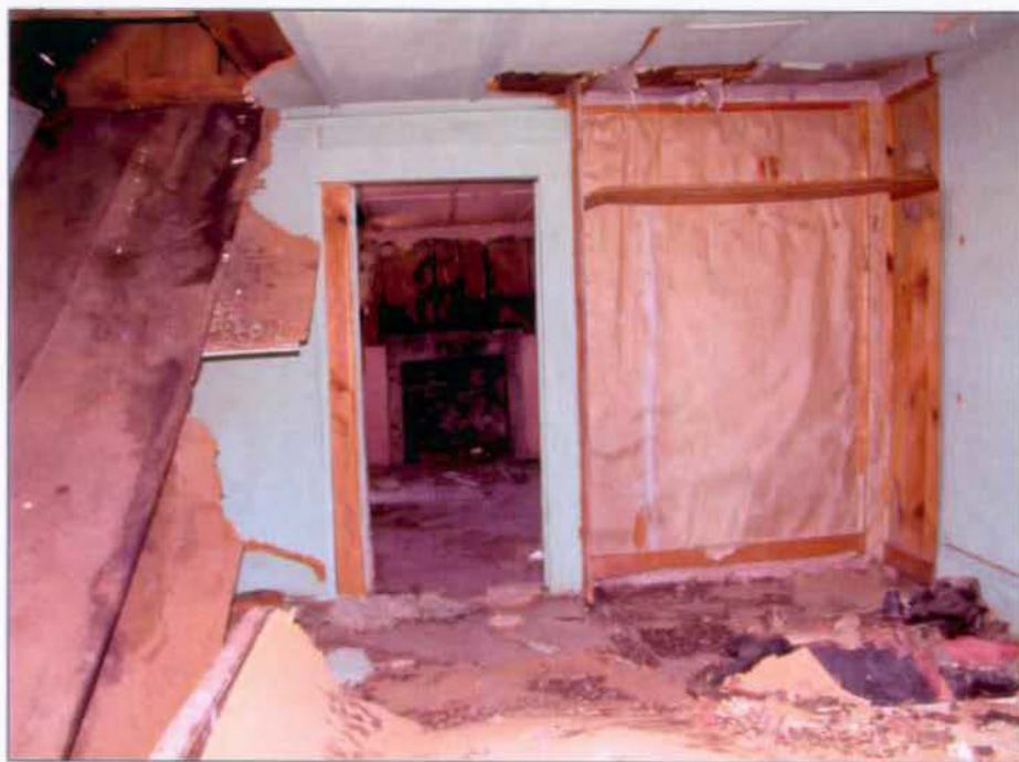
Interior of room2, looking west.
