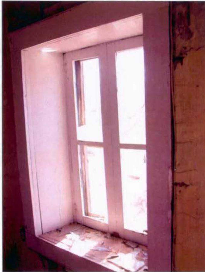
Detail of window in east wall, in room 3 (north room).
