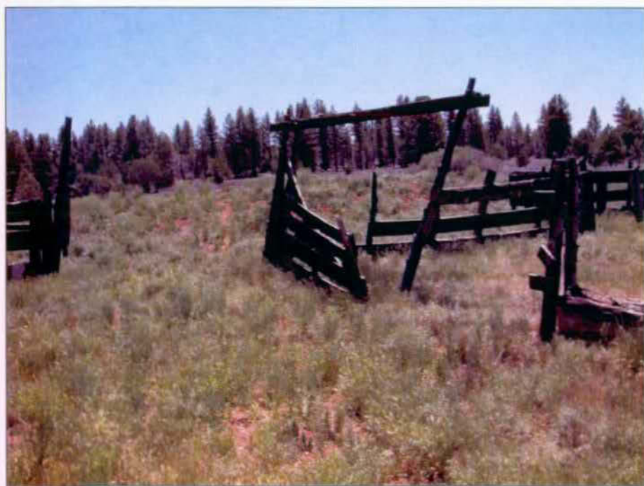
Fence and gate near loading ramp.
