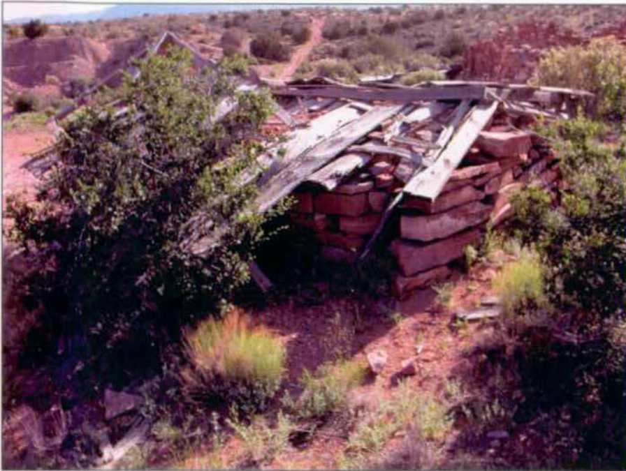
View from southwest.
