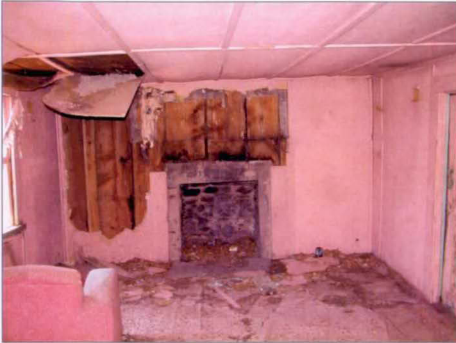
Interior of room 1, looking west. Note fireplace.
