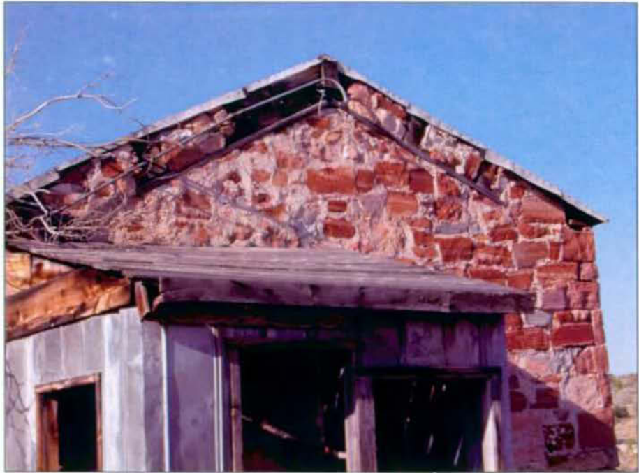
Detail of north gable end and roof of north addition.
