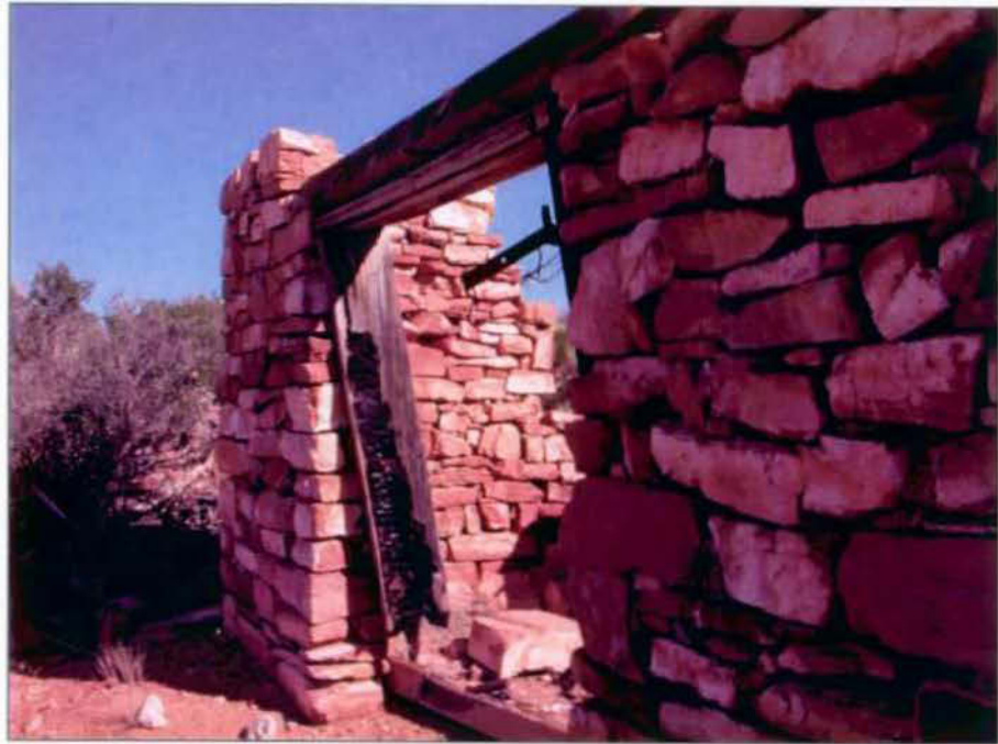
Detail of south wall showing doorway. Note charred jamb.
