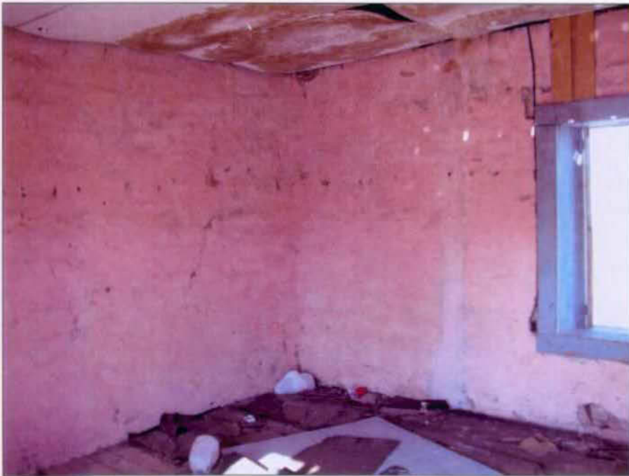
View of room 1 (south room), looking southeast.
