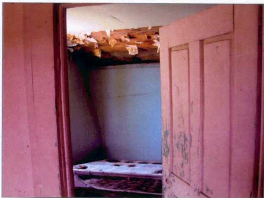
Interior of room 4, looking northwest through door from southwest room.
