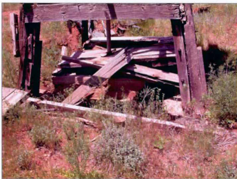
Detail of base of windmill structure. Note well below.
