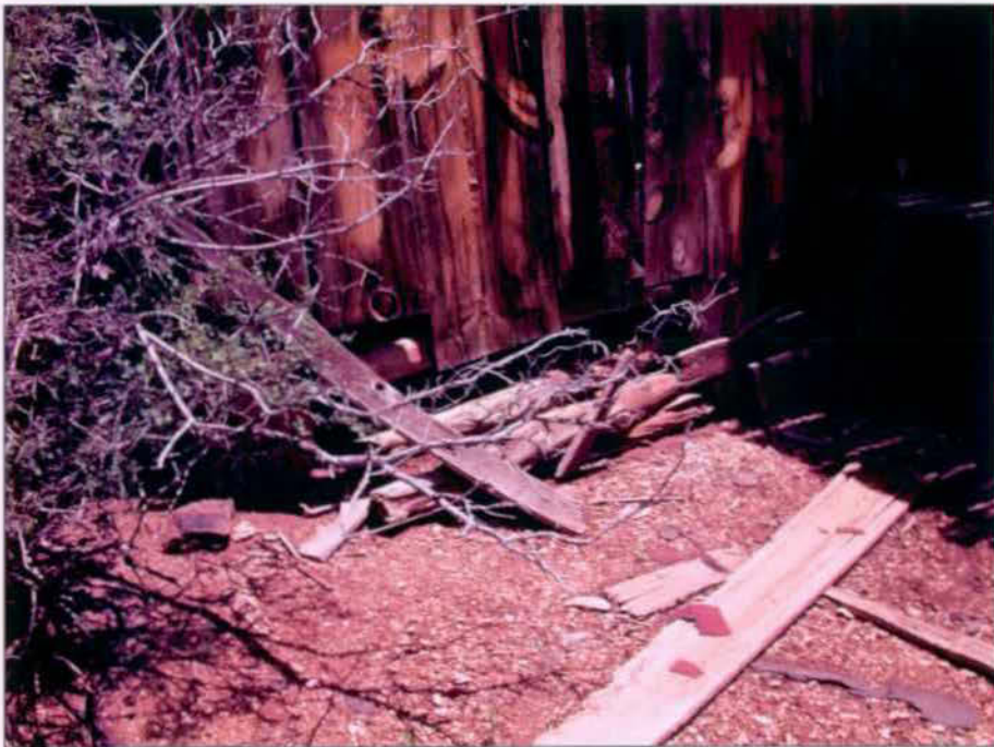
Detail of west end of south elevation. Note log skirting.
