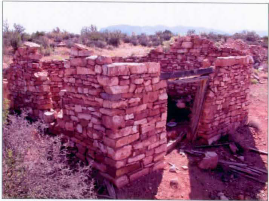
View from southwest, showing doorway.
