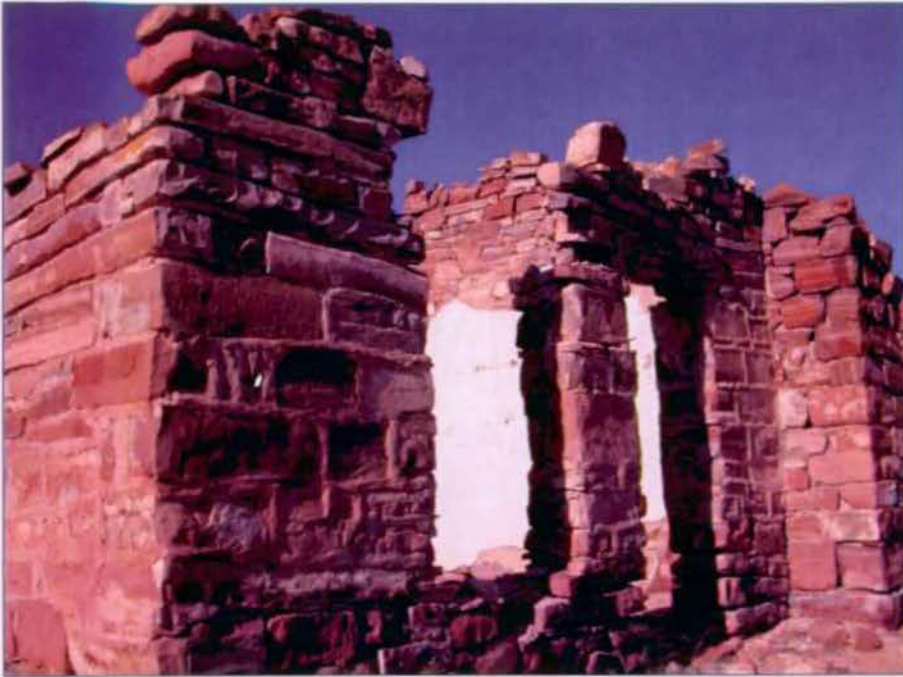
Close-up of north wall of addition. Note mortar joints.
