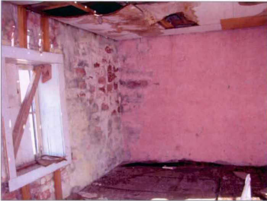
View of room 3 (north room), looking northwest.
