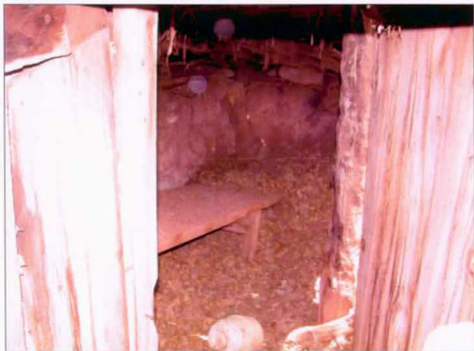
Detail of interior from doorway on south.
