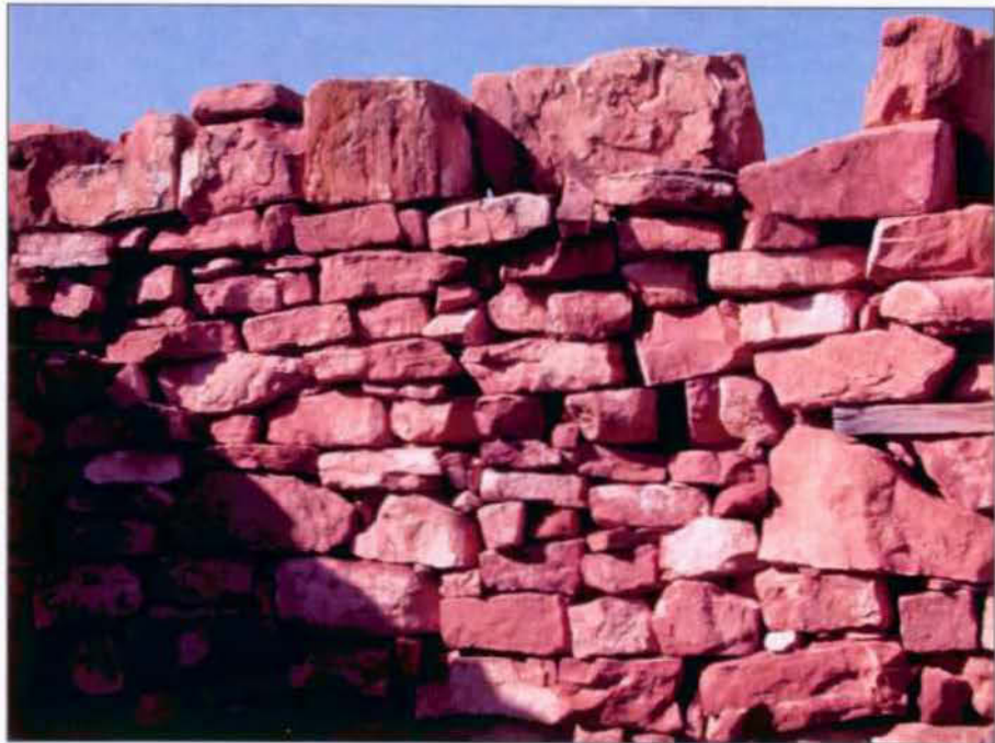
Detail of stone wall, showing header/bond course at top.
