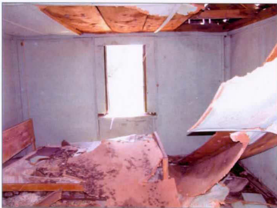
Interior of room 2, looking east.
