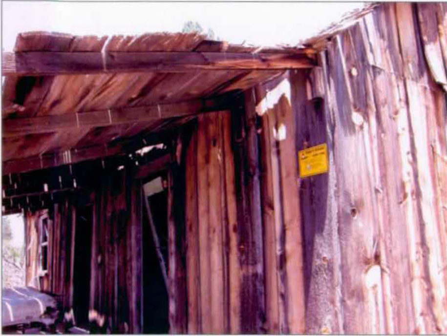
Detail of east end of porch.
