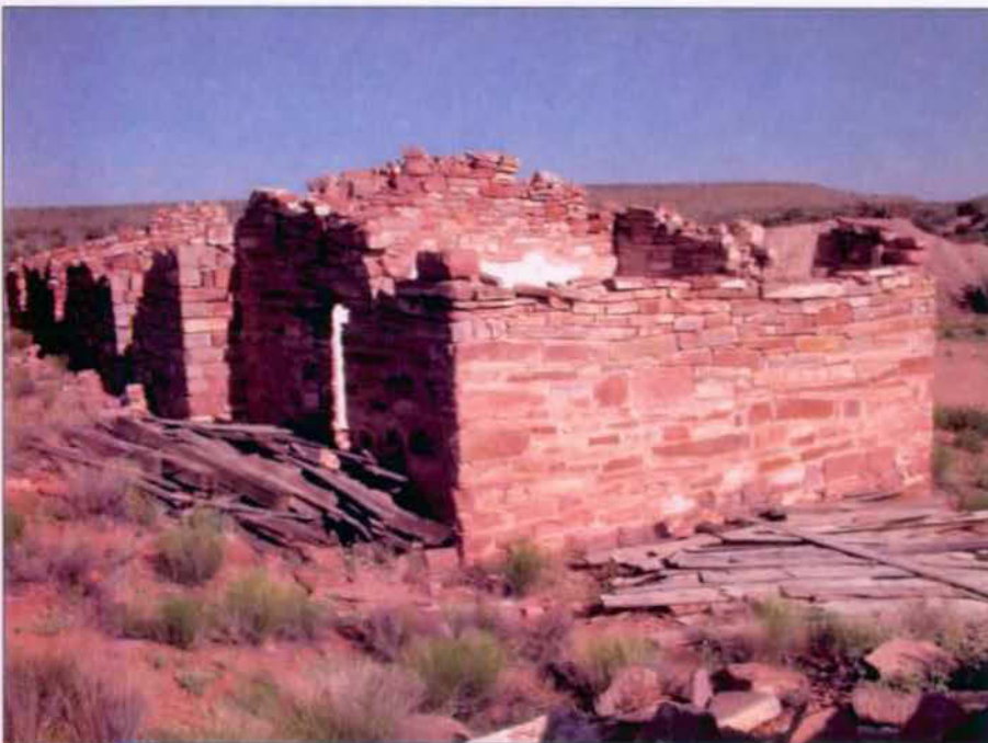
View from southeast, addition in foreground. Note walls rising to peak in center.
