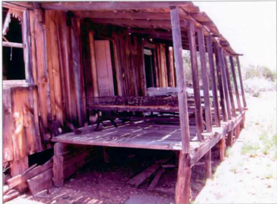
Detail of west end of porch, and south wall. Note posts and beams supporting floors and walls, displaced framing, and skirting at original cabin.
