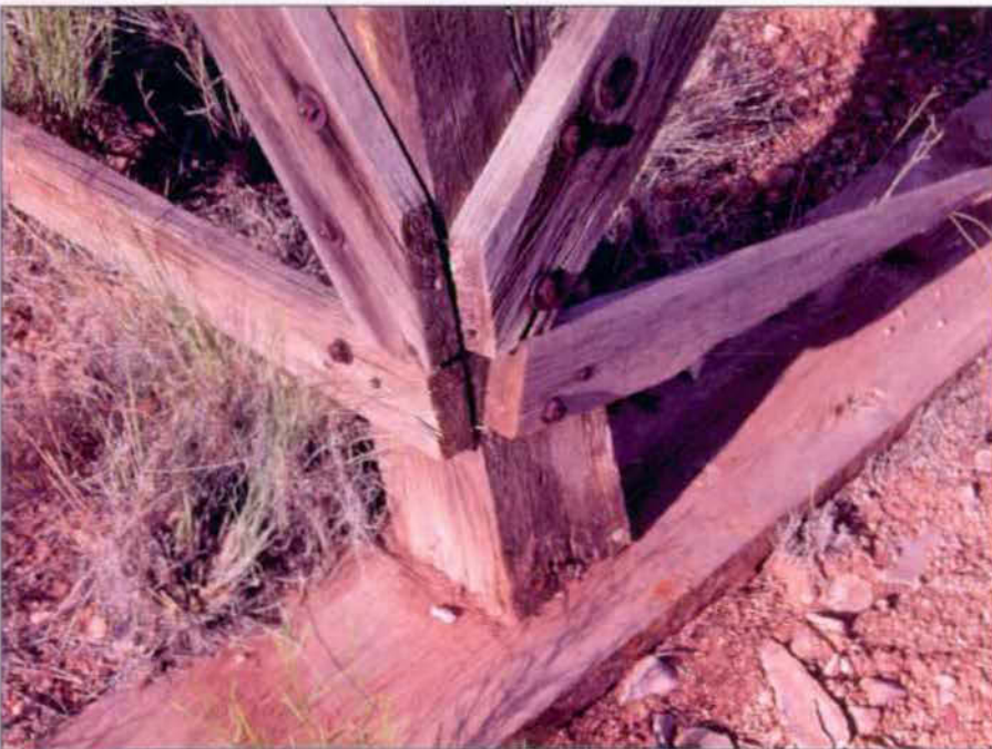
Detail of connection at bottom. Note bolted joints, and posts sitting on 2x12 plate.
