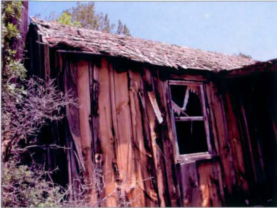
Detail of west end of south elevation. Note siding
