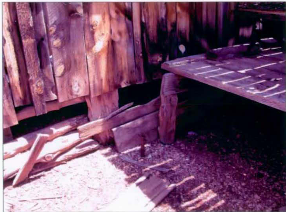
Detail of west end of south wall. Note posts and beams supporting floors and walls, and skirting at original cabin.
