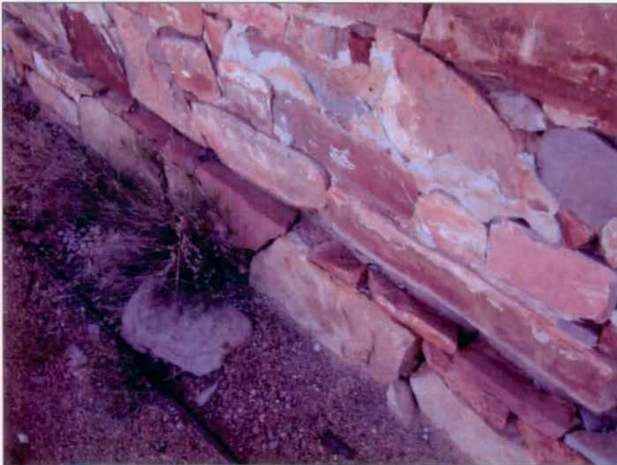
Detail of "water table" at bottom of west wall.
