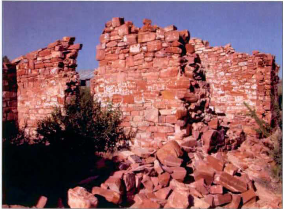
Interior of room 3. Note walls rising to peak in center.
