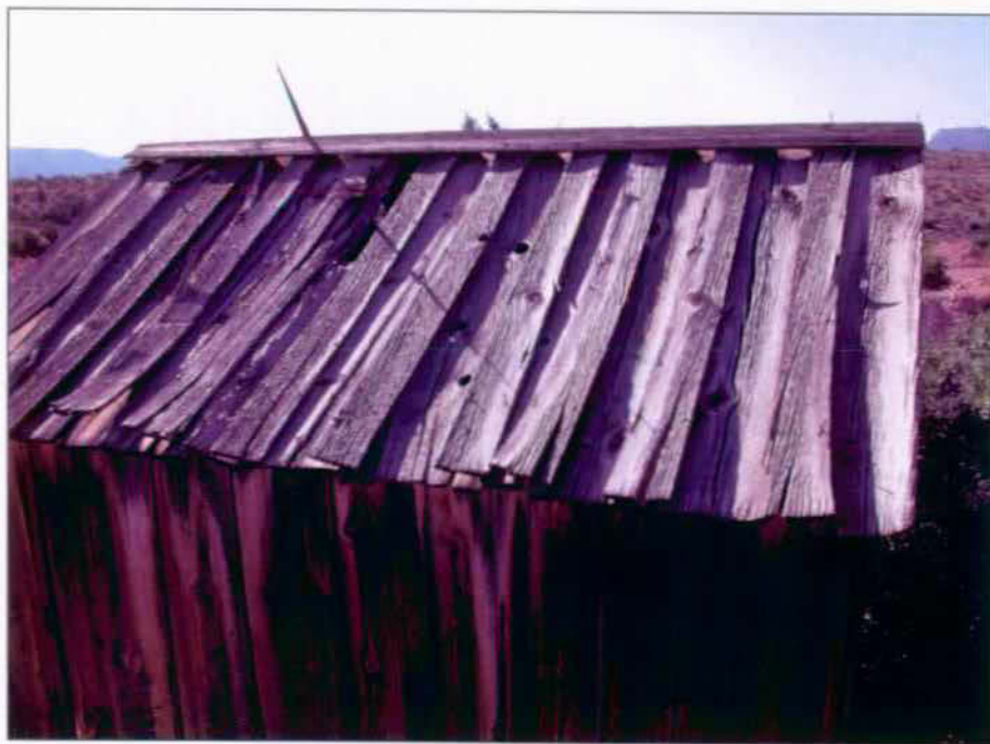
Detail of roof. Note board and batten structure.
