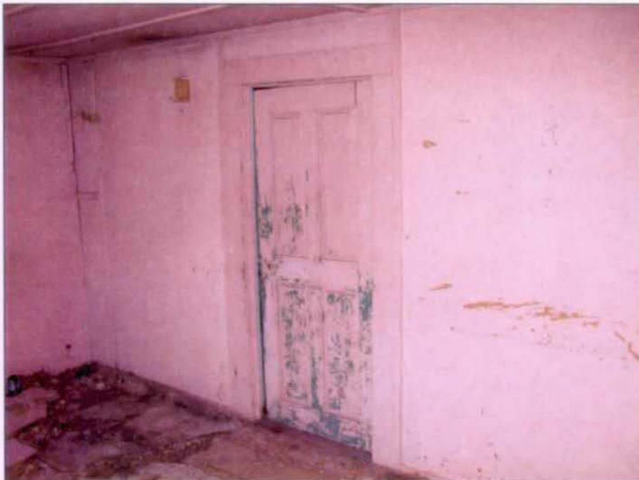
Interior of room 1, looking northwest, at door into northwest room.
