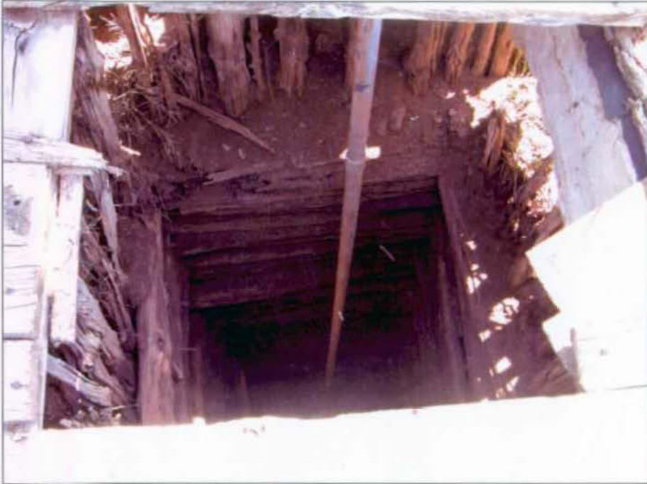
Detail of interior of well. Note log liner.
