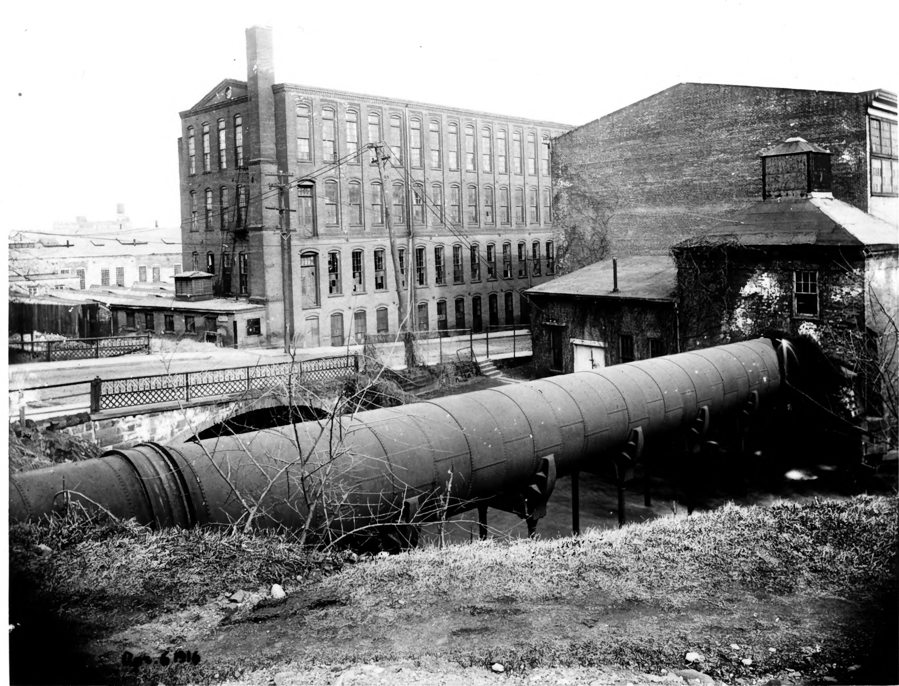
Plate 7 - Ivanhoe Wheelhouse with penstock, April 6, 1916, Reid Studio
