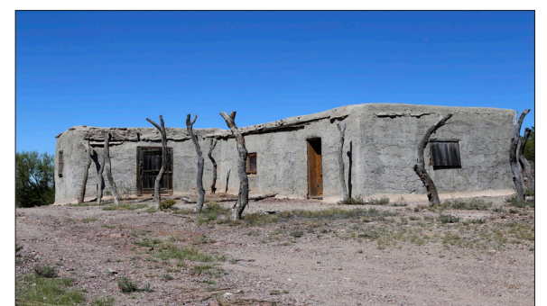
Ranch House at Blankenship Well
