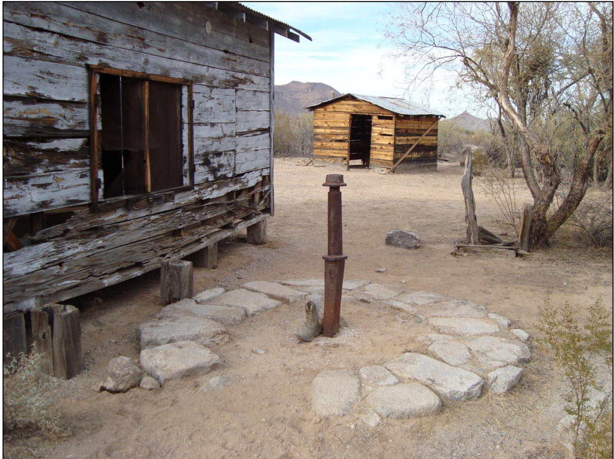
Figure 17. The remains of the arrastra at Bates Well Ranch. A large (ore-cart?) axle is used as the central fulcrum around which the burro dragged the heavy boulder to pulverize and separate the ore. The axle is likely not the original fulcrum. The cowboy bunkhouse (left) was moved to its location after the arrastra fell into dis-use, because there is not enough clearance to operate the arrastra at present. A small cowboy boot shrine was placed on the arrastra in memory of an unknown cowboy. Facing north.
