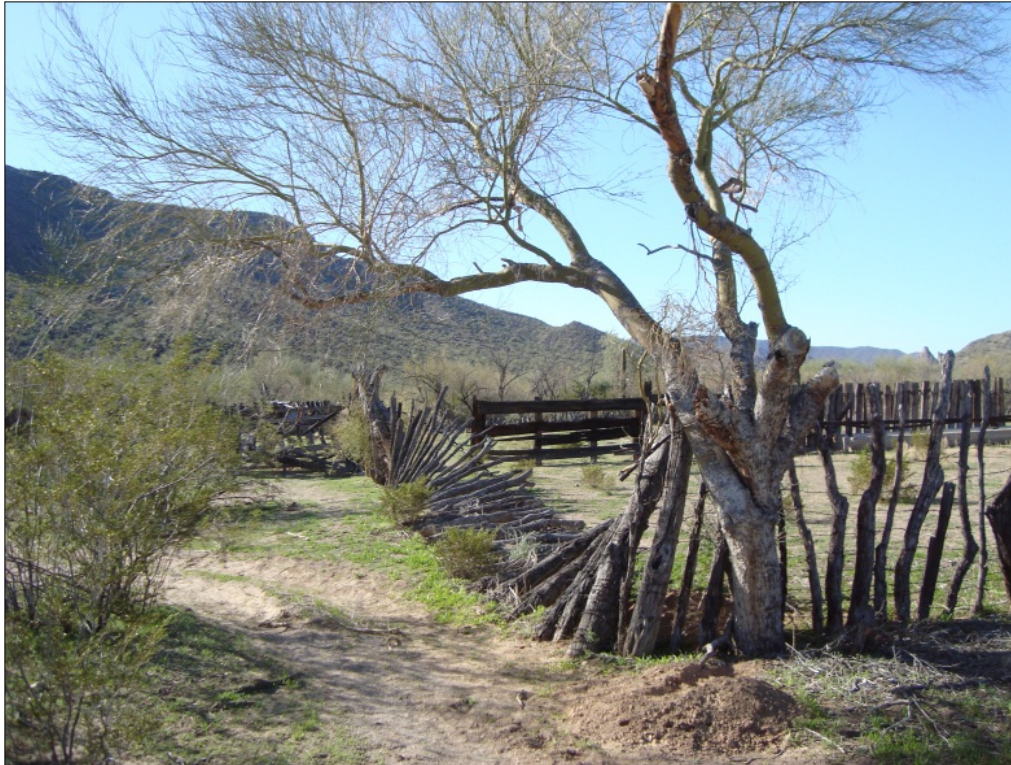
Figure 13. Collapsing corral fences at the Bates Well eastern corral, January 2010, facing south.
