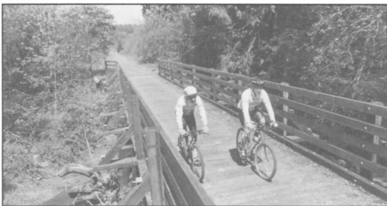
Fig. 46. The bicycle, hiking and equestrian trail at Banks-Vernonia State Park is a 21-mile linear park feature situated near the base of the Coast Range, on the west edge of the lower Willamette Valley. It is one of the few trails in the State Parks system to be developed from abandoned railroad right-of-way. 1991.
