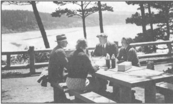
Fig. 6. Picnickers enjoy day-use facilities at Devil's Punchbowl State Park on the central Oregon coast. Fence rails and picnic table assemblies of peeled logs were crafted by CCC workers to harmonize with the surroundings in accordance with National Park Service guidelines. 1940s. Ralph Gifford Photo #490, Oregon State Highway Department.
