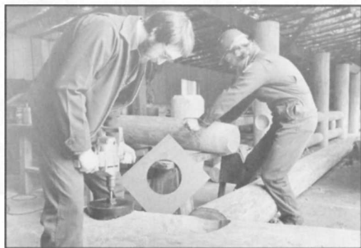
Fig. 40. Downed trees from the forested terrain of Silver Creek Canyon were located to reproduce deteriorated members of the Silver Falls Lodge veranda during the 1980 restoration effort. Park ranger John Allen, left, and park aide Wally Judd use a combination of traditional hand tools and power tools to finish porch railing assemblies in the shop. 1980.
