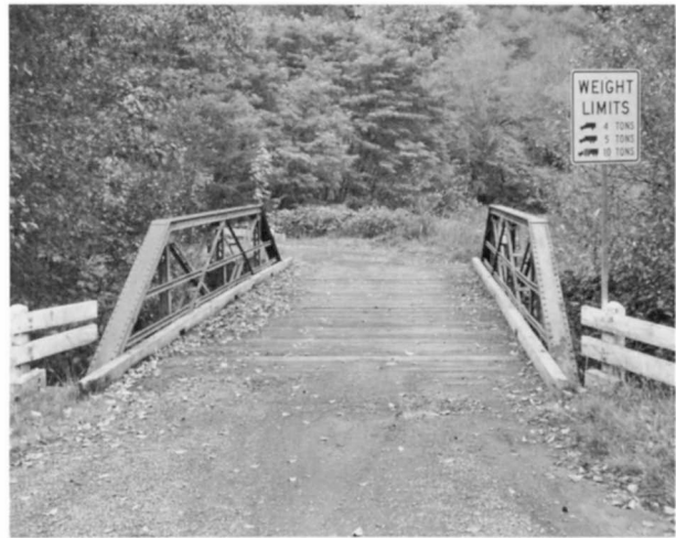
Beaver Creek (Kukkla Road) Bridge Structure Number 9C83 Constructed - Ca. 1915 (Site-1964) Steel Pony Truss (Double-Intersection Warren) Kukkla County Road 4087 Clatskanie vicinity, Columbia County Ownership - Columbia County
