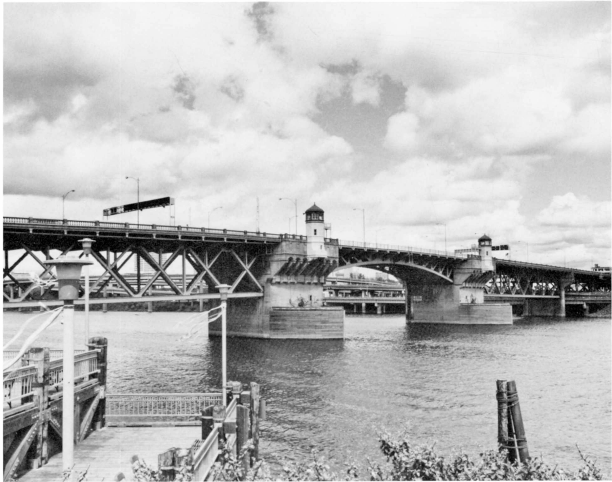
Structure Number 511 Constructed - 1926 Burnside Street Steel Double-Leaf Bascule Portland, Multnomah County Ownership - Multnomah County
