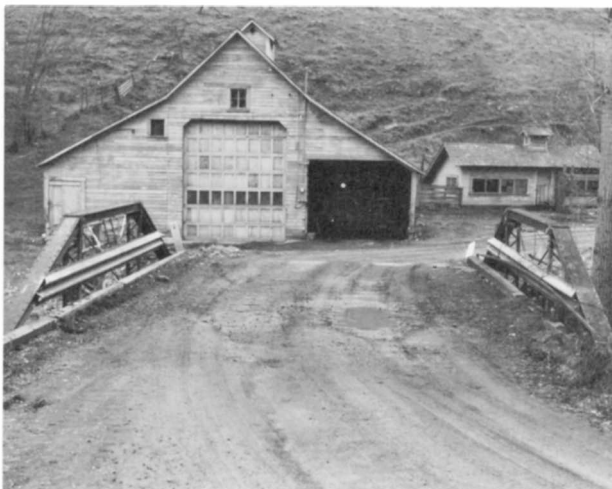
Pine Creek Bridge Structure Number 10712 Constructed - Ca. 1910 (Site-1936) Steel Pony Truss (Queenpost) County Road 676 Weston vicinity, Umatilla County Ownership - Umatilla County
