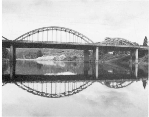
South Umpqua River (Winston) Bridge Structure Number 1923 Constructed - 1934 Steel Through Tied Arch Coos Bay-Roseburg Highway 35, M.P. 74.47 Winston vicinity, Douglas County Ownership - State of Oregon
