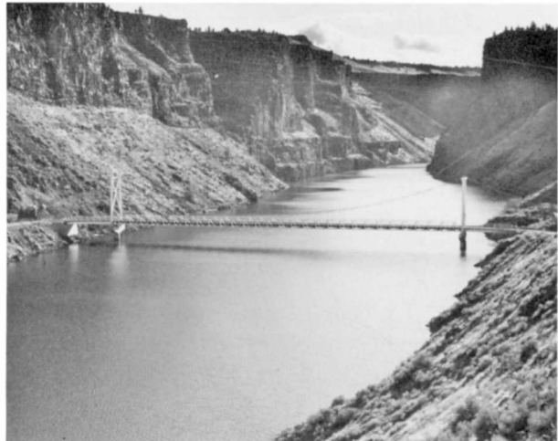
Crooked River (Lake Billy Chinook) Bridge Structure Number 16C06 Constructed - 1962 Steel Suspension Jordan County Road 579 Madras vicinity, Jefferson County Ownership - Jefferson County
