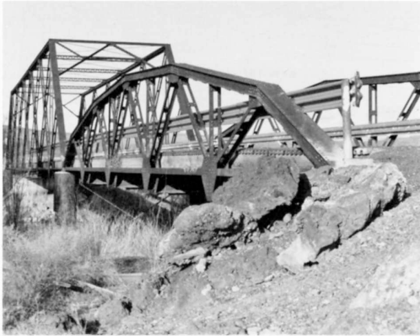
Crooked River (Elliott Lane) Bridge Structure Number 7C12 Constructed - Ca. 1914 (Site-1936) Steel Through Truss (Double-Intersection Warren) Elliott Lane County Road 124 Prineville vicinity, Crook County Ownership - Crook County
