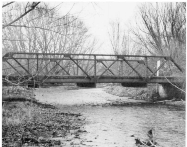
Pine Creek (Crow Lane) Bridge Structure Number 1C826 Constructed - 1911 Steel Pony Truss (Warren) Crow Lane County Road 1027 Halfway vicinity, Baker County Ownership - Baker County
