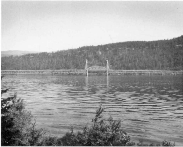
Columbia River (White Salmon) Bridge Structure Number 6645 Constructed - 1924 Steel Through Truss (Pennsylvania-Petit) Vertical Lift Port Road connecting with Columbia River Highway 2, M.P. 64.62 Hood River, Hood River County (Oregon) and White Salmon, Klickitat County (Washington) Ownership - Port of Hood River
