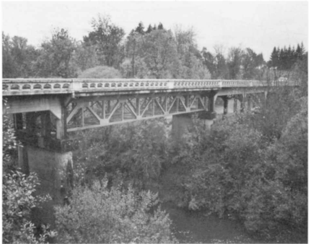
North Yamhill River Bridge Structure Number 441 Constructed - 1921 Steel Deck Truss (Warren with Verticals) Pacific Highway West 1W, M.P. 34.99 McMinnville vicinity, Yamhill County Ownership - State of Oregon
