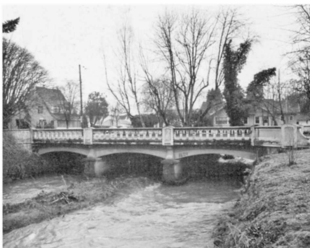
Mill Creek (Summer Street, N.E.) Bridge Structure Number 1357S Constructed - 1929 Reinforced Concrete Deck Girder Pacific Highway East 1E, M.P. 49.28 Salem, Marion County Ownership - State of Oregon
