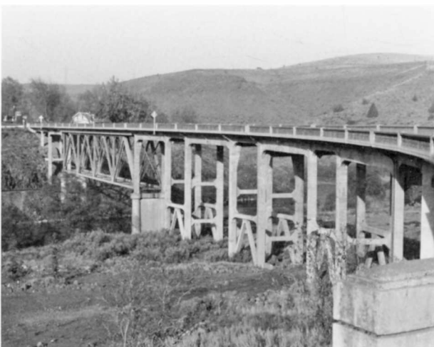
Deschutes River (Maupin) Bridge Structure Number 966 Constructed - 1929 Steel Deck Truss (Warren) The Dalles-California Highway 4, M.P. 45.87 Maupin vicinity, Wasco County Ownership - State of Oregon
