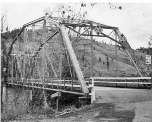
South Umpqua River (Worthington) Bridge Structure Number 7408 Constructed - Ca. 1910 (Site-1951) Steel Through Truss (Pennsylvania-Petit) County Road 42, M.P. 8.82 Days Creek, Douglas County Ownership - Douglas County
