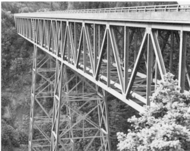
Thomas Creek Bridge Structure Number 8459 Constructed - 1961 Steel Deck Truss (Warren with Verticals) Oregon Coast Highway 9, M.P. 374.78 Brookings vicinity, Curry County Ownership - State of Oregon
