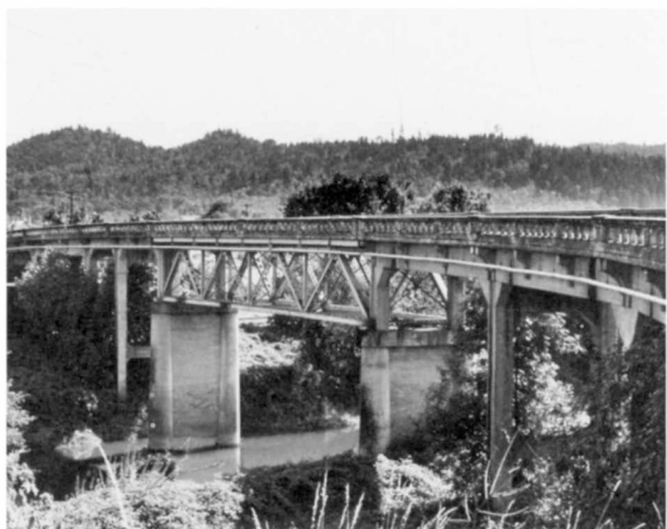
Calapooya Creek (Oakland) Bridge Structure Number 603 Constructed - 1925 Steel Deck Truss (Warren) Oakland-Shady Highway 324, M.P. 1.08 Oakland, Douglas County Ownership - Douglas County
