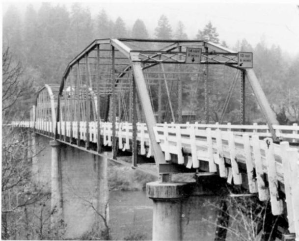
Rogue River (Robertson) Bridge Structure Number 1592 Constructed - Ca. 1909 (Site-1929) Steel Through Truss (Parker) Rogue River Loop Highway 260, M.P. 12.91 Merlin Vicinity, Josephine County Ownership - State of Oregon
