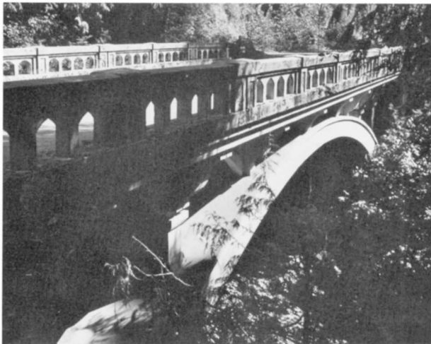
Soapstone Creek Bridge Structure Number 1319 Constructed - 1928 Reinforced Concrete Deck Arch Necanicum Highway 46, M.P. 6.50 Necanicum Junction vicinity, Clatsop County Ownership - State of Oregon
