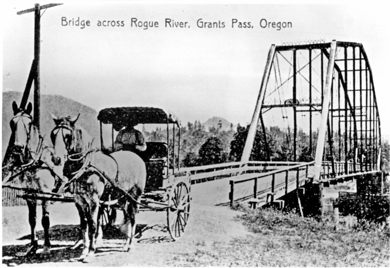
FIGURE 7. Typical of the early metal high truss bridges in Oregon is this span across the Rogue River at Grants Pass, circa 1890. (Photograph courtesy of the Josephine County Historical Society.)
