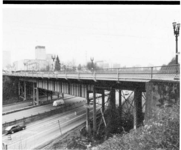
N.E. Grand Avenue Overcrossing Structure Number 7040 Constructed - 1907 Steel Deck Girder Pacific Highway East 1E, M.P. 0.20 Portland, Multnomah County Ownership - State of Oregon
