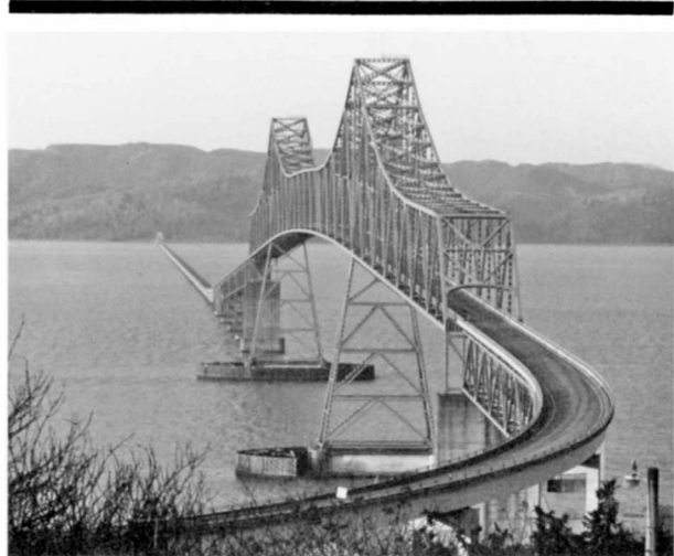
Columbia River (Astoria) Bridge Structure Number 7949 Constructed - 1966 Steel Through Truss (Cantilever) Oregon Coast Highway 9, M.P. 0.00 Astoria, Clatsop County (Oregon) and Megler vicinity, Pacific County (Washington) Ownership - State of Oregon
