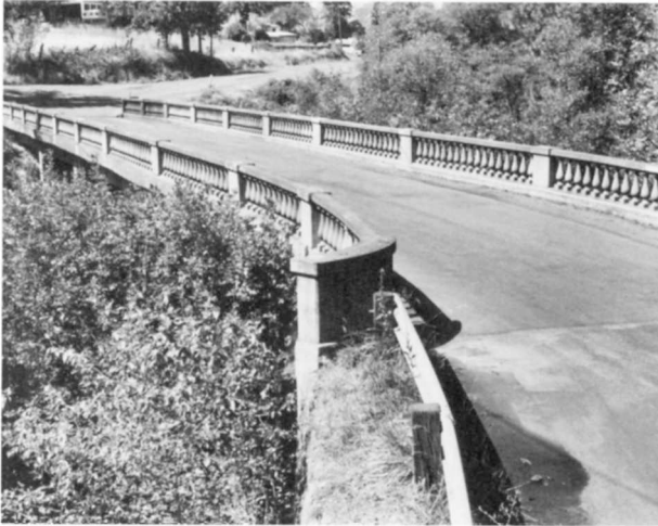
Mosier Creek (State Road) Bridge Structure Number 118 Constructed - 1917 Reinforced Concrete Deck Girder State (County) Road Mosier vicinity, Wasco County Ownership - Wasco County
