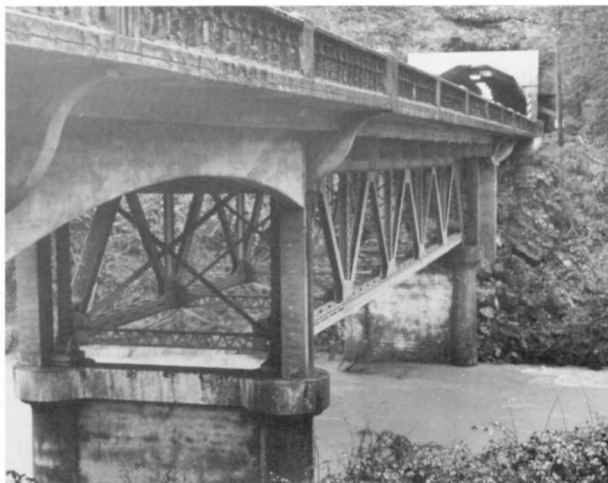
Elk Creek (Fourth Crossing) Bridge Structure Number 1406 Constructed - 1931 Steel Deck Truss (Warren with Verticals) Umpqua Highway 45, M.P. 39.97 Elkton vicinity, Douglas County Ownership - State of Oregon
