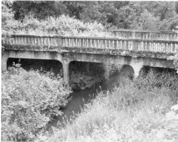
McCarthy Creek Bridge Structure Number Unknown Constructed - Ca. 1914 Reinforced Concrete Deck Girder Lower Columbia River Highway 2W, M.P. 13.19 (Bypassed) Portland vicinity, Multnomah County Ownership - State of Oregon
