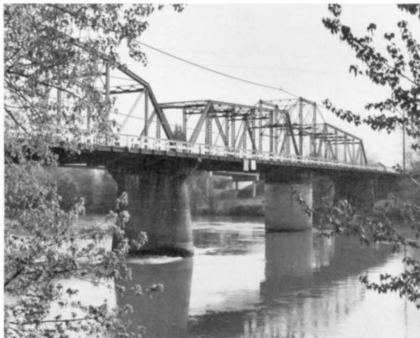
Willamette River (Van Buren Street) Bridge Structure Number 2728 Constructed - 1913 Steel Through Truss (Pratt) Swing Corvallis-Lebanon Highway 210, M.P. 0.13 Corvallis, Benton-Linn counties Ownership - State of Oregon
