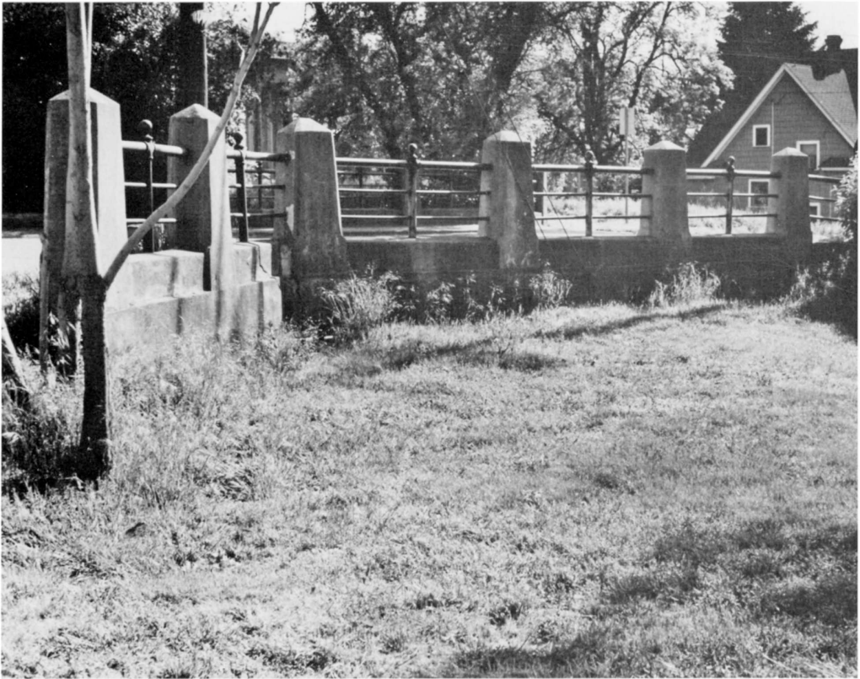
Structure Number 24TO4 Constructed - 1914 S.E. Court Place Reinforced Concrete Slab Pendleton, Umatilla County Ownership - City of Pendleton
