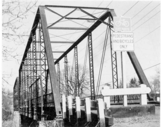
South Yamhill River (Steel) Bridge Structure Number 53C05 Constructed - Ca. 1910 Steel Through Truss (Pratt) County Road 669 (Closed) Willamina, Polk County Ownership - Polk County
