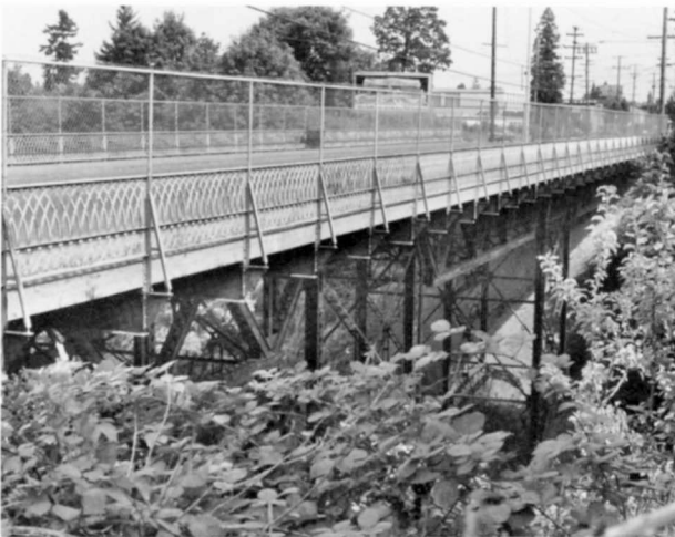
North Lombard Street Overcrossing Structure Number 6.2 Constructed - 1909 Steel Deck Truss (Warren) North Lombard Street Portland, Multnomah County Ownership - Burlington Northern Railroad
