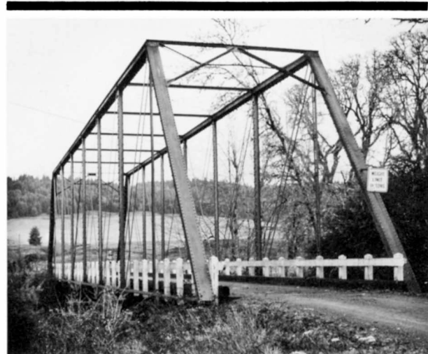
Luckiamute River (Grant Road) Bridge Structure Number 53C139 Constructed - 1918 (Site-1958) Steel Through Truss (Pratt) Grant County Road 1062 Kings Valley vicinity, Polk County Ownership - Polk County
