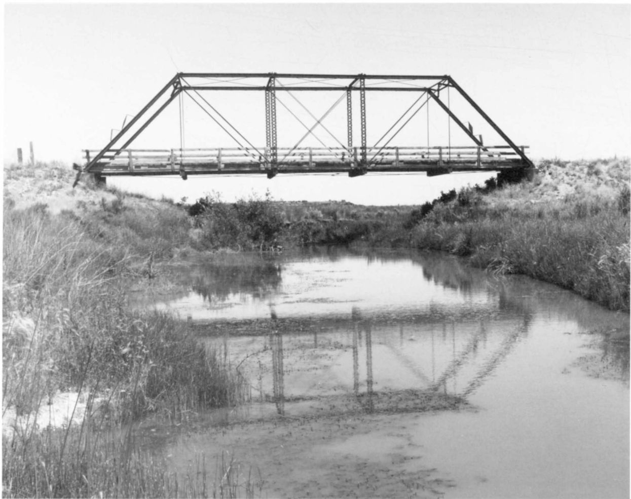
Structure Number 45C609 Constructed - Ca. 1910 County Road 793 Steel Through Truss (Pratt) Danner vicinity, Malheur County Ownership - Malheur County
