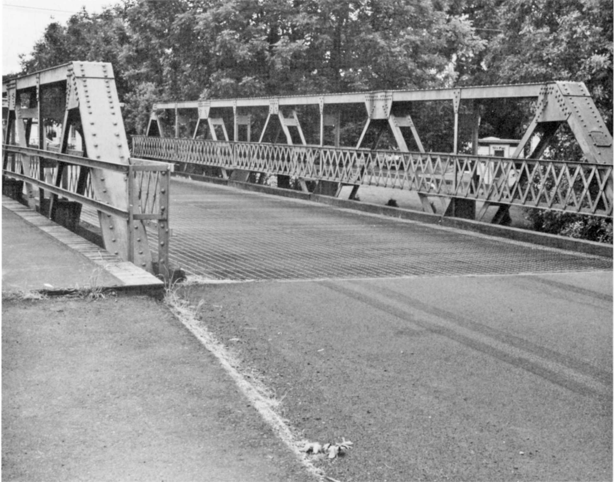
Structure Number 13757 Constructed - 1914 Milton Way Steel Pony Truss (Warren) St. Helens, Columbia County Ownership - City of St. Helens
