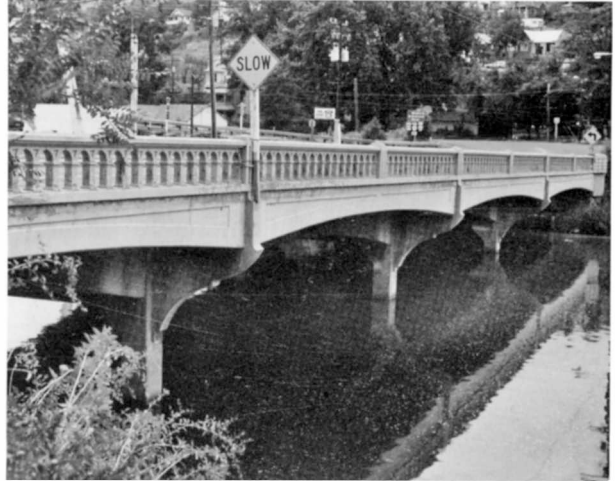
Link River Bridge Structure Number 1579 Constructed - 1931 Reinforced Concrete Deck Girder Klamath Falls-Lakeview Highway 20, M.P. 0.02 Klamath Falls, Klamath County Ownership - State of Oregon
