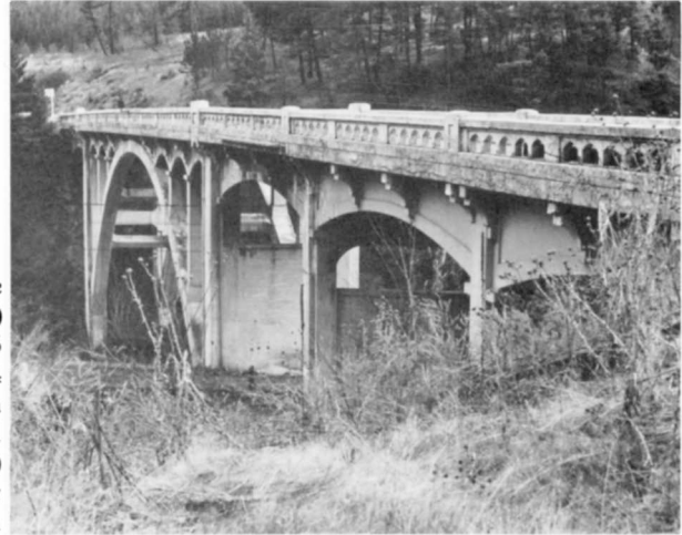
Grande Ronde River Bridge (Perry Overcrossing) Structure Number 626 Constructed - 1924 Reinforced Concrete Deck Arch Old Oregon Trail Highway 6, M.P. 256.31 (Frontage Road) La Grande vicinity, Union County Ownership - State of Oregon
