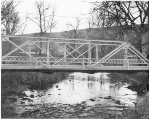
Powder River (Myrtle Street) Bridge Structure Number 4T04 Constructed - 1920 Steel Pony Truss (Pratt) Myrtle Street Baker, Baker County Ownership - Baker County
