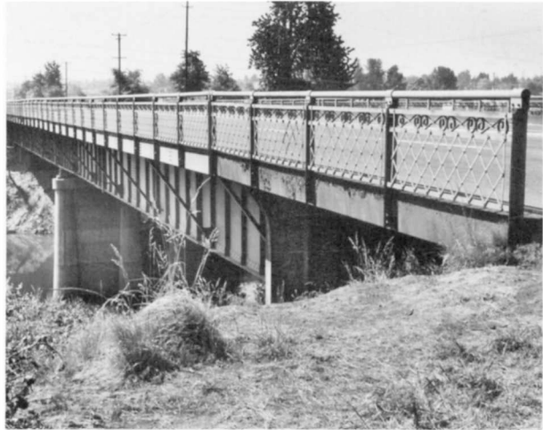
Columbia Slough (N.E. Union Avenue) Bridge Structure Number 1377C Constructed - 1916 Steel Deck Girder N.E. Union Avenue Crossing of the Pacific Highway East 1E, M.P. 4.41 Portland, Multnomah County Ownership - State of Oregon
