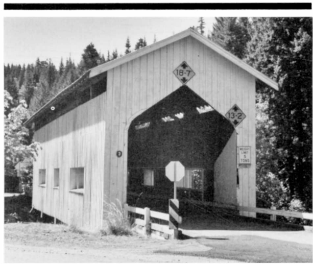
Little River (Cavitt Creek) Bridge Structure Number 19C18 Constructed - 1943 Timber Through Truss (Howe) Covered Bridge Cavitt Creek County Road 17 Glide vicinity, Douglas County Ownership - Douglas County
