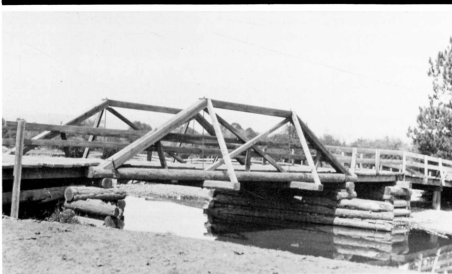
FIGURE 9. This timber and wrought iron queenpost truss is representative of early bridges in Oregon. Inexpensive, made of local materials, and constructed by local builders, these timber bridges were functional if not always long-lasting. (This bridge spanned Camas Creek near Ukiah, Umatilla County, and was built about 1900.)
