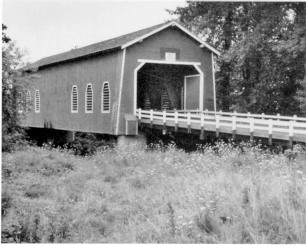
Thomas Creek (Shimanek) Bridge Structure Number 12965 Constructed - 1966 Timber Through Truss (Howe) Covered Bridge Richardson Gap County Road 673 Scio vicinity, Linn County Ownership - Linn County
