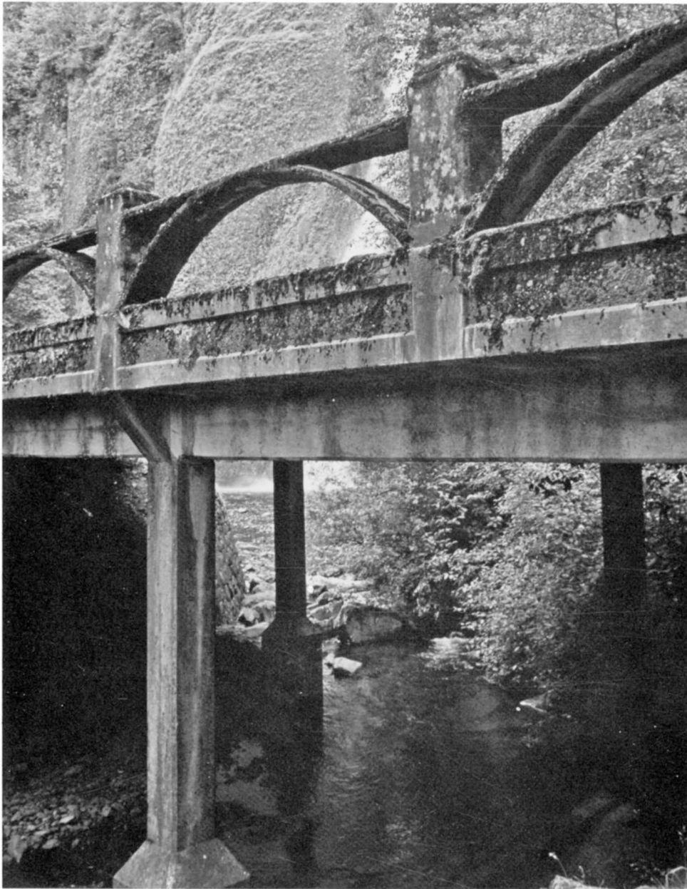
Structure Number 4543 Constructed - 1914 Crown Point Highway 125, M.P. 22.21 Reinforced Concrete Slab Oneonta vicinity, Multnomah County Ownership - State of Oregon
