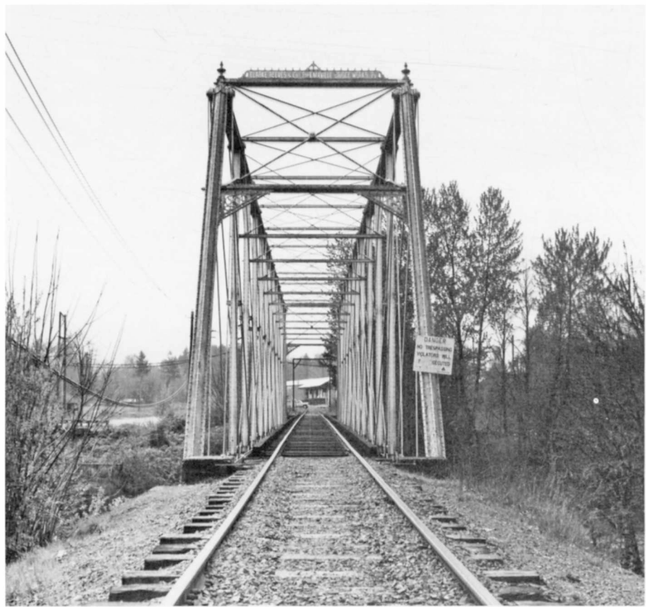
FIGURE 10. The Booth-Kelly Railroad Bridge (also called the Hayden Bridge) across the McKenzie River at Springfield is considered the oldest surviving bridge in Oregon. The wrought iron truss structure was first erected near Corrine, Utah, in 1882 and was moved to its present location in 1900. The Whipple truss and Phoenix columns make it a unique structure.
