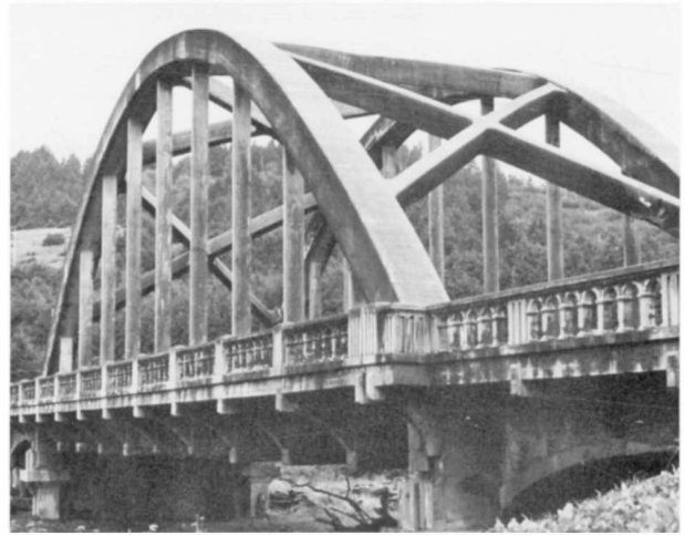
Big Creek Bridge Structure Number 1180 Constructed - 1931 Reinforced Concrete Through Tied Arch Oregon Coast Highway 9, M.P. 175.02 Heceta Head vicinity, Lane County Ownership - State of Oregon
