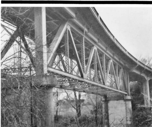
Elk Creek (First Crossing) Bridge Structure Number 1614 Constructed - 1931 Steel Deck Truss (Warren with Verticals) Umpqua Highway 45, M.P. 36.39 Elkton vicinity, Douglas County Ownership - State of Oregon
