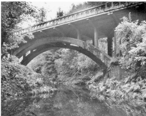
Salmon River Bridge Structure Number 4192 Constructed - 1930 Reinforced Concrete Deck Arch Salmon River Highway 39, M.P. 6.23 Rose Lodge vicinity, Lincoln County Ownership - State of Oregon
