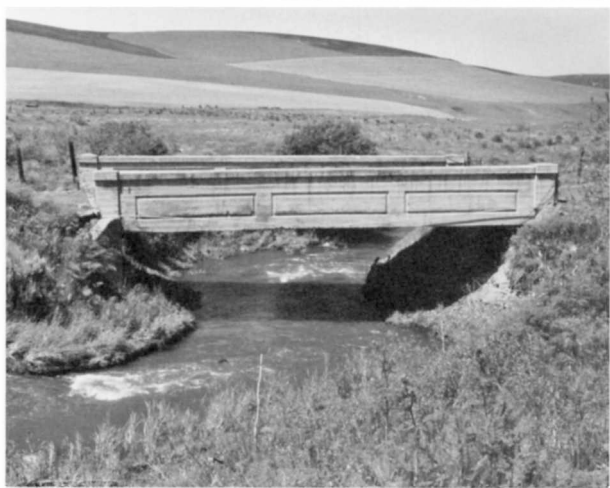
Rhea Creek Bridge Structure Number 49C23 Constructed - 1916 Reinforced Concrete Through Girder Ruggs-Jordan County Road 581 Jordan vicinity, Morrow County Ownership - Morrow County
