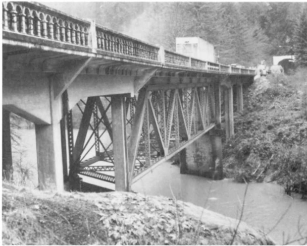
Elk Creek (Third Crossing) Bridge Structure Number 1465 Constructed - 1931 Steel Deck Truss (Warren with Verticals) Umpqua Highway 45, M.P. 39.64 Elkton vicinity, Douglas County Ownership - State of Oregon
