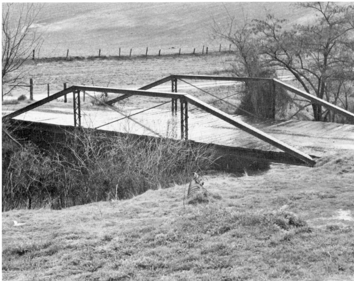
Structure Number 59C534 Constructed - Ca. 1910 (Site-1935) County Road 697 Steel Pony Truss (Queenpost) Umapine vicinity, Umatilla County Ownership - Umatilla County
