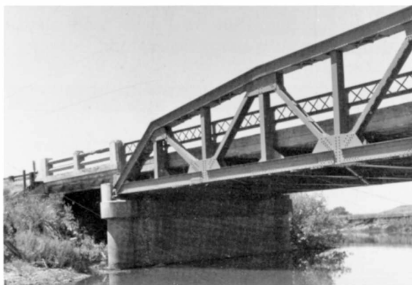
Riveted gusset plates form rigid truss joints which decrease the wear on individual bridge members and extend the service life. The riveted joint made the pin-connected joint obsolete.
