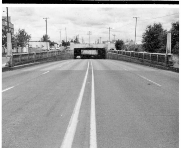
Portland Road, N.E., Undercrossing Structure Number 2131 Constructed - 1936 Steel Deck Girder Pacific Highway East 1E, M.P. 47.78 Salem, Marion County Ownership - State of Oregon
