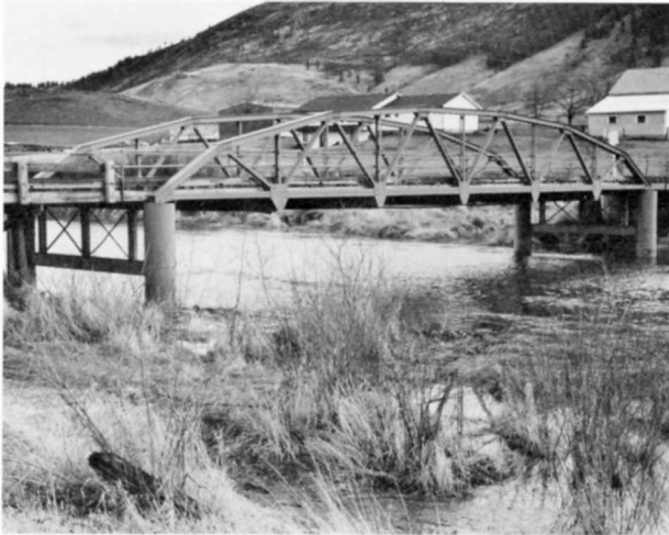
Grande Ronde River Bridge (McKennon Road) Structure Number 61C19 Constructed - 1925 Steel Pony Truss (Warren with Polygonal Upper Chords) McKennon County Road 132 Imbler vicinity, Union County Ownership - Union County
