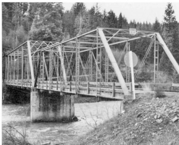
Grande Ronde River (Yarrington) Bridge Structure Number 61C16 Constructed - 1906 (Site-1925) Steel Through Truss (Pratt) Yarrington-Scott County Road 49 Palmer Junction, Union County Ownership - Union County
