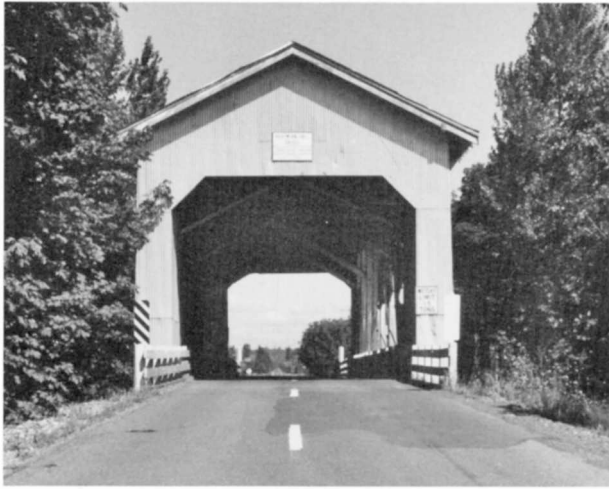
Crabtree Creek (Bohemian Hall) Bridge (Also, Richardson Gap Bridge) Structure Number 12890 Constructed - 1947 Timber Through Truss (Howe) Covered Bridge Richardson Gap County Road 25 Scio vicinity, Linn County Ownership - Linn County
