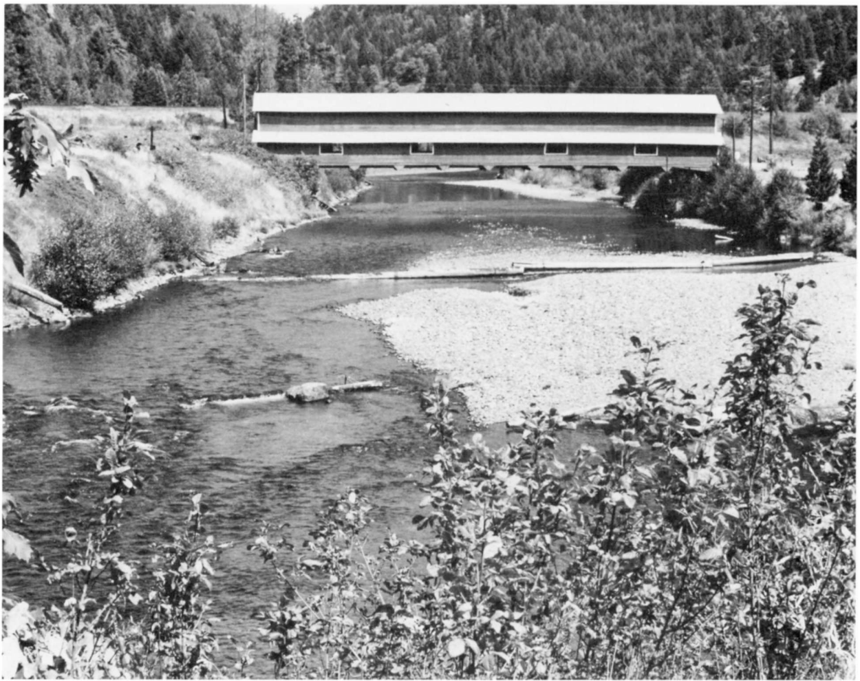
Structure Unnumbered Constructed - 1944 Private Road Timber Through Truss (Howe) Covered Bridge Westfir vicinity, Lane County Ownership - Private
