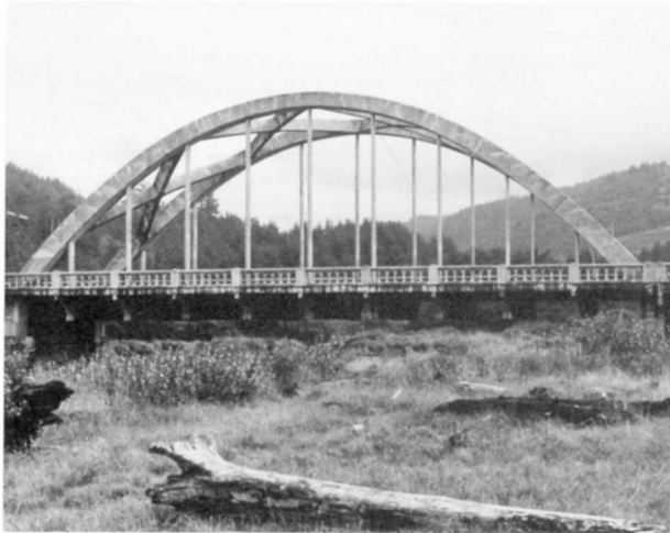
Tenmile Creek Bridge Structure Number 1181 Constructed - 1931 Reinforced Concrete Through Tied Arch Oregon Coast Highway 9, M.P. 171.44 Yachats vicinity, Lane County Ownership - State of Oregon
