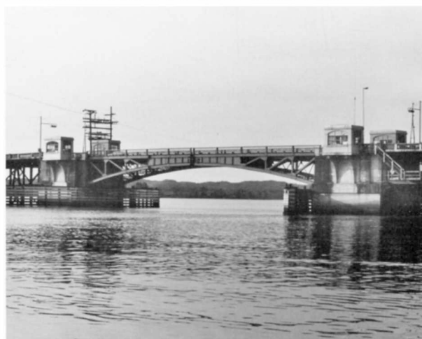
Old Young's Bay Bridge Structure Number 330 Constructed - 1921 Steel Double-Leaf Bascule Warrenton Highway 105, M.P. 6.89 Astoria vicinity, Clatsop County Ownership - State of Oregon
