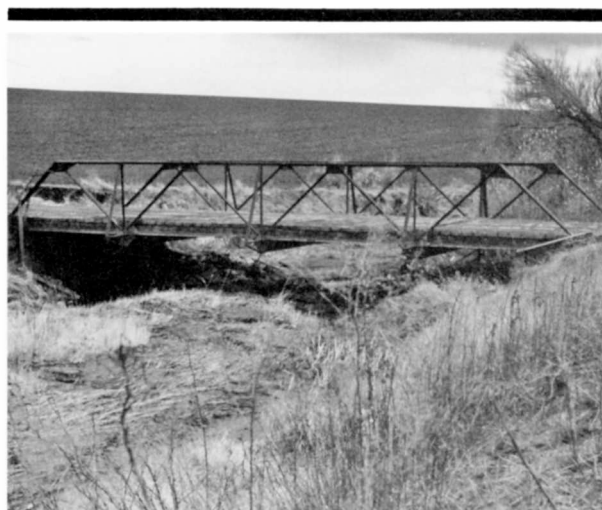
Greasewood Creek Bridge Structure Number 59C590 Constructed - 1907 (Site-1929) Steel Pony Truss (Warren) County Road 854 Adams vicinity, Umatilla County Ownership - Umatilla County
