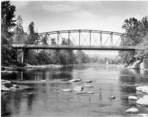
Clackamas River (Park Place) Bridge Structure Number 604 Constructed - 1921 Steel Through Truss (Parker) 82nd Avenue (Closed) Gladstone, Clackamas County Ownership - City of Gladstone
