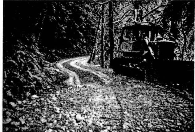
Graves Creek Road after grading and re-gravelling
