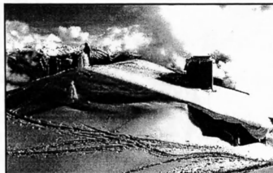
Hurricane Ridge Visitor Center buried in snow in mid March
