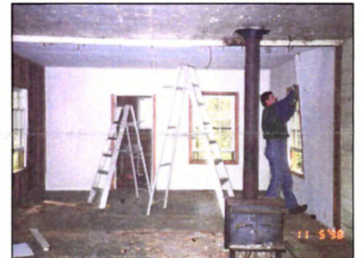
refurbishing station's interior
