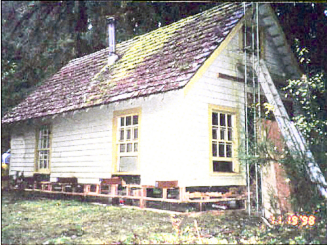
North Fork Quinault Ranger Station under repair
