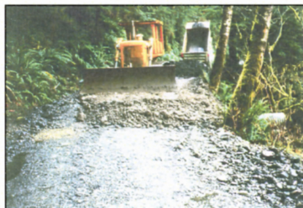
bulldozers resurfacing Graves Creek road
