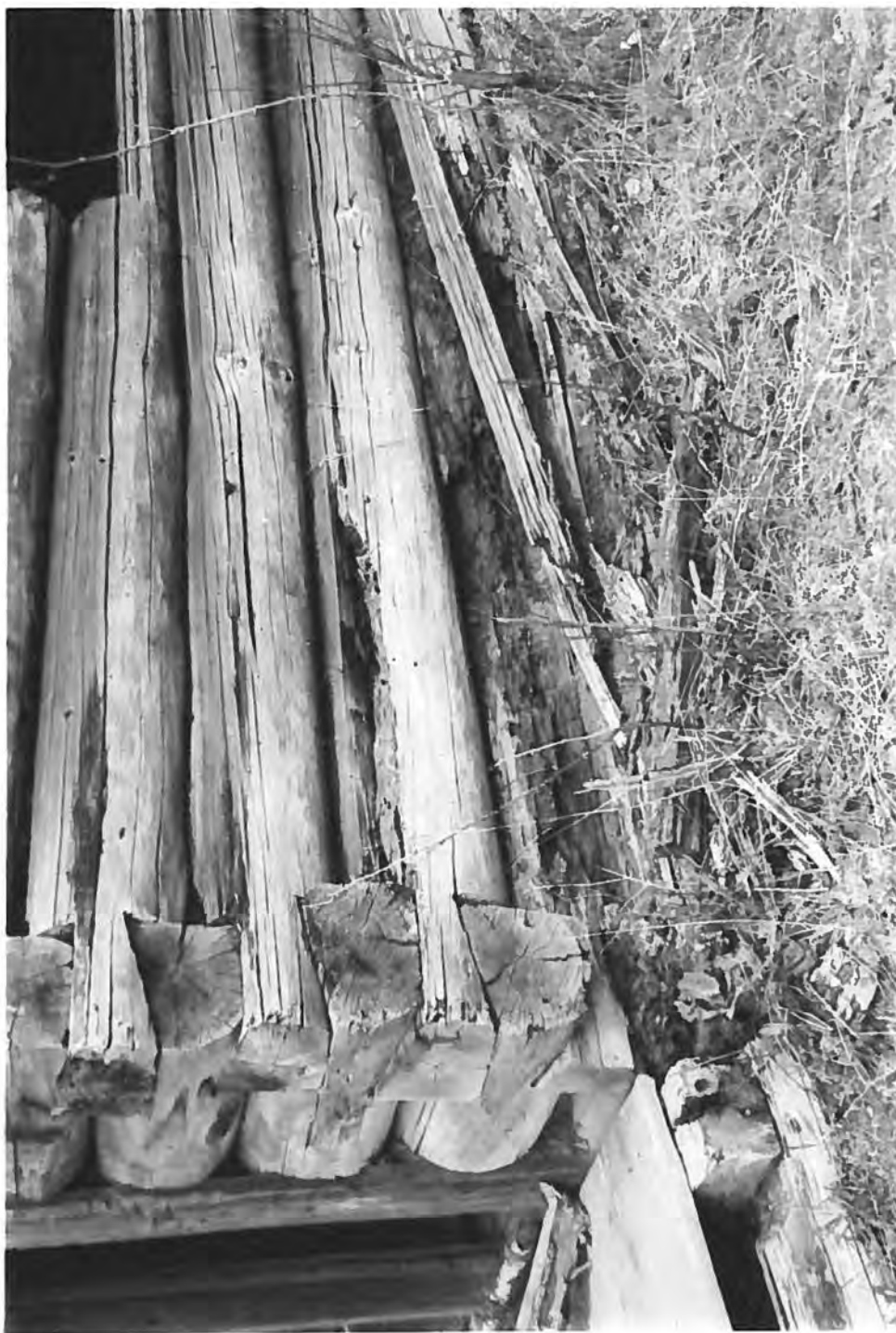
Illustration No. 10: Condition of logs - westerly side at entrance.
