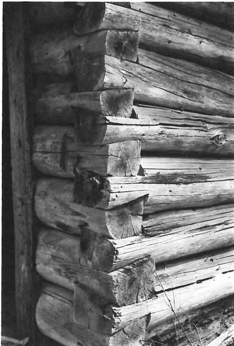
Illustration No. 11: Detail, corner joints of logs.
