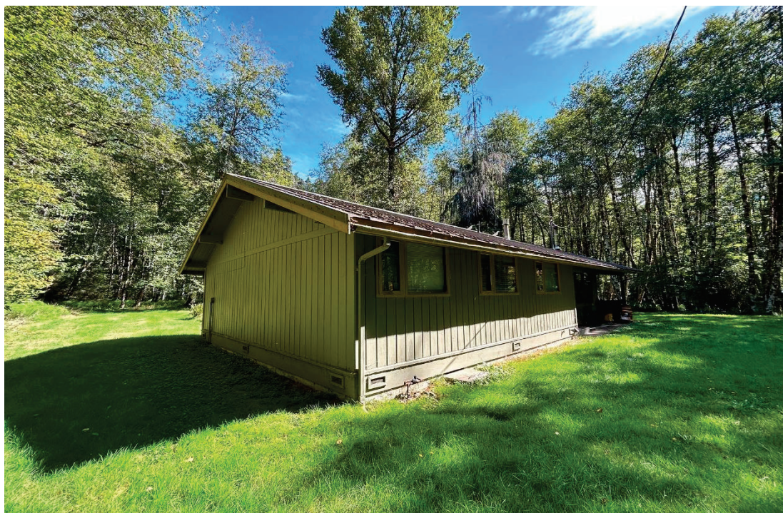
Photo 14. Building 1155 (Oly House). View to southeast.
