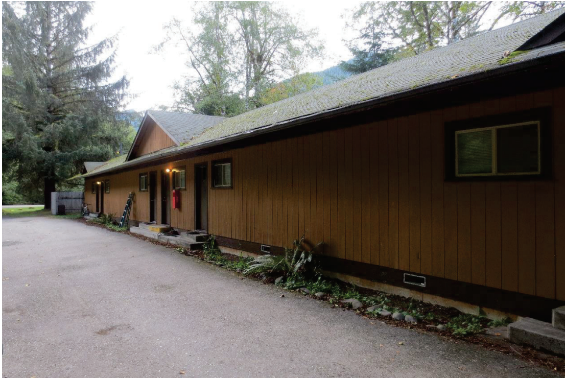
Photo 15. Building 1156, which in 2025 is used as concession housing. View to south.
