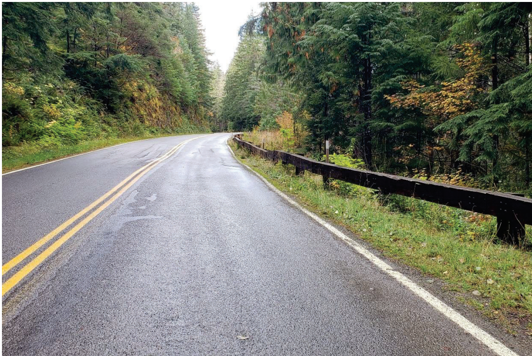
Photo 4. Wood guardrails line the road along steep slopes (here, at 1.7 miles). View to southwest.
