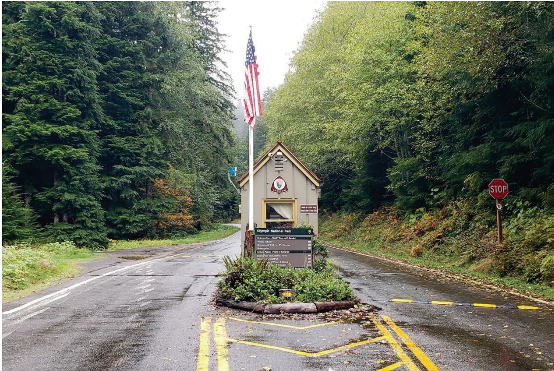
Photo 3. Fee station at 0.3 miles. View to southwest.
