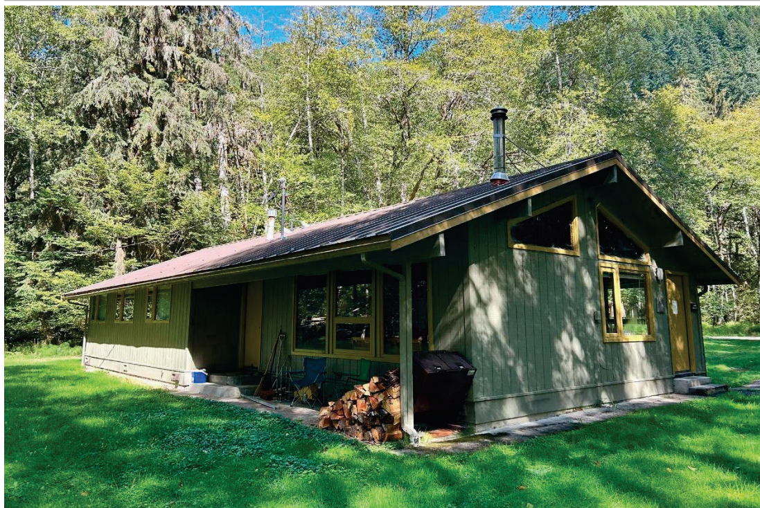
Photo 13. Building 1155 (Oly House). View to north-northeast.
