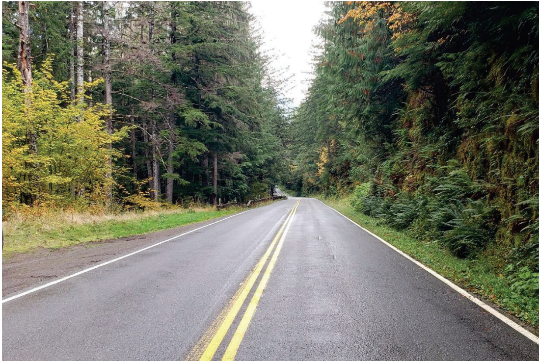
Photo 5. A typical section of Sol Duc Road, at 2.4 miles. View to northeast.
