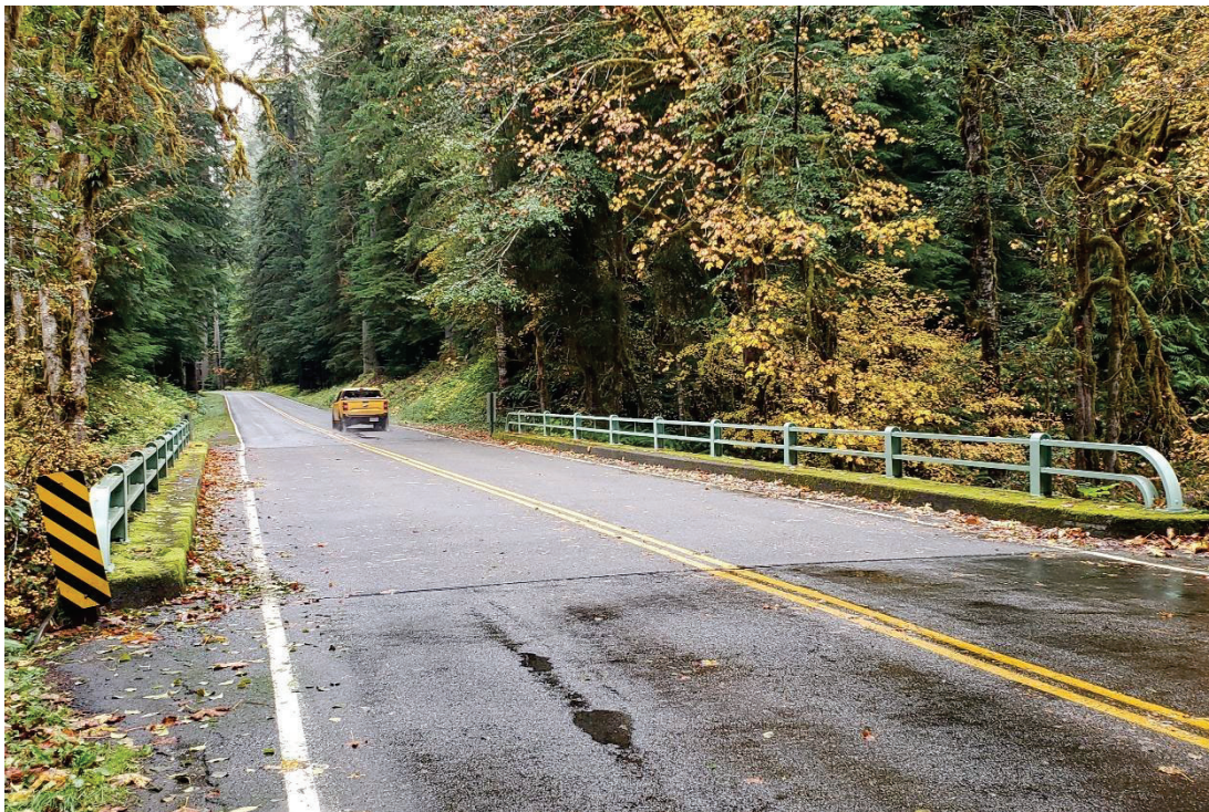
Photo 6. North Fork Sol Duc River Bridge, at 5.2 miles. View to northwest.
