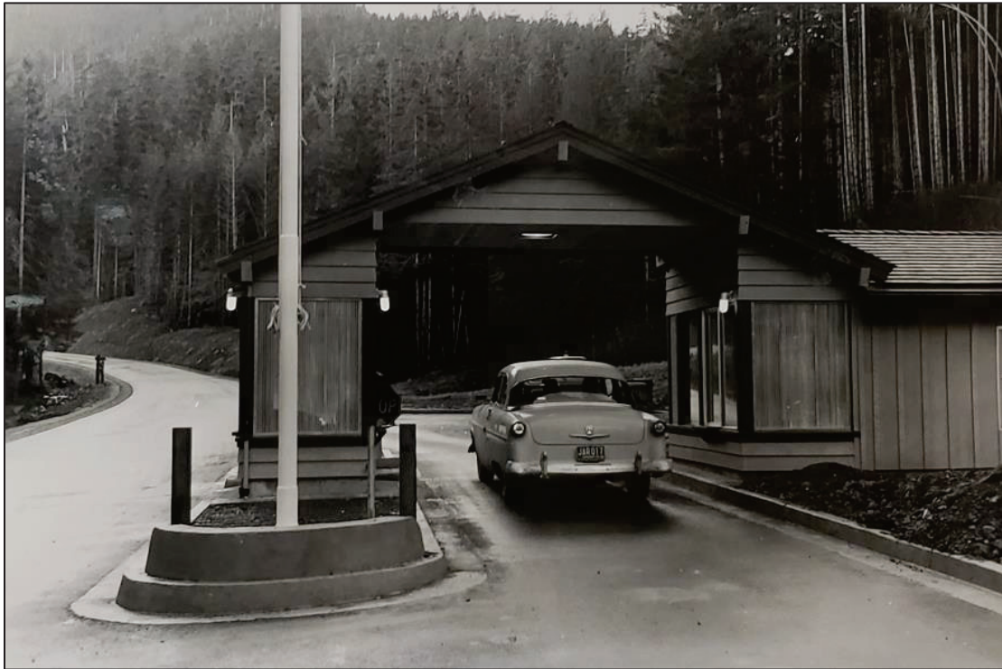
Figure 10. Heart o' The Hills entrance station. The fee booth was on the left, while staff offices were on the right. National Park Service photo.
