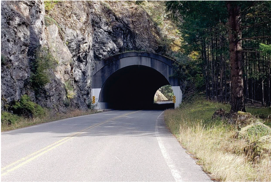
Photo 9. The southwest (uphill) side of Tunnel #2. View to northeast.
