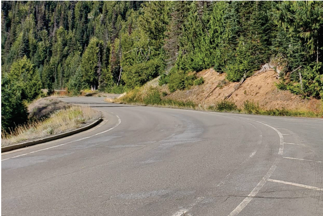
Photo 13. A section of road just west of the Switchback Trailhead. View to west.
