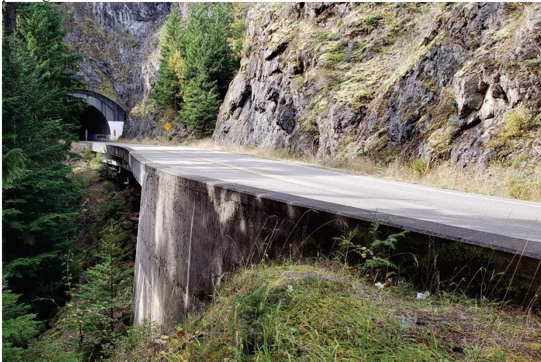
Photo 8. The North Viaduct and Tunnel #1 are located just south of the Morse Creek Overlook. View to west-southwest.
