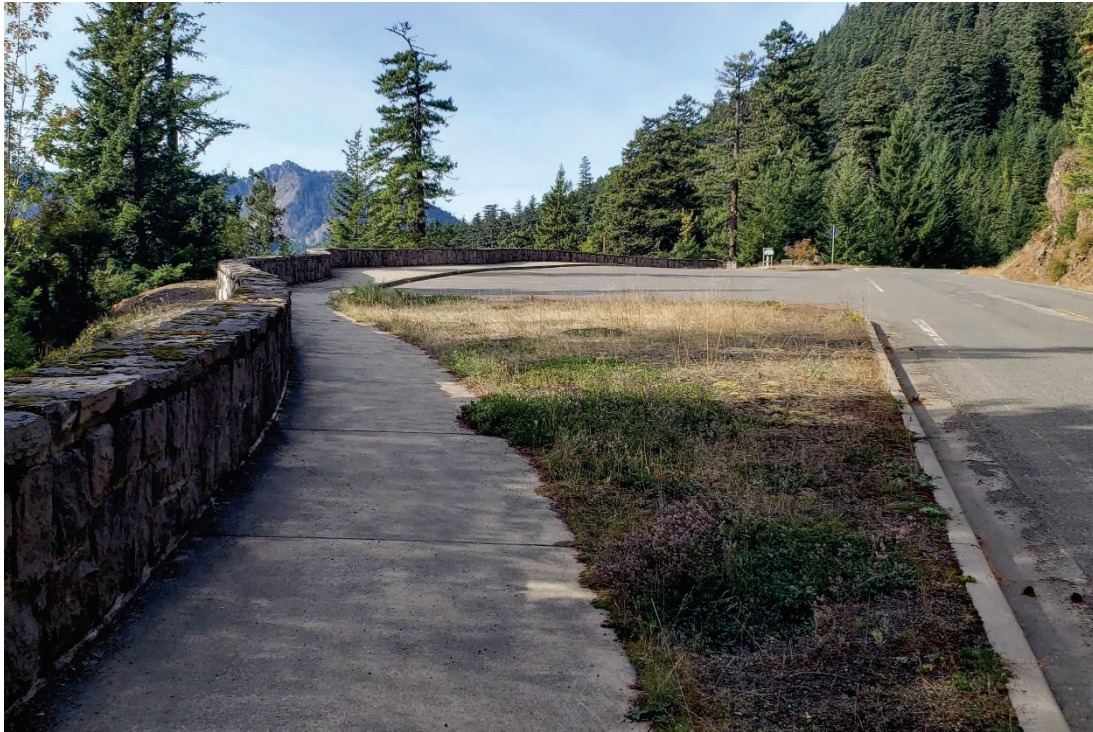
Photo 11. Double Overlook at mile 11.6 includes two parking areas that are connected by a walkway (added in 2008) and bordered by a rock-faced wall (erected in 2008). View to southwest.
