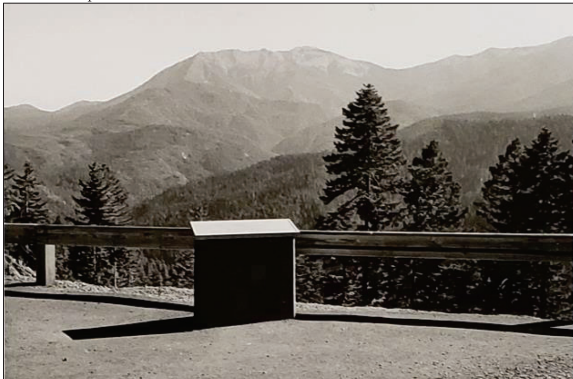
Figure 7. "Station 330," now part of Double Overlook, in 1957. The concrete and aluminum interpretive stands have been replaced with fiberglass stands, and the guardrail has been replaced by a stone-faced concrete wall. National Park Service photo.
