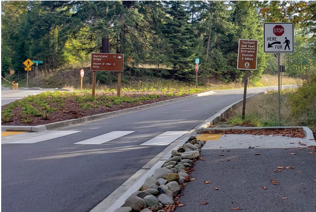
Photo 1. Hurricane Ridge Road begins at the intersection with Mt. Angeles Road in Port Angeles. View to south.
