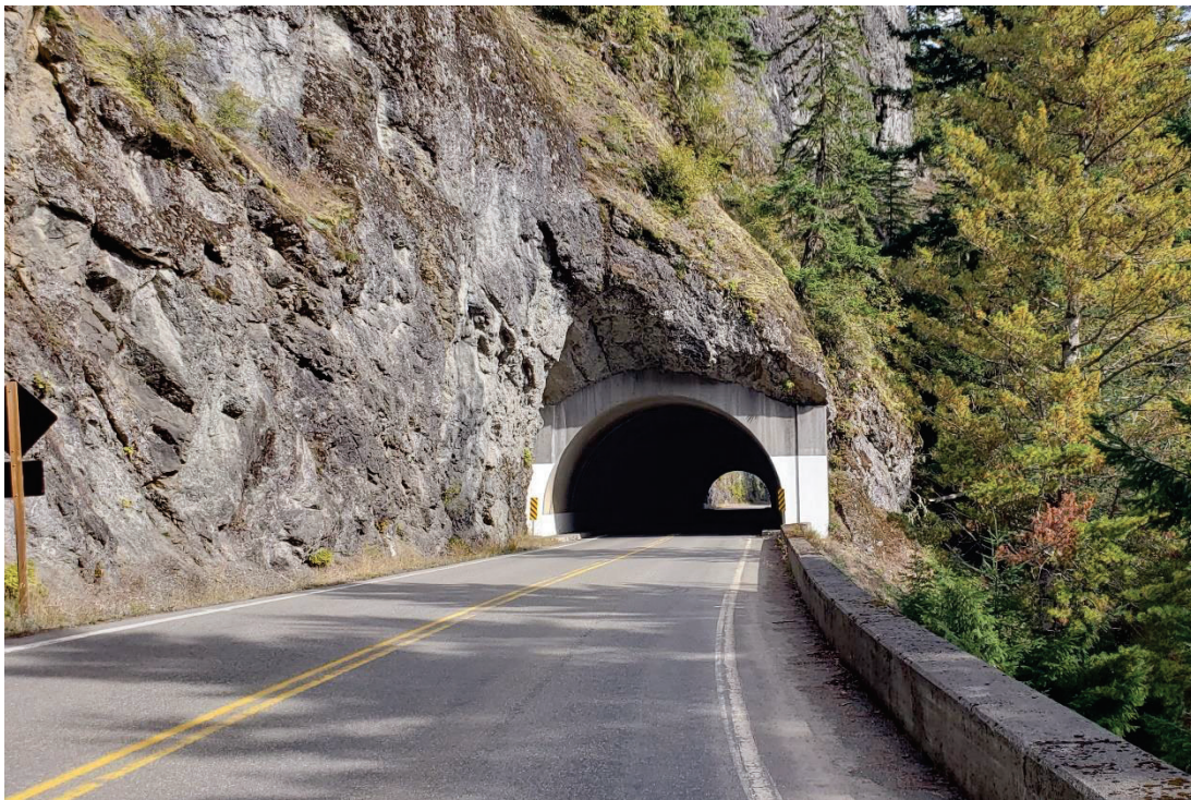
Photo 10. The southwest (uphill) side of Tunnel #3. The road in this section is supported by the South Viaduct. View to northeast.
