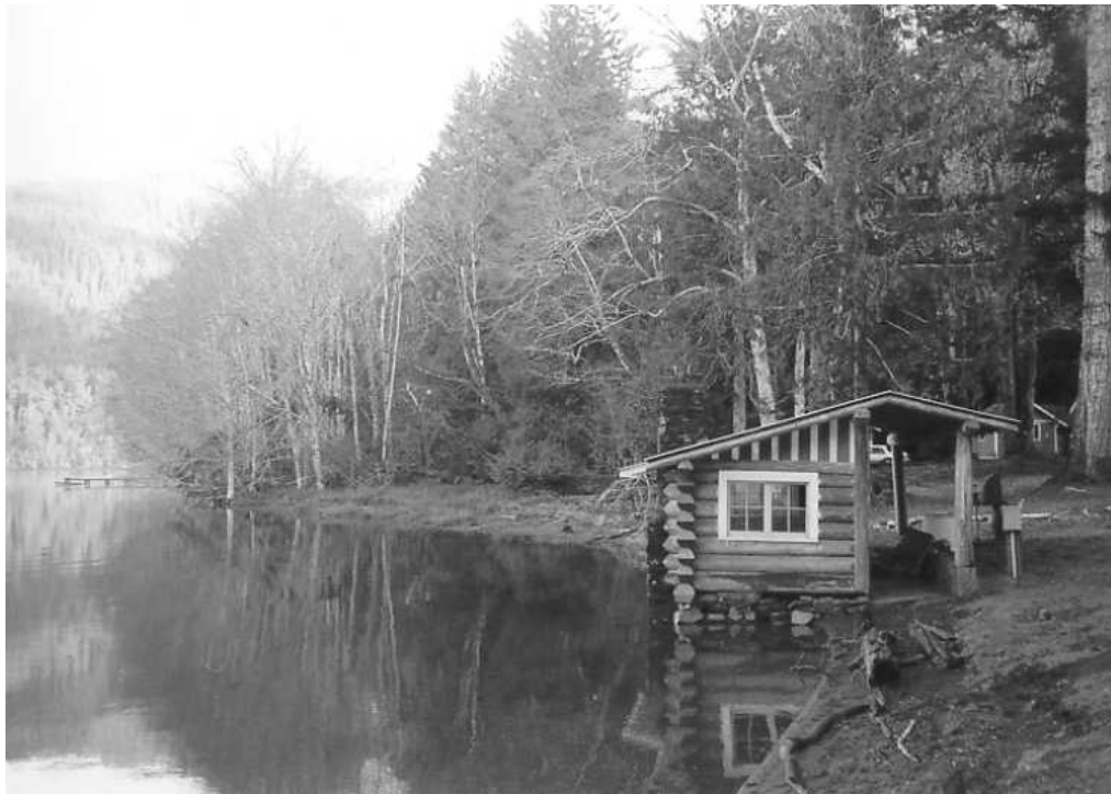
Contemporary photograph of Inglenook, the Fireplace Shelter at Rosemary Inn, built in 1933. Note the inundation of the foundation, due to the erosion of the lake shore. (CCSO, 1999.)
