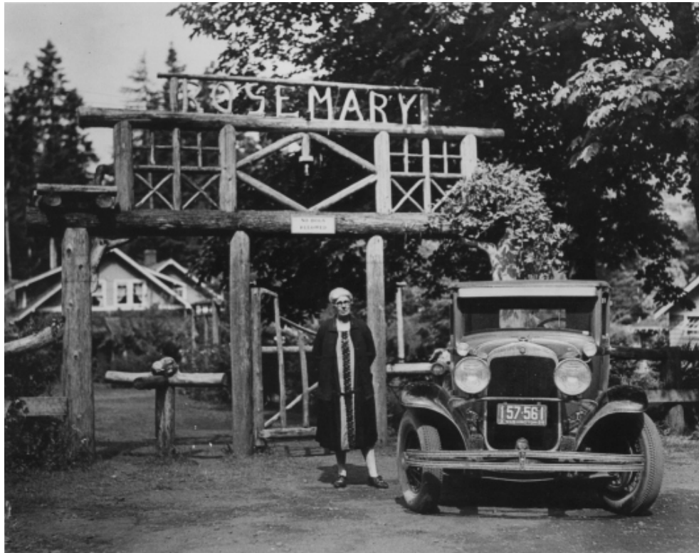
Historic photograph of the second Rosemary gate, built in response to the opening of the Olympic Highway in 1922. Rose Littleton appears in the photograph, along with rustic log fences and turnstyles, c. 1937. (OLYM 220/2397, n.d.)
