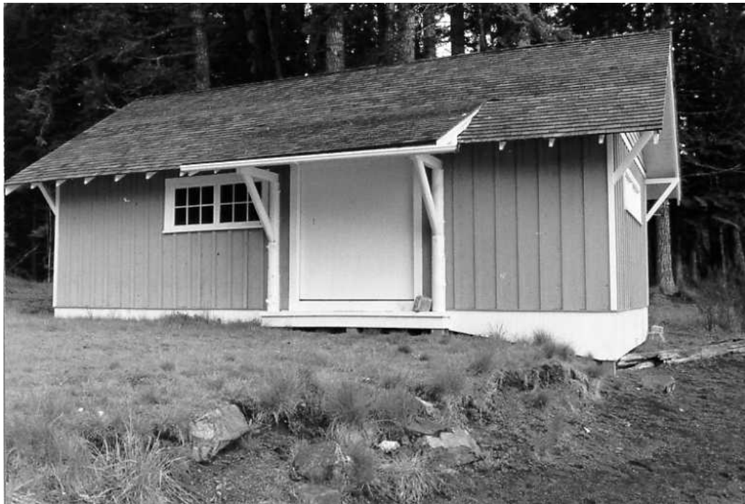
Contemporary photograph of the Boathouse at Rosemary Inn, built in 1936. (CCSO, 1999.)
