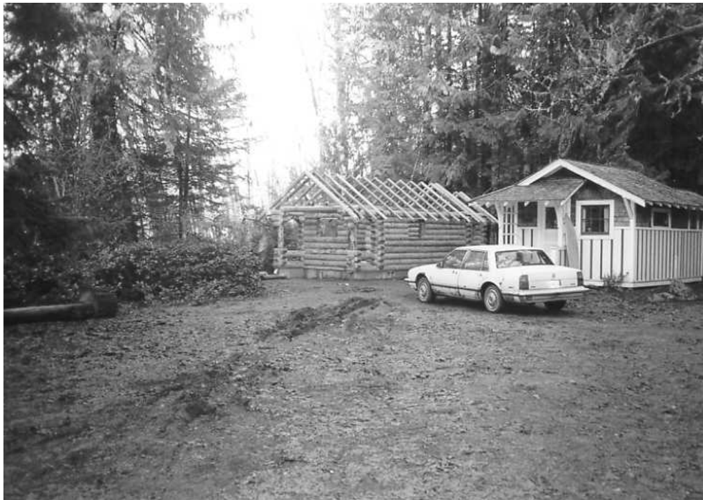
Contemporary photograph of Dixie (center), one of the guest cabins at Rosemary Inn, built before 1926. Dixie was being reconstructed at the time of the photograph. (CCSO, 1999.)
