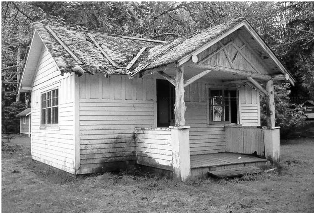
Contemporary photograph of Summerie, a guest cabin at Rosemary Inn, built before 1926. Summerie had not been reconstructed at the time of the photograph and was in poor condition. (CCSO, 1999.)
