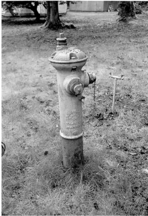
LCS photograph of a small scale feature at Rosemary Inn: a fire hydrant. The fire hydrant is inscribed with "Rensselaer Valve Co, Troy NY, Makers" and "The Corey" and dates from the historic period. (CCSO, 1990.)
