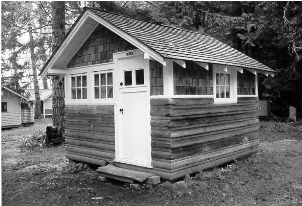
Contemporary photograph of Wren, one of the guest cabins at Rosemary Inn, built before 1926 and reconstructed in the 1990s. (CCSO, 1999.)
