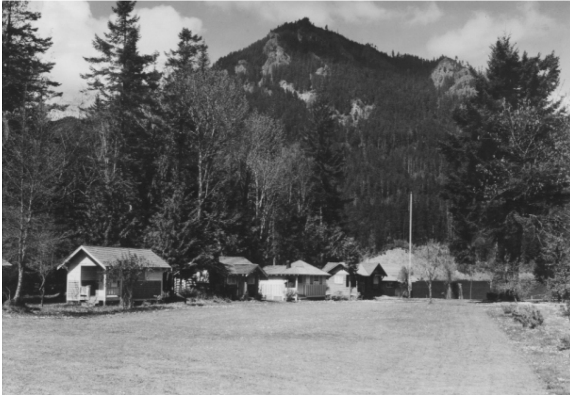
Historic photograph of the unique guest cabins that replaced the tent cabins at Rosemary Inn. Note the flagpole in the distance which was added in the 1930s, and the plantings around the cabins. (OLYM 220/2434C, n.d.)
