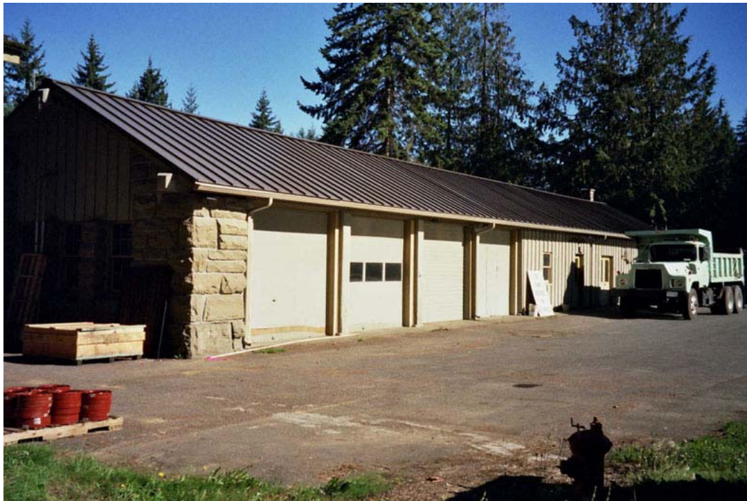
Contemporary photograph of the historic Roads & Trails Shop completed in 1941, looking northeast. (CCSO, 2002)
