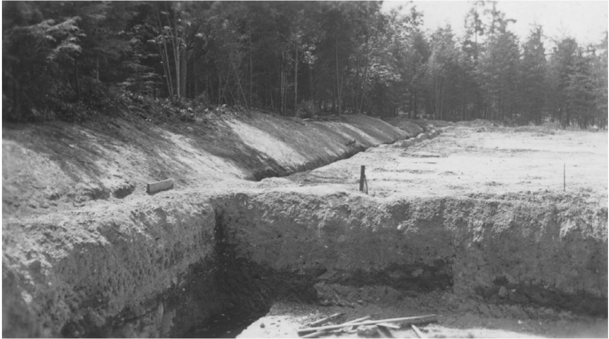
Historic photograph showing the beginning stages of construction in 1940 of the Equipment Shed/Carpenter Shop that was not completed until 1944. (Monthly Report 6/24/40, OLYM archives)
