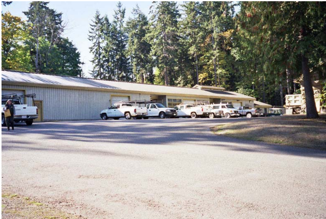
Contemporary photograph showing a historic portion of the maintenance area circulation system in front of the Maintenance/Procurement building. (CCSO, 2002)
