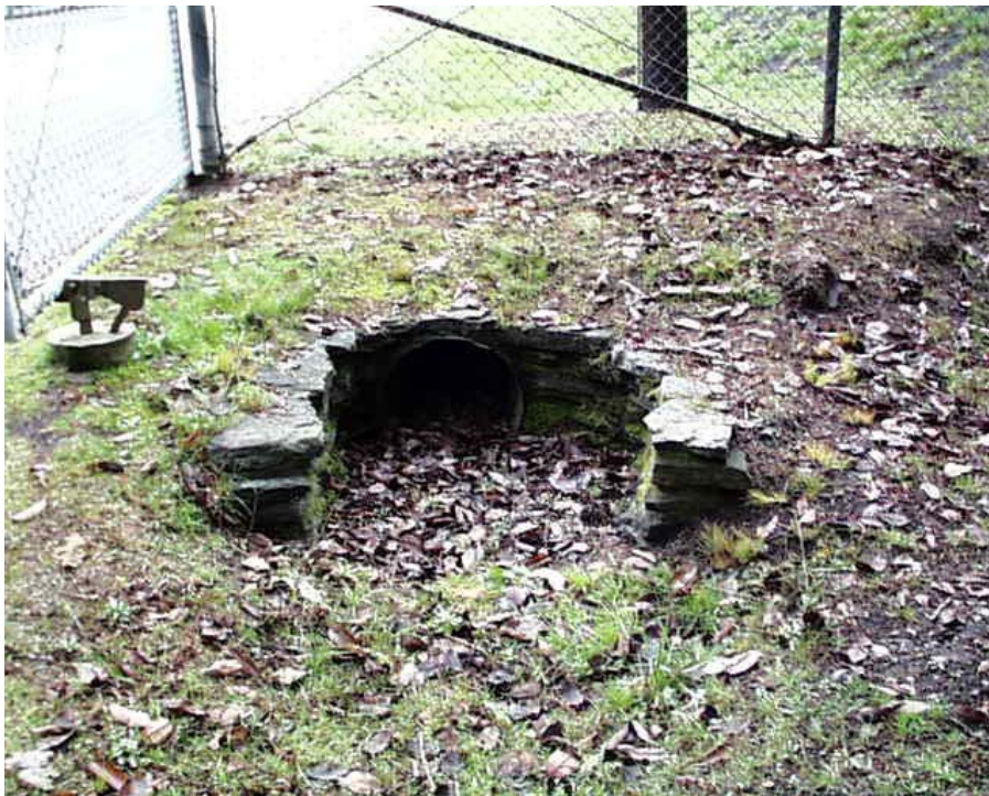
Contemporary photograph showing the non-historic culvert installed in conjunction with the chain-link fence. (CCSO, 2002)
