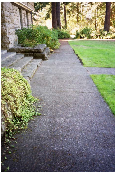
Contemporary photograph showing the non-historic concrete walkways that replaced the original flagstone walkways in front of the Administration building in the late 1950s. (CCSO, 2002)
