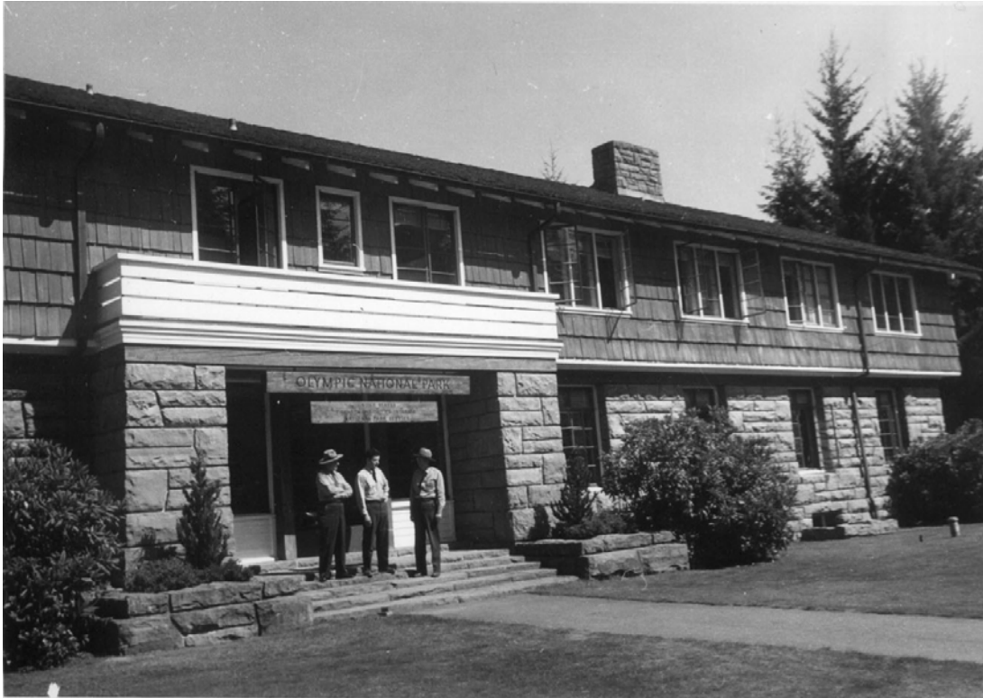
1950s photograph showing the concrete walk that replaced the flagstone walk at the back entrance to the Administration building. Note that no other connecting walkways exist at this time. (OLYM 2548A, OLYM archives)
