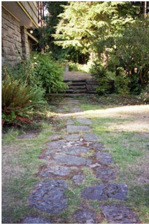
Contemporary photograph showing a historic flagstone path and terrace at the Superintendent's residence. (CCSO, 2002)
