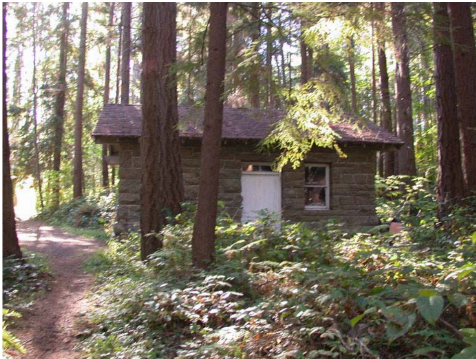
Contemporary photograph of the historic Transformer/Pump house completed in 1941, looking south. (CCSO, 2002)
