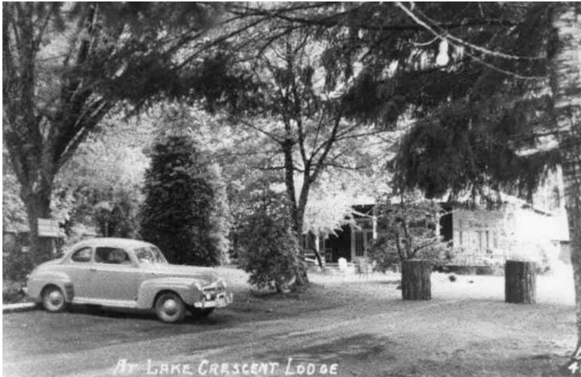
Historic photograph from the late 1940s showing the parking area developed near the lodge for guests' vehicles. (OLYM / At Lake Crescent Lodge, ca. 1948.)
