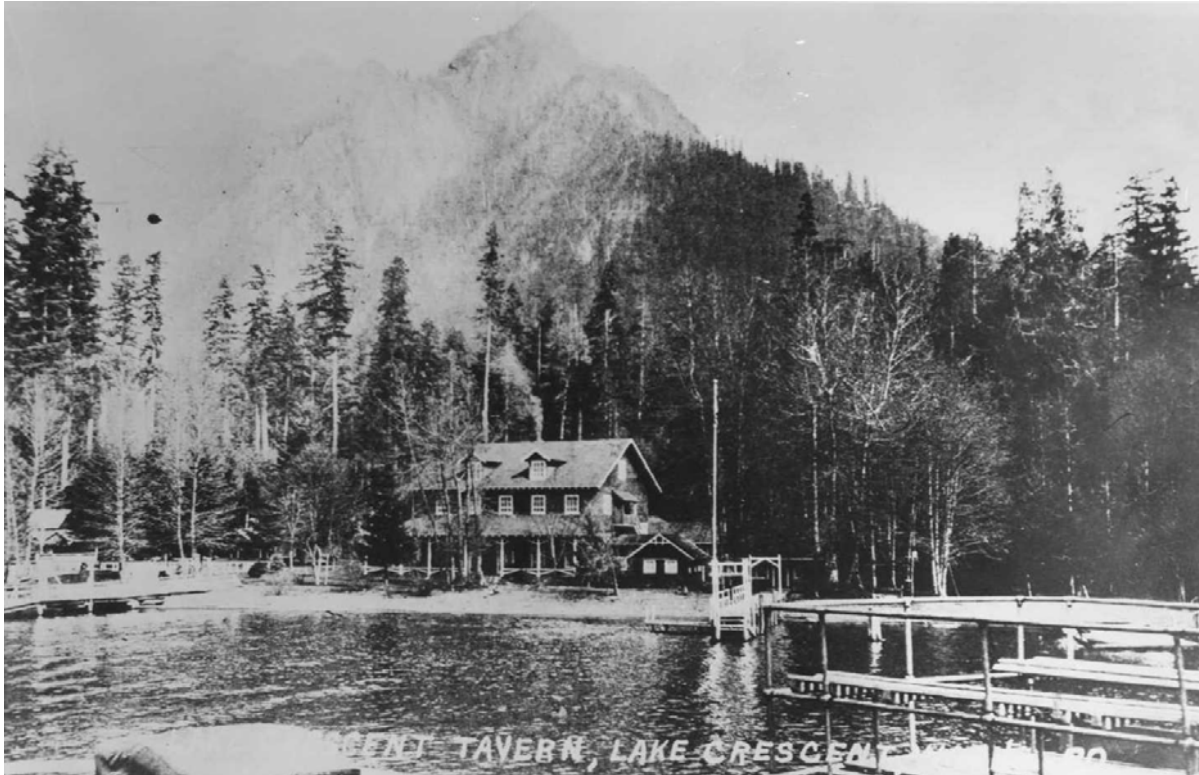
Historic photograph of the lodge from the ferry boat in Lake Crescent. Note the large ferry dock and the small craft dock, and the mature trees along the beach. (OLYM / P.A.West/217, Bert Kellogg Collection, Clallam County Historical Society, n.d.)
