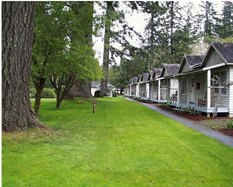
Contemporary photograph showing the row of reconstructed cabins that provide a major edge to the central courtyard space. Note the two mature Hawthorn trees and the water hydrant. (CCSO, 2000.)
