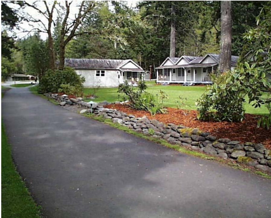
Contemporary photograph of the rubblestone wall. Rebuilt in the 1980s, this wall originally bordered the horseshoe pit. The wall currently retains planting beds. (CCSO, 2000.)
