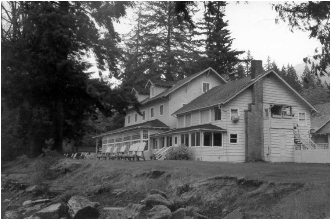
Contemporary photograph of lodge from the lakeshore. (CCSO, 2000.)
