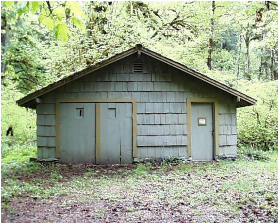
Contemporary photograph of the garage/wood shed located in the Graves Creek Ranger Station Historic District. (CCSO, 2000.)
