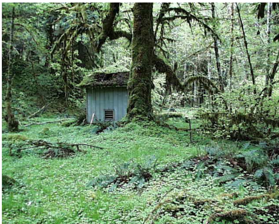
Contemporary photograph showing the vegetative path that leads from the rear of the ranger station to the generator house. (CCSO, 2000.)
