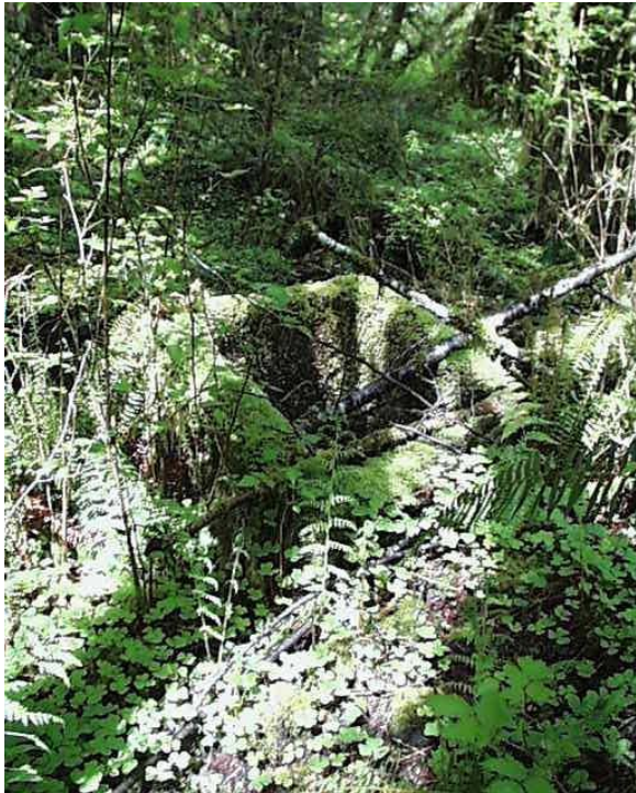
Contemporary photograph of the second concrete basin that was part of the water intake system. (CCSO, 2000.)
