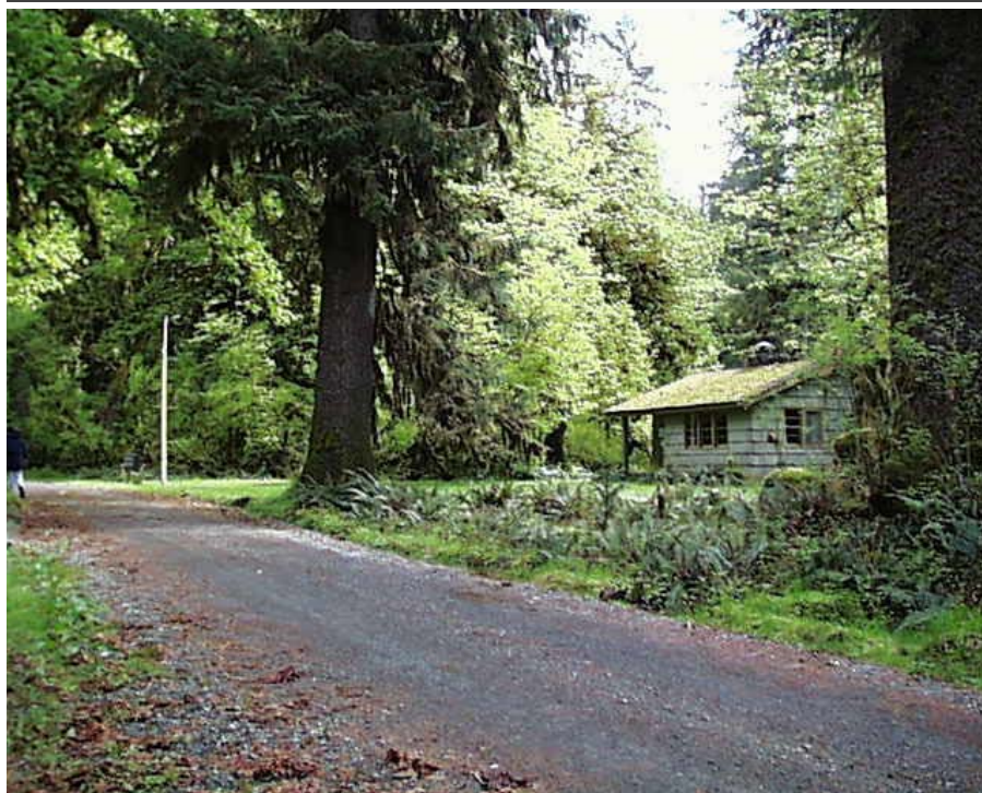
Contemporary photograph showing the view of the ranger station from the road. (CCSO, 2000.)
