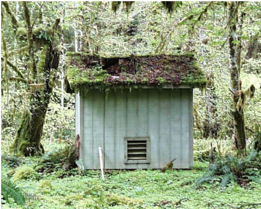
Contemporary photograph of the generator house located in the Graves Creek Ranger Station Historic District. (CCSO, 2000.)
