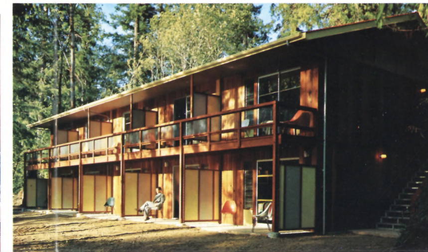
STORM KING MOTOR LODGE
