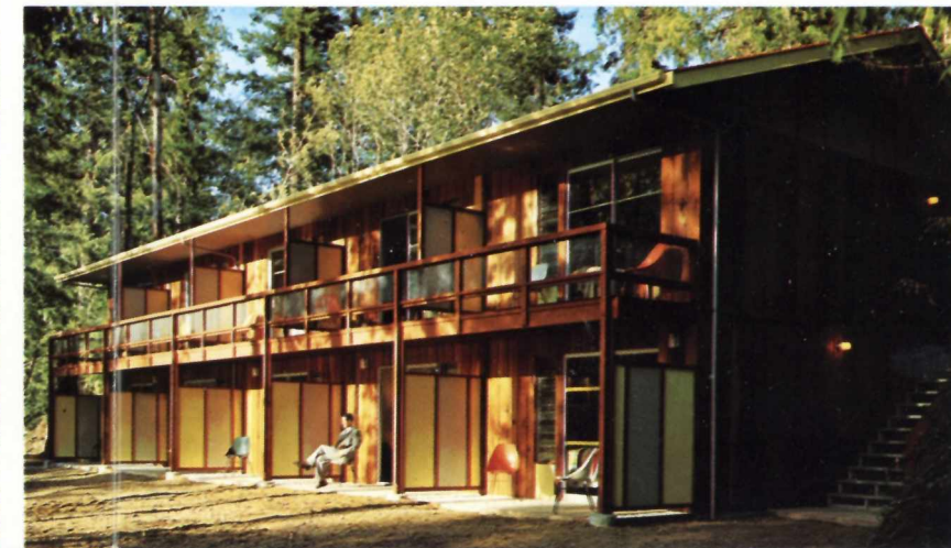
STORM KING MOTOR LODGE
