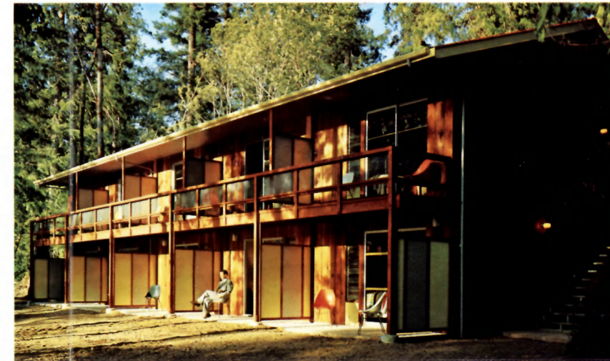
STORM KING MOTOR LODGE
