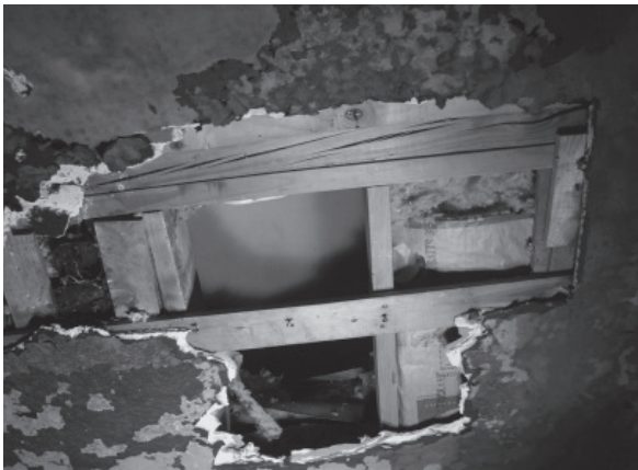
Figure 7. View of framing for ceiling in Room 108 that was added in 1952-1953, left, and a view of typical roof framing in the attic, right.
