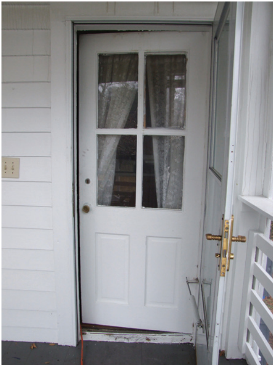
Figure 13. View of kitchen back door, installed in 1952.
