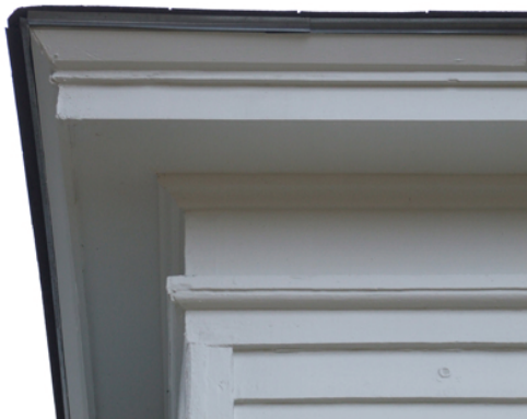
Figure 14. View of typical original exterior woodwork.
