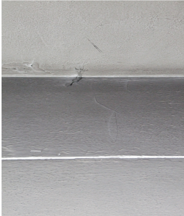
Figure 18. View of juncture of living room wall with ceiling, showing the slightly thicker plaster evident in the frieze.
