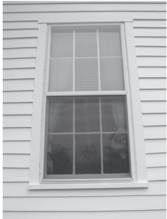
Figure 9. View of typical 1856 window opening.
