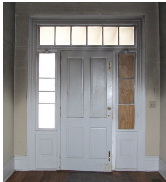
Figure 12. View of front door, transom, and side-lights.
