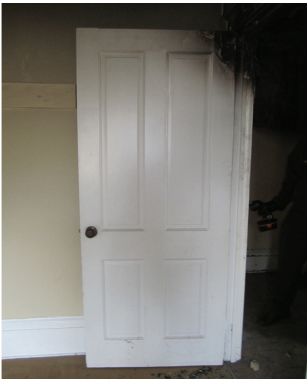
Figure 24. View of typical four-panel door.
