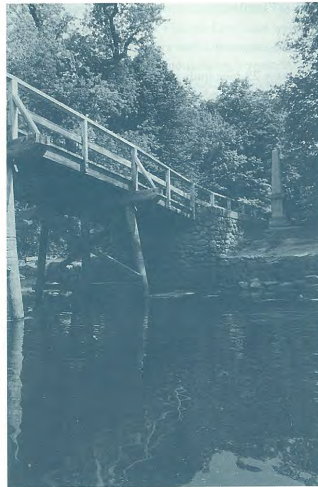
North Bridge, Concord.
